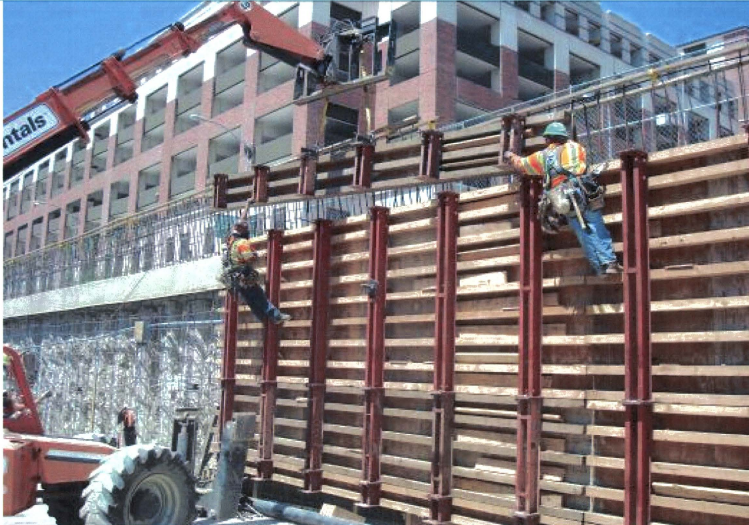
Placement of U-Section Wall Form at Grade Separation Trench Structure
