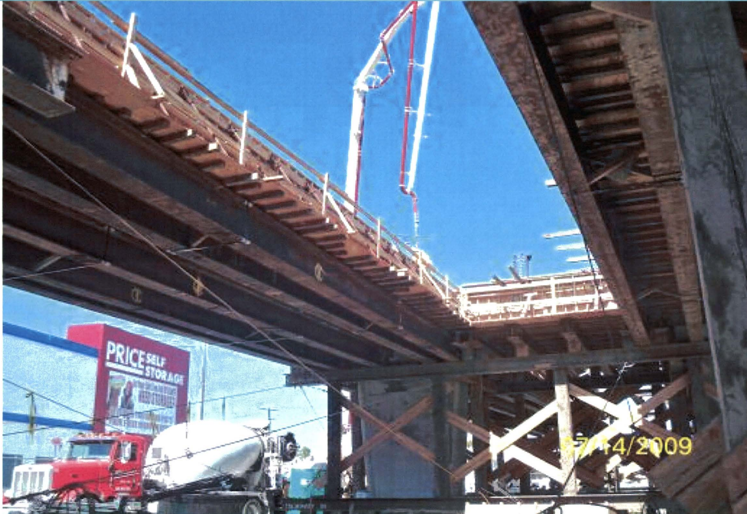
Concrete Placement for Soffit and Stem Wall at La Brea Overcrossing Structure
