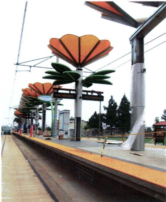
East Los Angeles Civic Center Station
