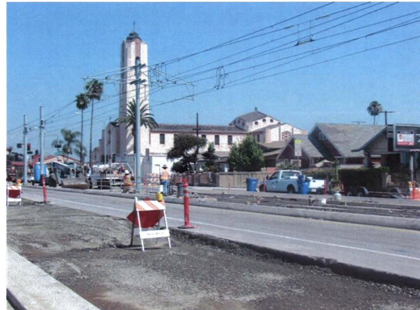
Demolition and removal of colored concrete topping slab near 3 rd /Ditman.
