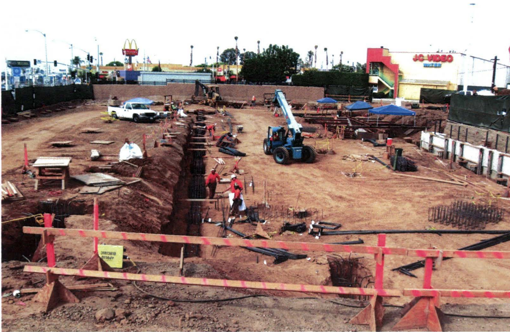
View of the construction site looking south
