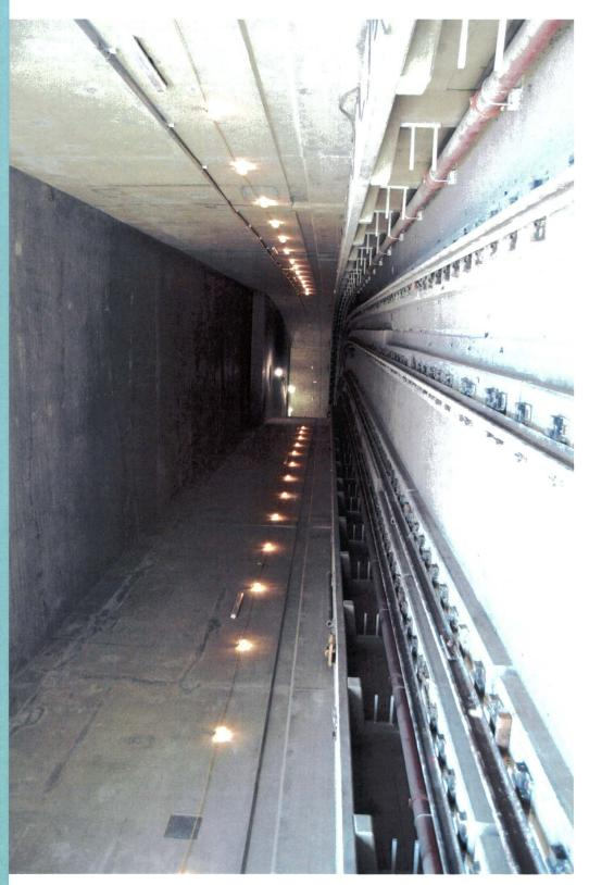
**Direct Fixation Trackwork in Trench Structure**
