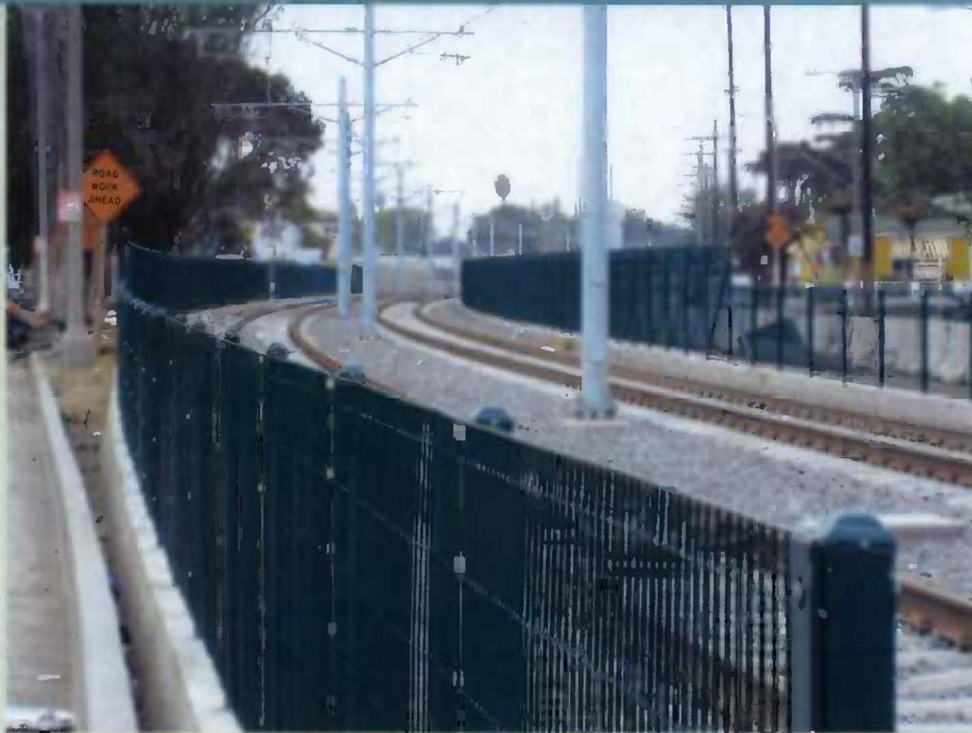
Installed Right-of-Way Fencing near Arlington Avenue
