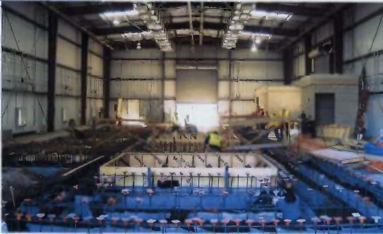
Concrete formwork for the under-floor duct system and vehicle hoists pits.
