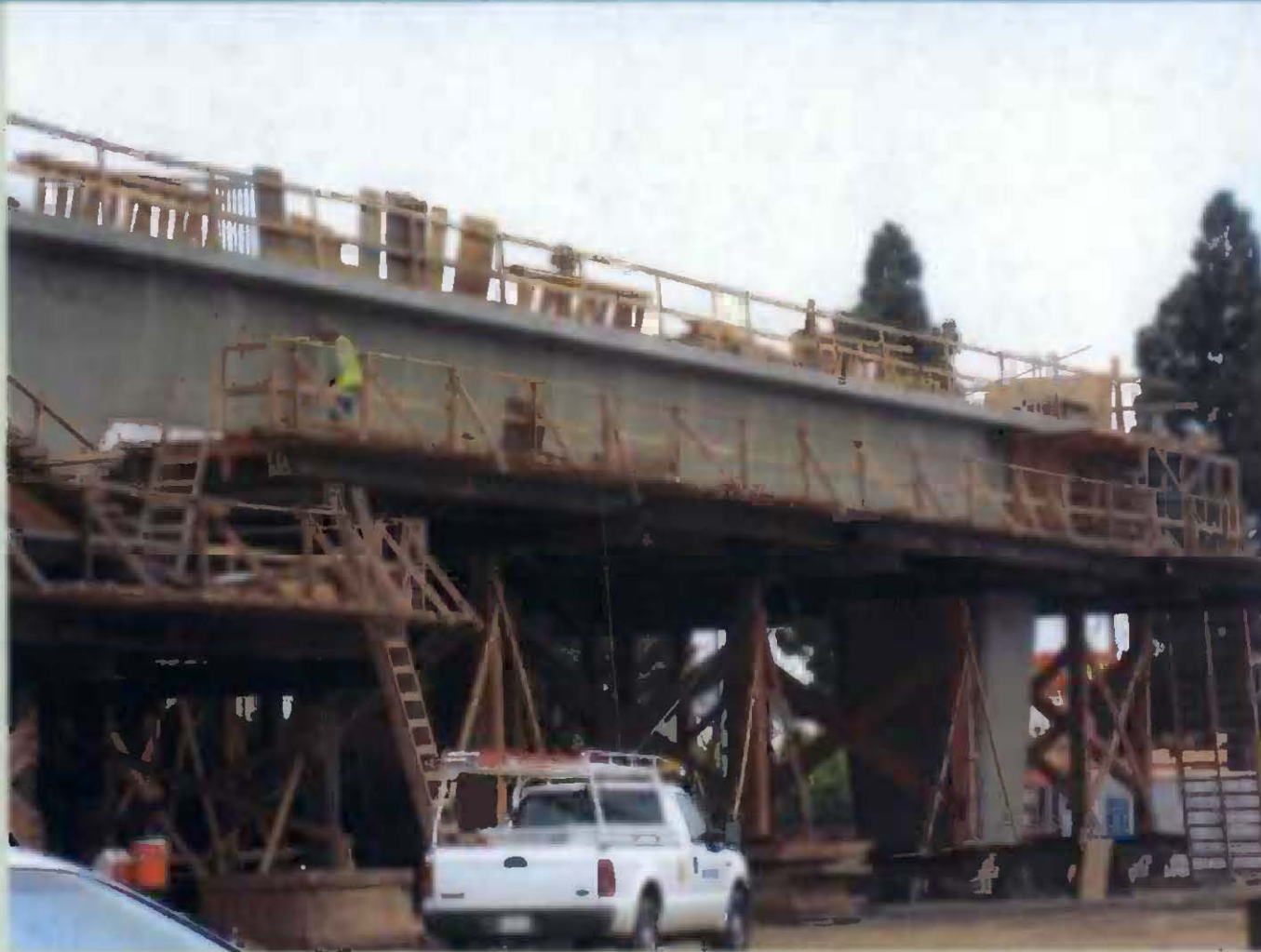
Progress on the Venice/Robertson Aerial Structure
