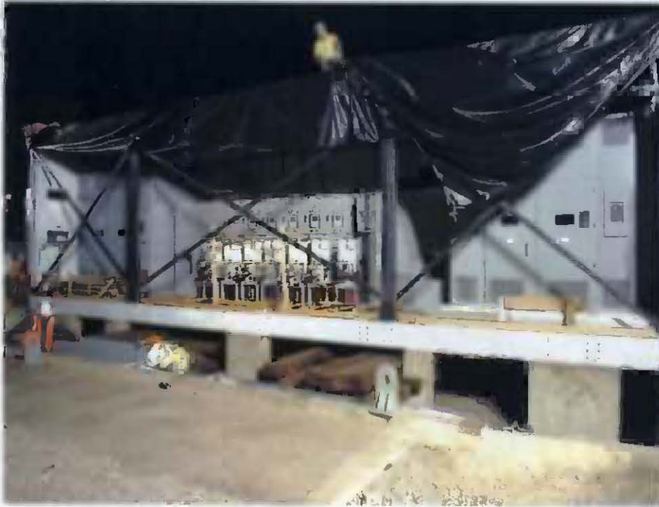
Installation of 1 st Substation on July 10, 2010
