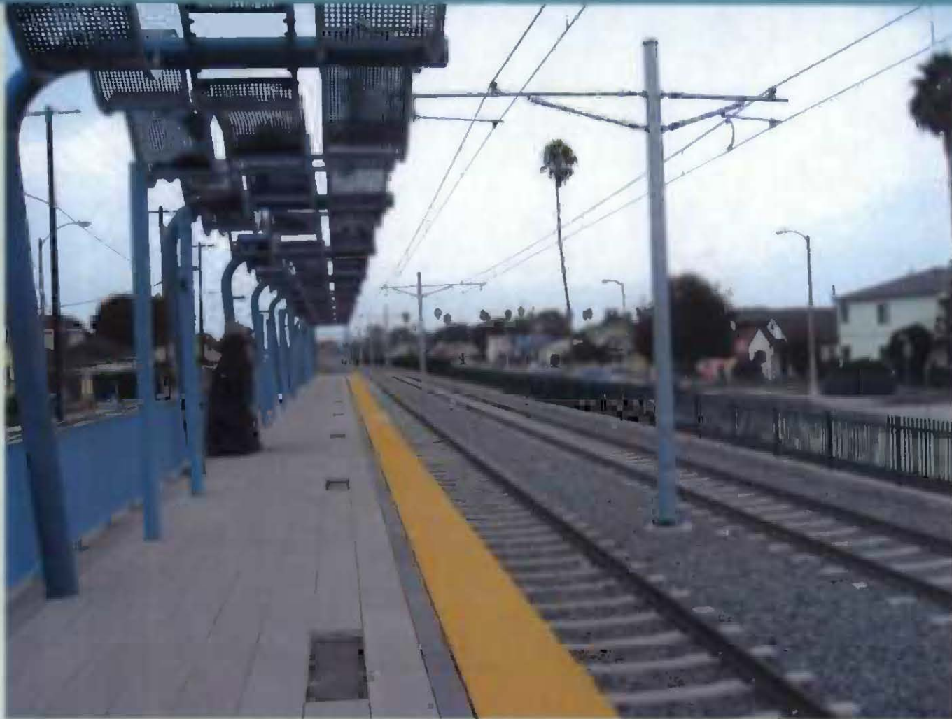
Crenshaw Station Eastbound Platform
