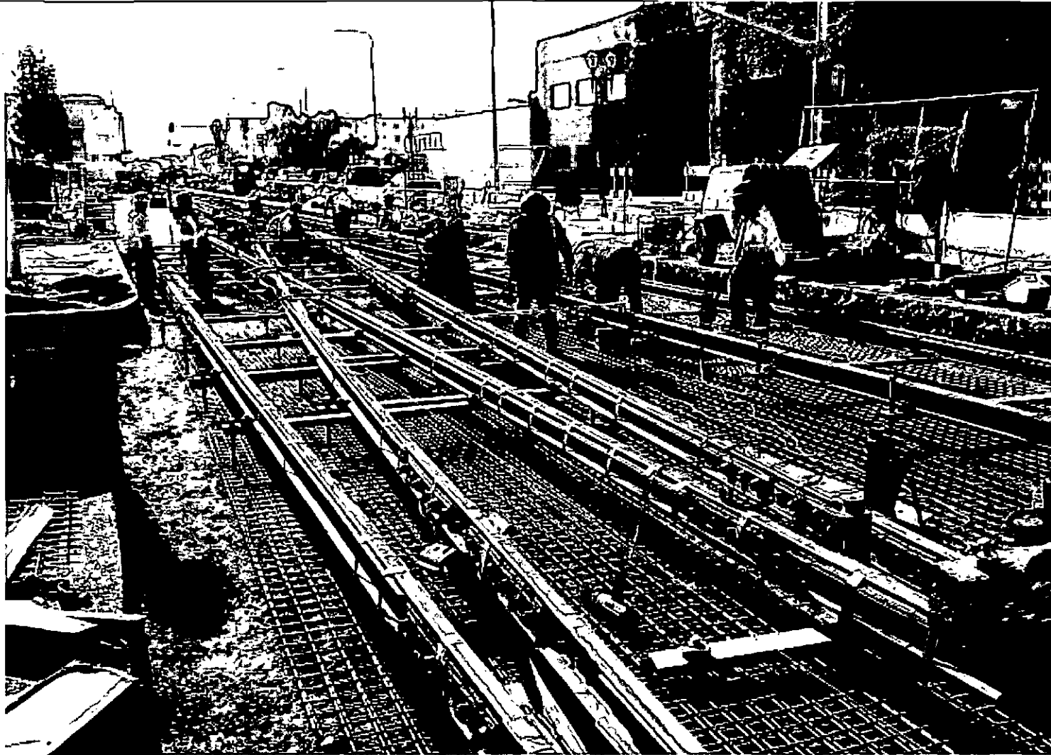
Installation of Embedded Crossover at 23rd Street and Flower Street
