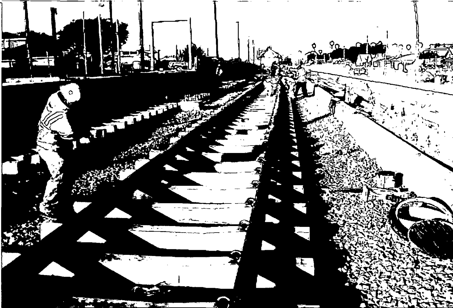
Installation of Tracks at Crenshaw Station
