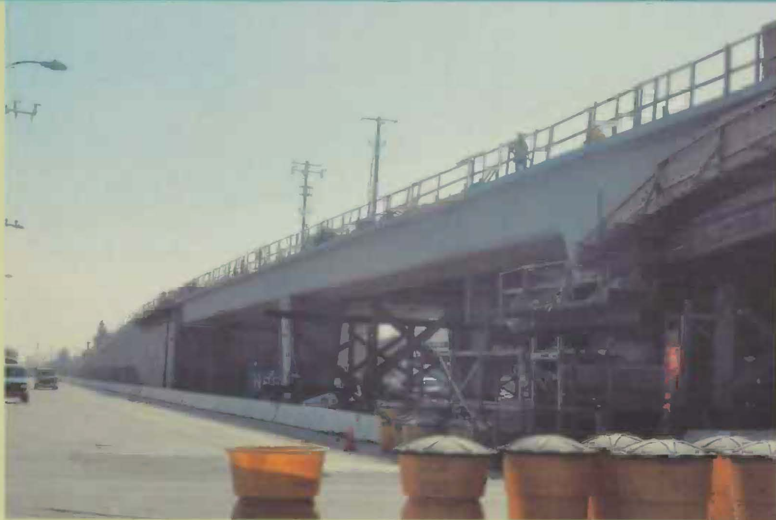
Falsework Removal at La Brea Aerial Structure
