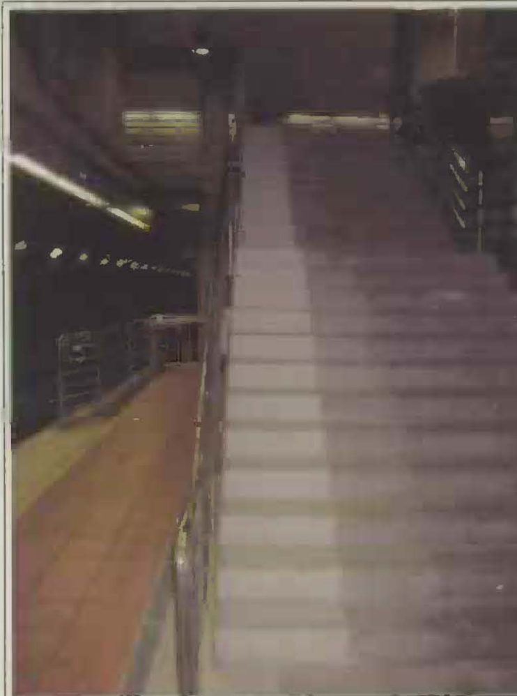
Station Emergency Egress – widening of stairs
