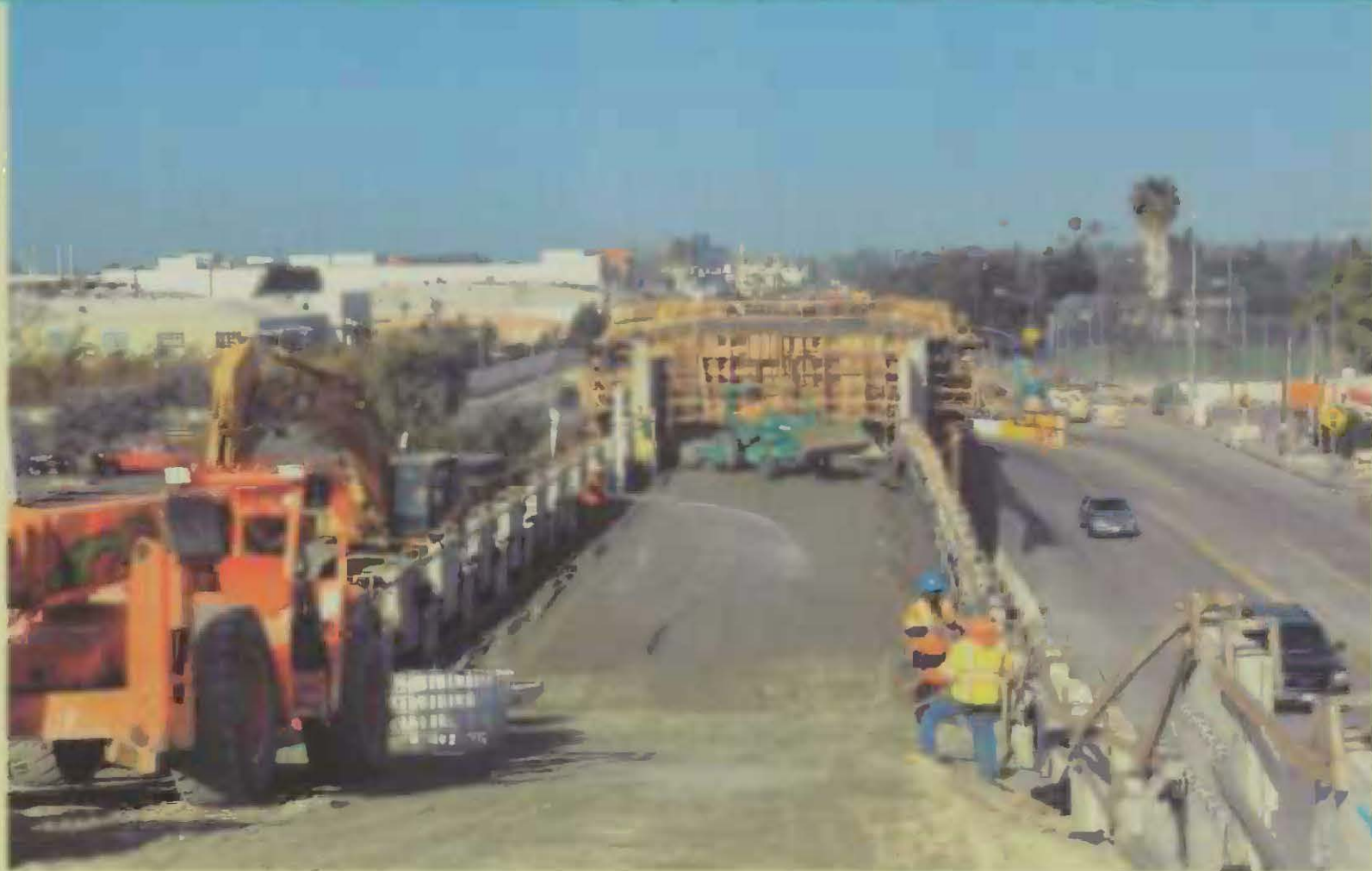
MSE Walls From La Cienega Aerial Structure to Ballona Creek Aerial Structure
