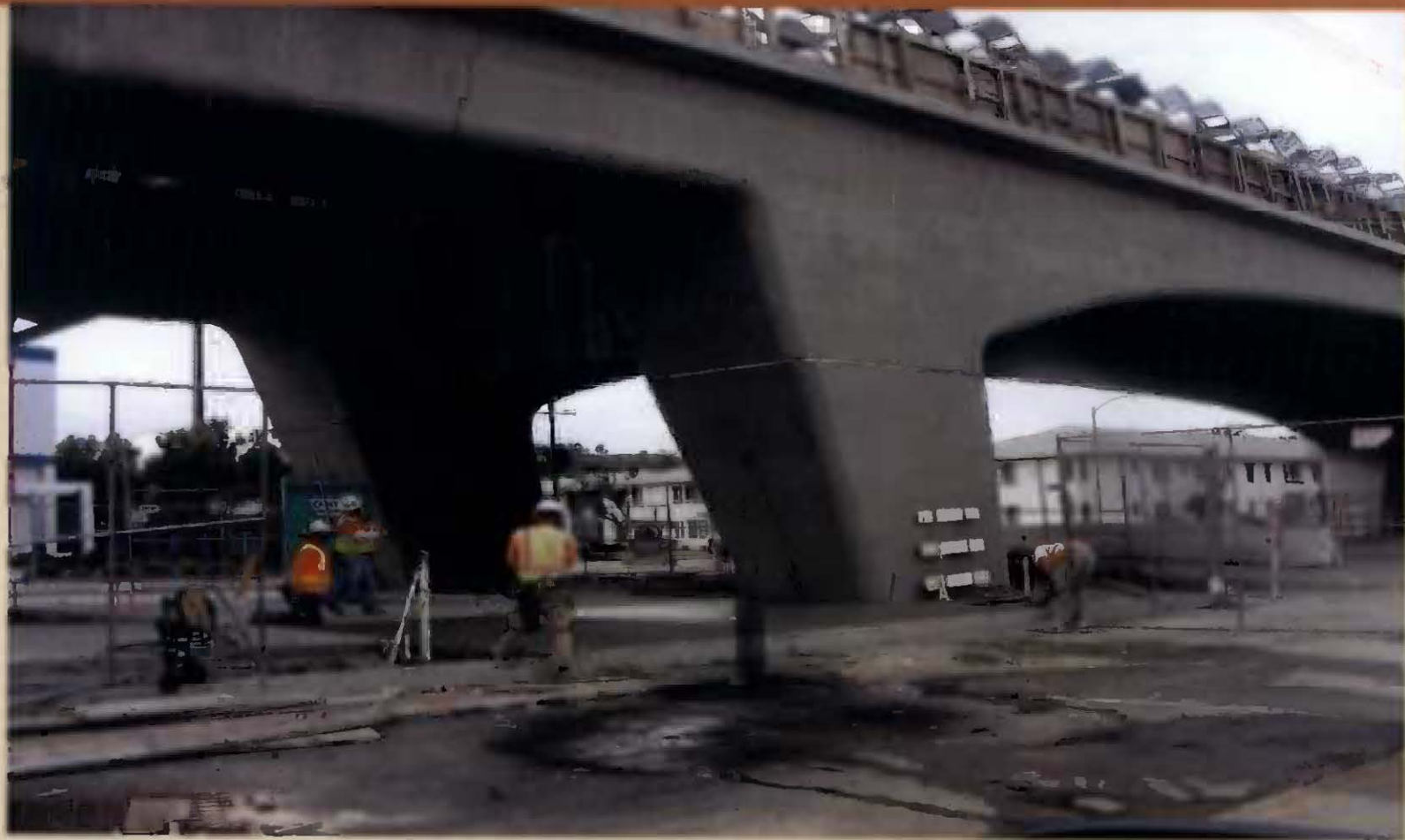
Slab-On-Grade Concrete Placement at La Brea Aerial Station East Plaza
