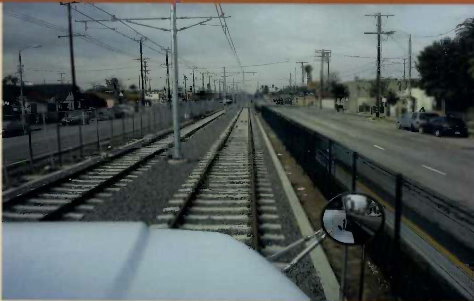
Looking West from Inside Cab of Track Geometry Testing Vehicle
