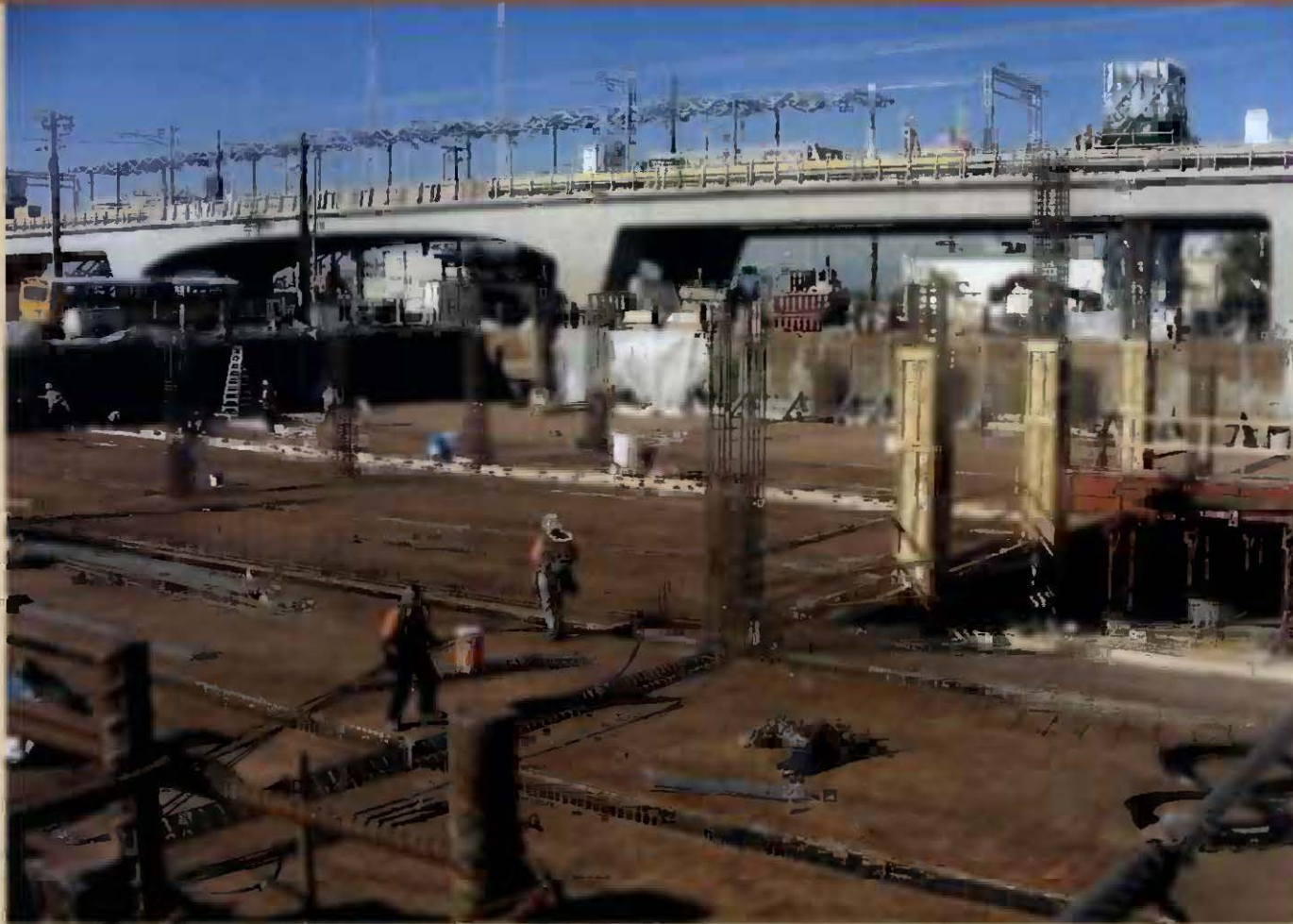
Rebar Installation for Parking Level 1 at La Cienega Parking Structure
