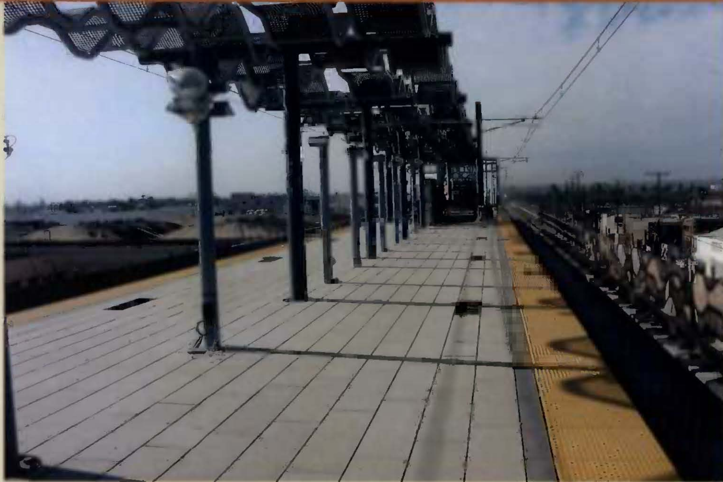
La Cienega Aerial Station Platform – Looking West
