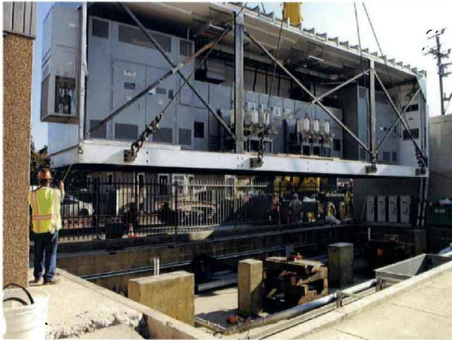
Installation of San Pedro Substation on November 16, 2010
