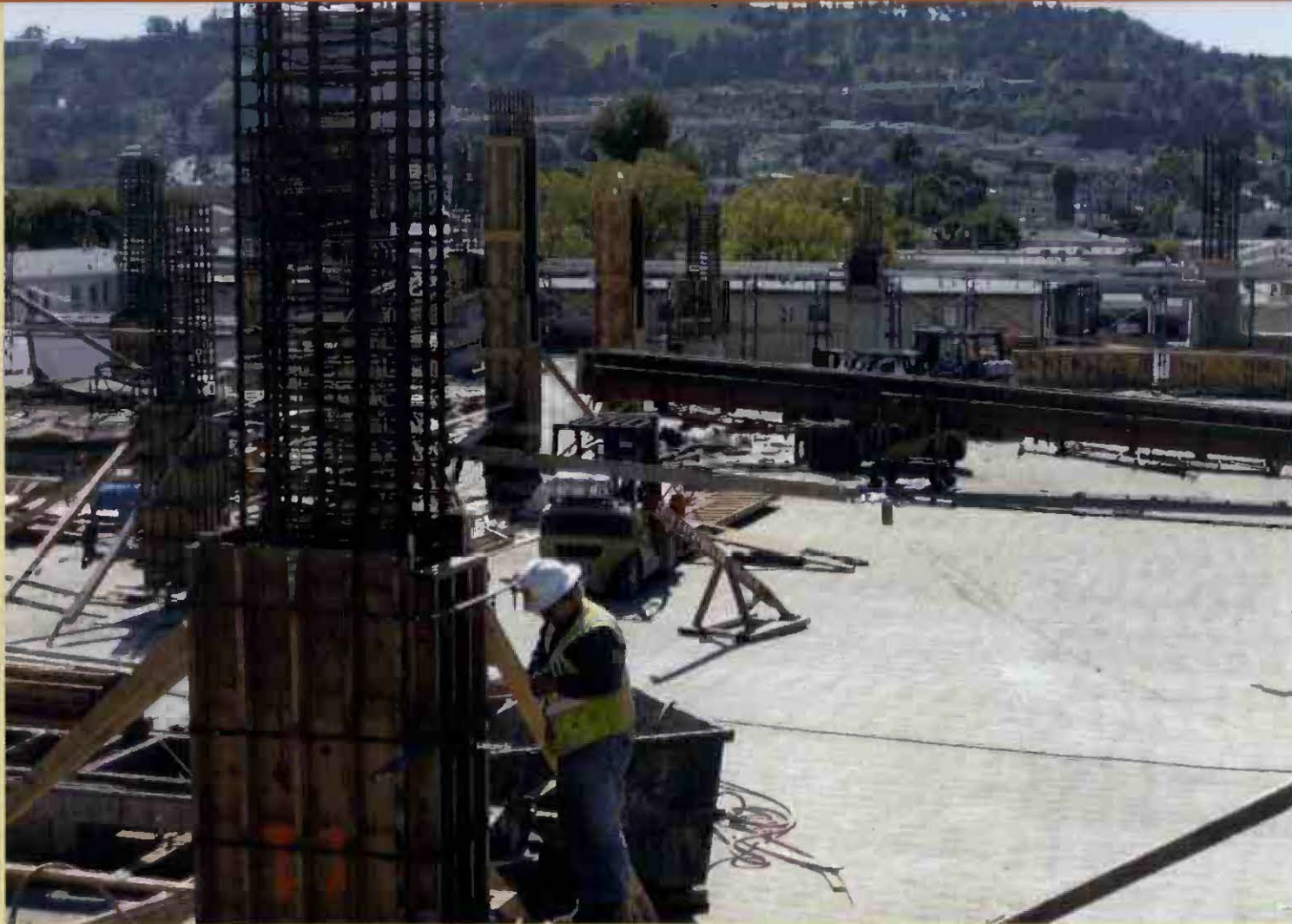
Progress on Columns for the La Cienega Parking Structure
