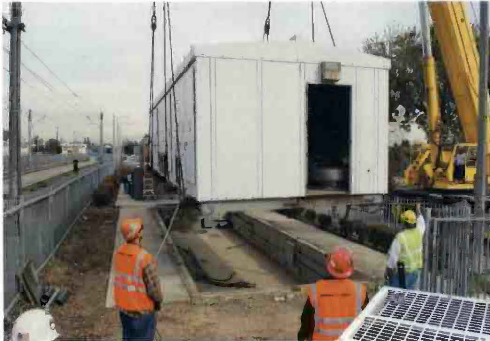
Removal of old Florence Substation on March 1, 2011
