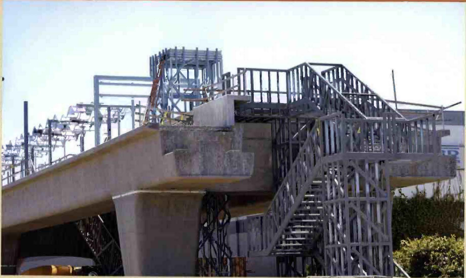
Progress at Culver City Station
