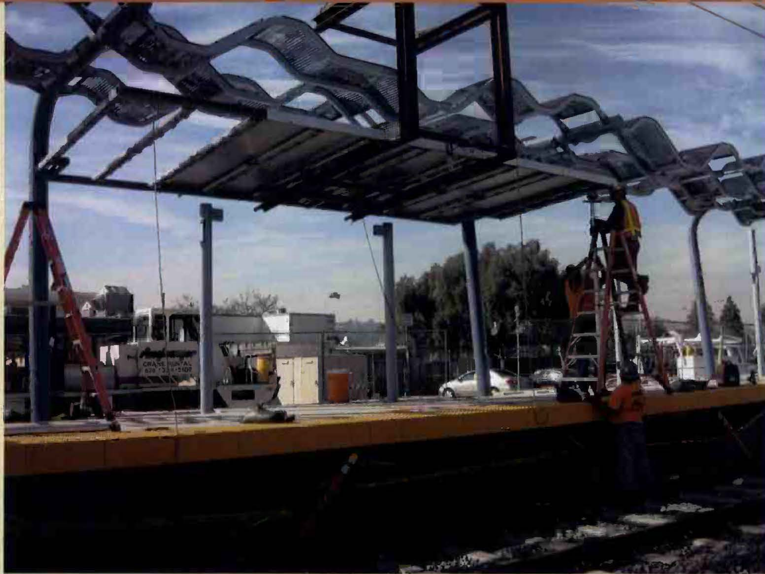
Canopy Rain Shield Installation at Farmdale Station
