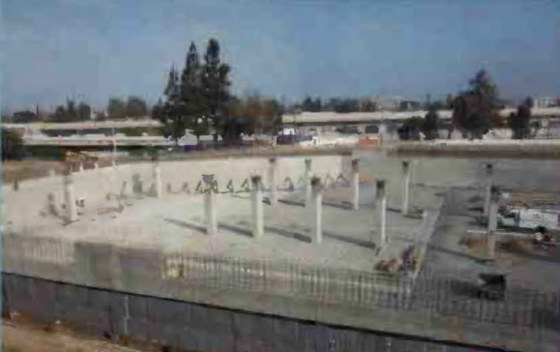
Site photo looking west
