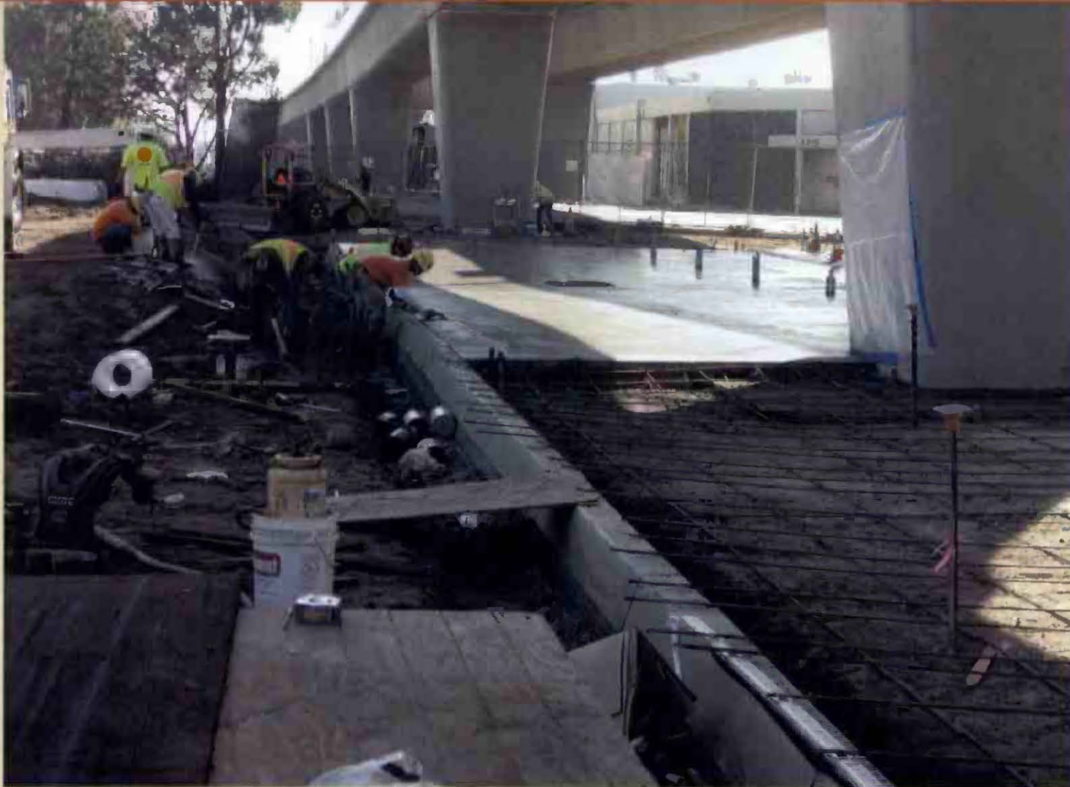
Culver City Station Plaza Concrete
