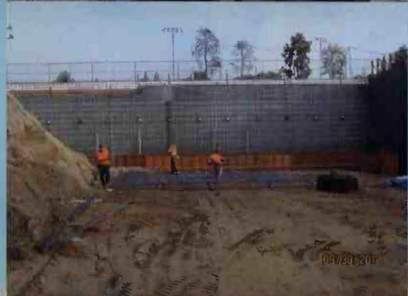
Rebar for wall panels
