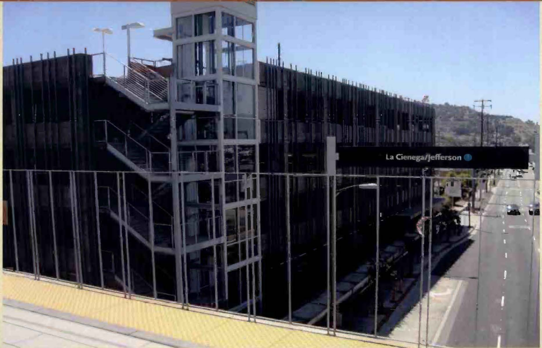
Progress at the La Cienega Parking Structure
