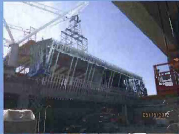
Framing for transit retail building
