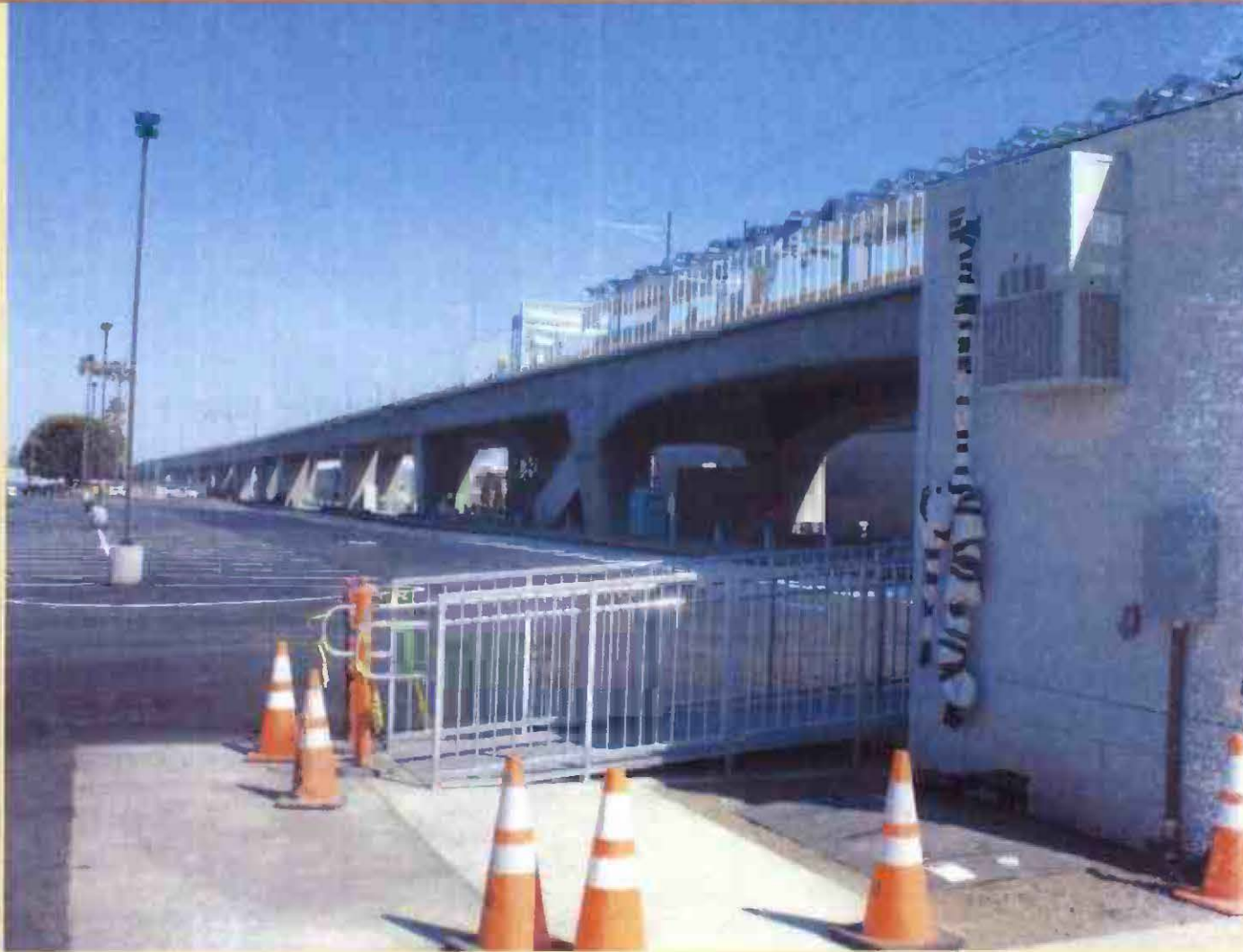
Progress of Parking Lot B at the Culver City Station
