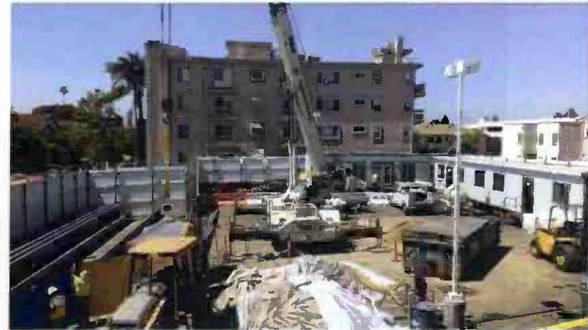
Construction site including staging and office trailers
