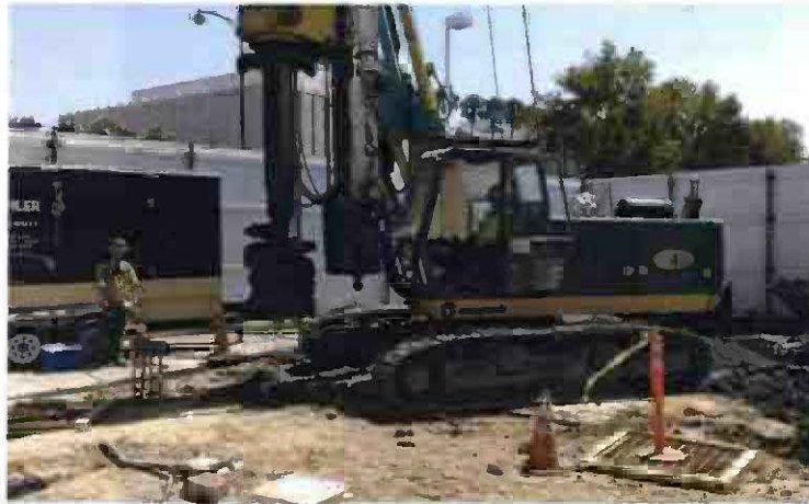
Installation of Shoring Piles
