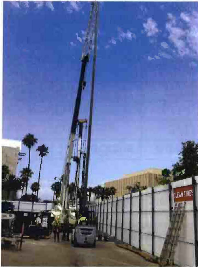
Installation of Shoring Piles
