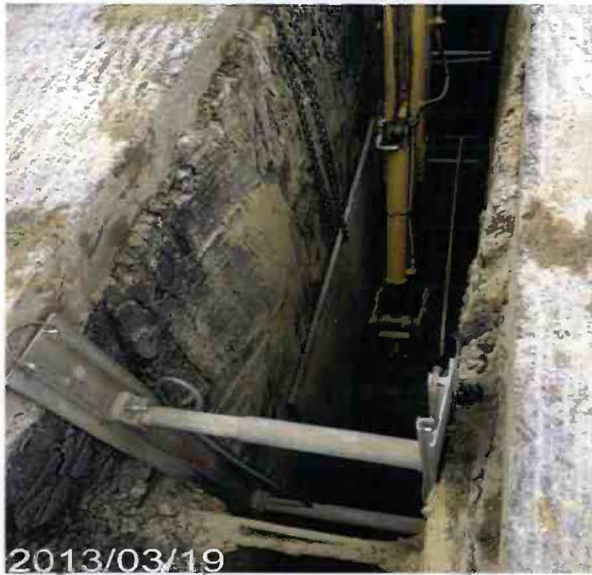
Installation of Steel Shoring Plates
