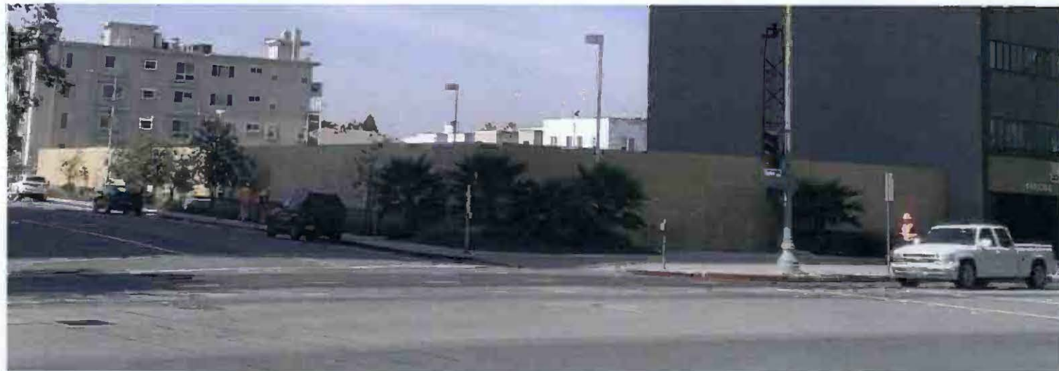
Construction of Project Fencing – Painting & Project Signage to follow
