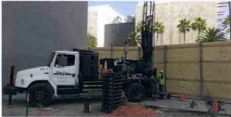
Placement of Geotechnical Instrumentation before Shaft Construction
