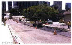
Asphalt base placement for DWP Power trench at 2<sup>nd</sup> & Hope Street.
