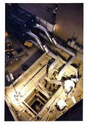
**Exploratory Shaft Contract C1034** - The temporary exploratory shaft was constructed to gather data related to soil conditions, gassy ground and ground water to assist in the geotechnical design of the Wilshire/Fairfax Station and tunnels. Risks associated with potential construction delays during the discovery and excavation of prehistoric fossils will be mitigated through planning of early construction activities.
