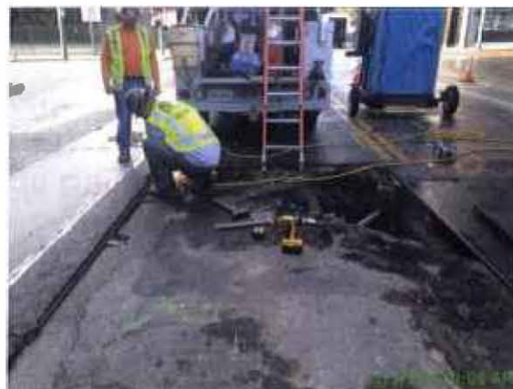
Advanced Utility Relocation – Cutting for encasement on Broadway ST.
