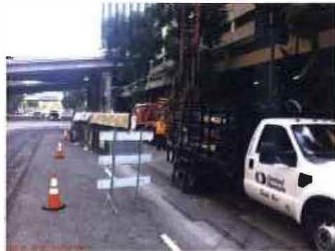
C0980 Pre-Construction work at Flower St.
