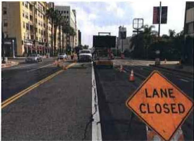
C1055 Utility Relocation Work at Wilshire/Orange
