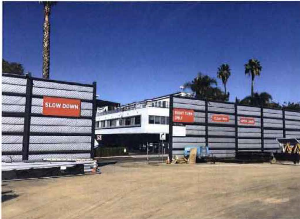
Sound Wall constructed by the C1055 Contractor at the Wilshire/Crenshaw site.
