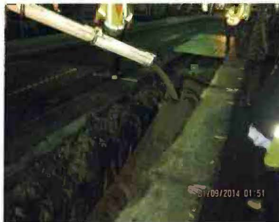
Solar Powered Generator and Slurry Backfill of Power Duct Bank
