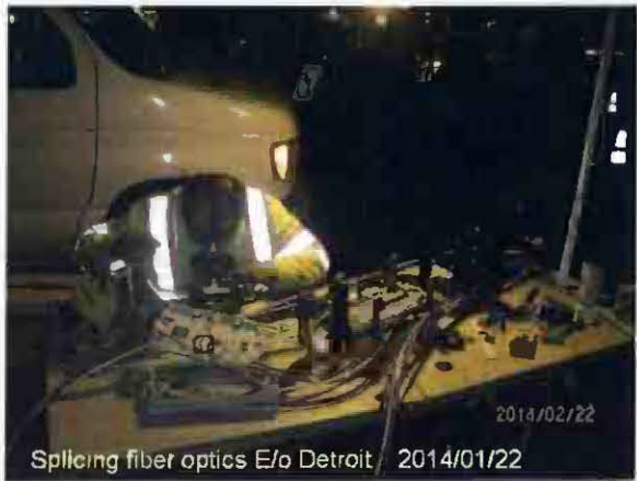
Fiber Optic Splicing and Advanced Utility Relocation work at Wilshire/La Brea
