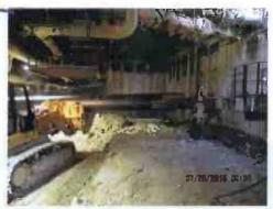
MLK STATION - Struts staged/inwork and excavation operations
