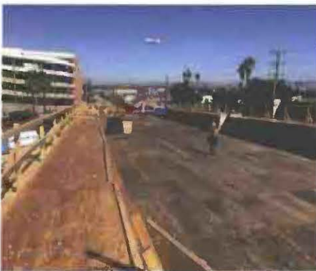
AVIATION/CENTURY – Bent cap rebar placement and Span 7 and 8 exterior girder stem and overhang formwork construction.
