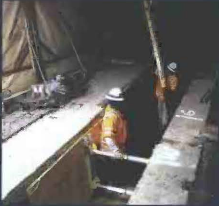
Westside Purple Line Extension Section 1 Project
