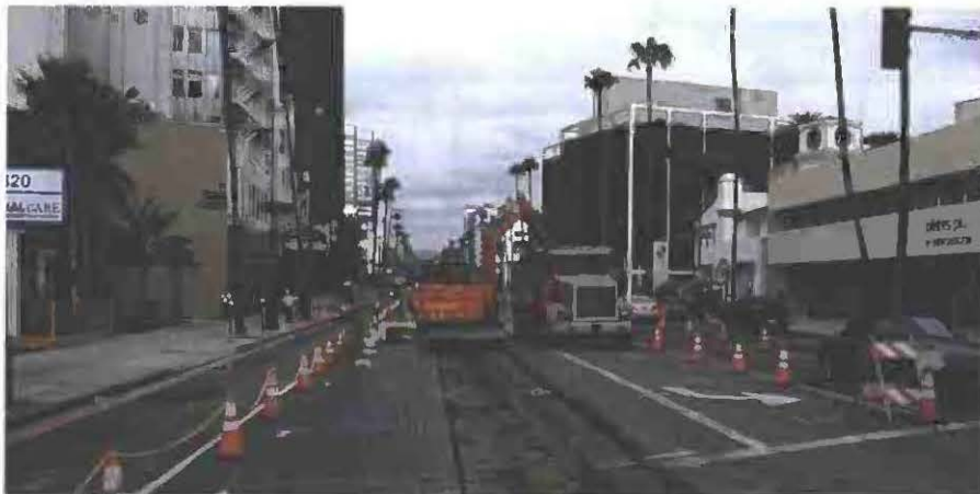
C1056 Sewer Line Trench Excavation West of Gale
