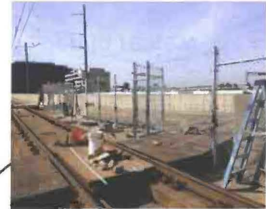
GREEN LINE – Safety barrier installation for upcoming counterweight removal and tie-in staging work
