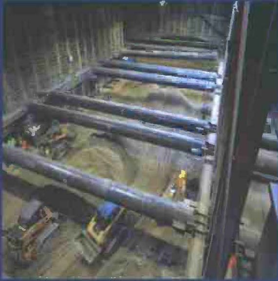
Crenshaw/LAX Transit Project
