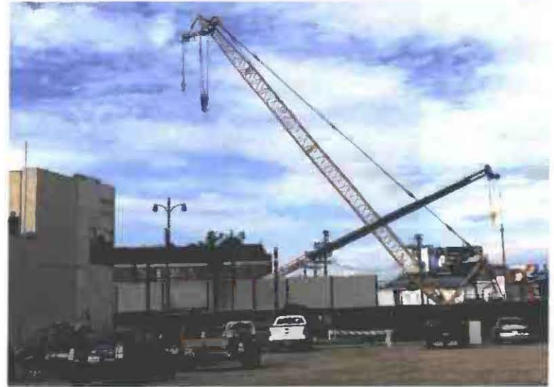
190 Ton Crane at Wilshire/La Brea staging area
