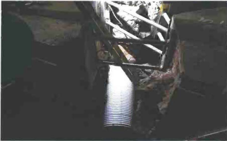
Contractor placing 24" HDPE into existing Storm drain
