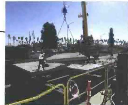
UG4 – Setting precast deck panels looking south
