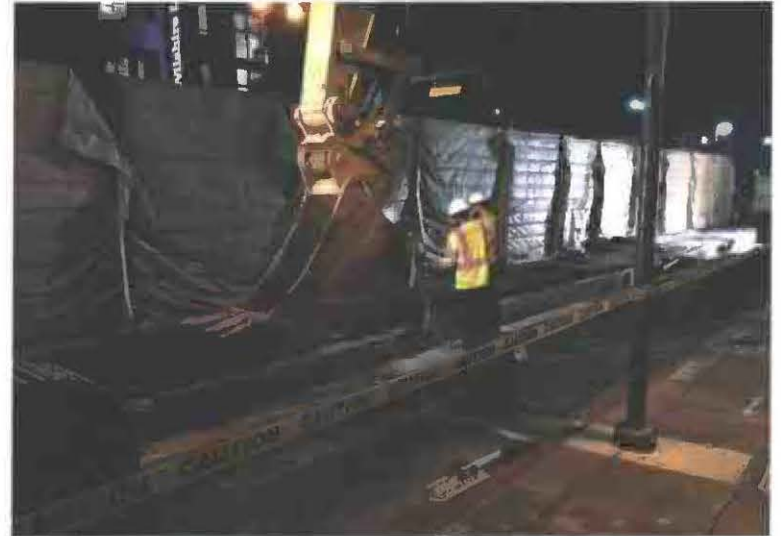
Excavating and installing trench shoring
