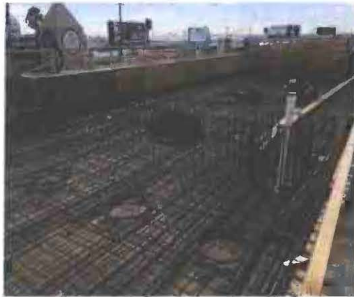
AVIATION/CENTURY – Bent cap rebar placement and Span 7 and 8 exterior girder stem and overhang formwork construction.
