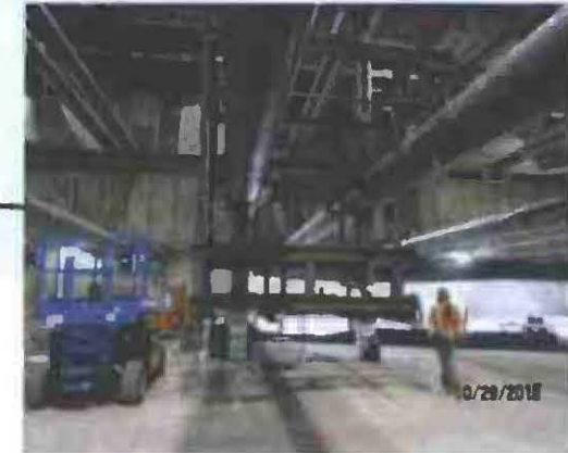
EXPOSITION/CRENSHAW STATION – Erection of construction elevator platform and installation of HCR membrane along the walls
