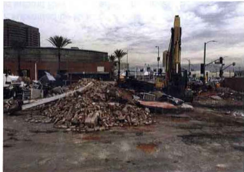
Demolition of Senior Fish Building at 1 st and Alameda Sts.
