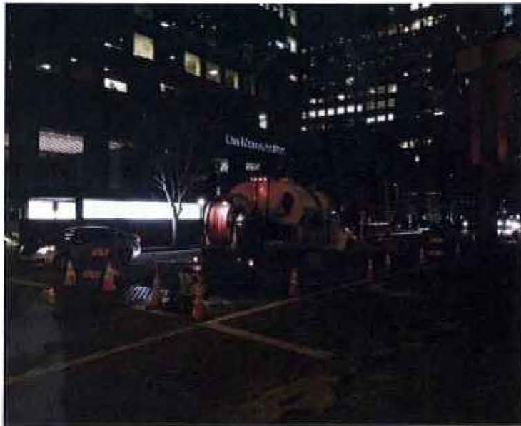
Advanced Utility Relocation – Flower St.
