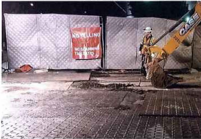
C1055 Utility Relocation Noise Mitigation Measures
