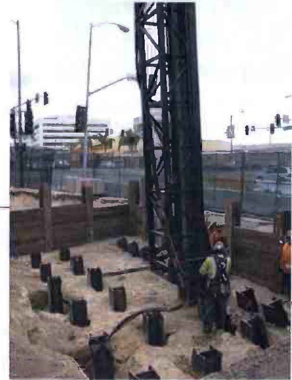
Pile Driving at La Brea Bridge Abutment 2 (East)
