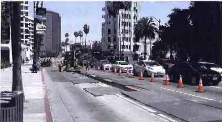
C1056 Utility Relocation Westbound on Wilshire Boulevard
