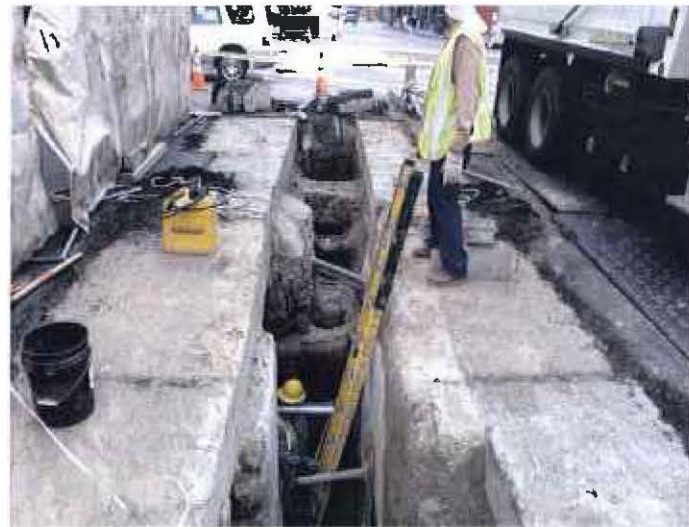
LADWP work at 6 th St. and Flower
