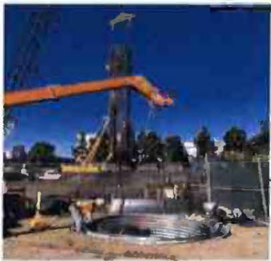
Green Line Bent 2 Isolation Casing
