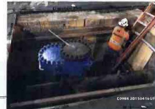
Completed Gas Line Relocation At Vernon
