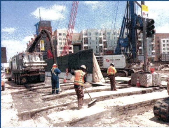
Westside Purple Line Extension Section 1 Project
