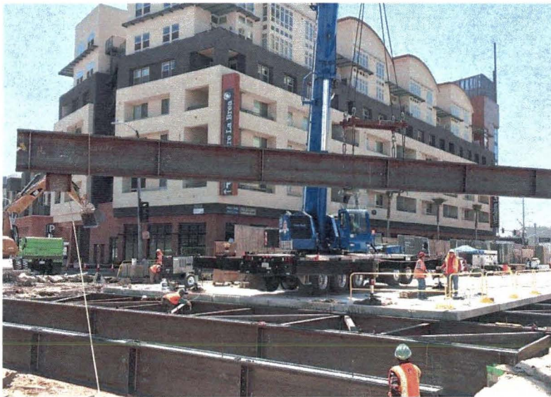
Installation of deck beams at Wilshire/La Brea Station
