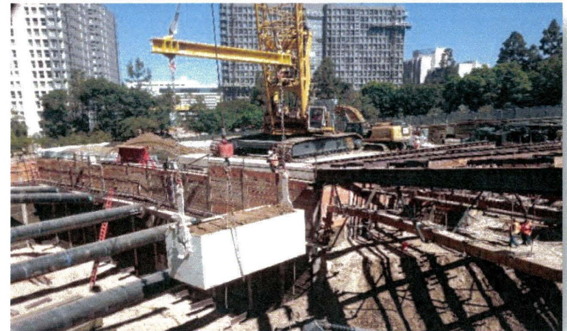
Muck removal at 2 nd /Hope Station
