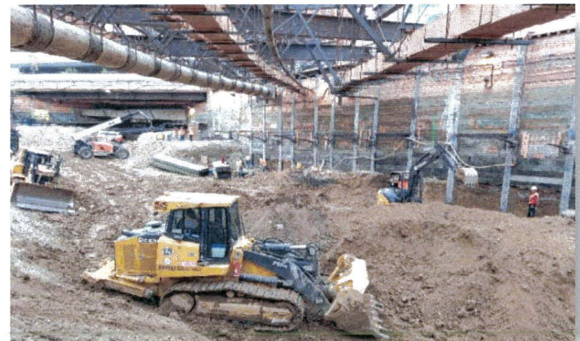
Excavation at 2 nd /Hope Station
