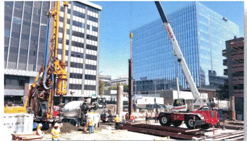
Piling at 2 nd /Broadway Intersection
