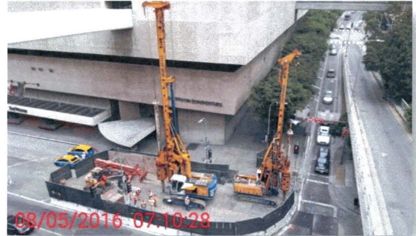
Piling setup at 4 th /Flower
