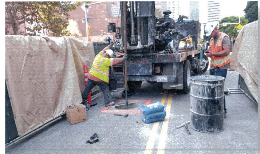
Installation of Geotechnical Instrumentation
