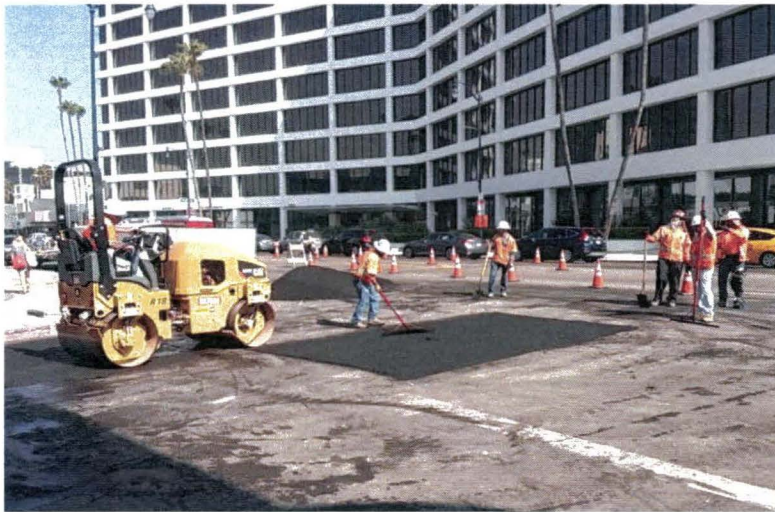
Advanced Utility Relocation paving at Tower and Wilshire
