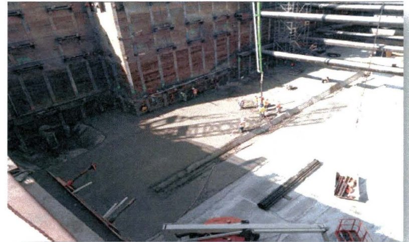
Pouring mud mat at 1 st /Central Station
