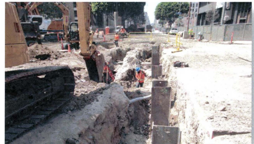
Cap beam excavation at 2 nd /Broadway
