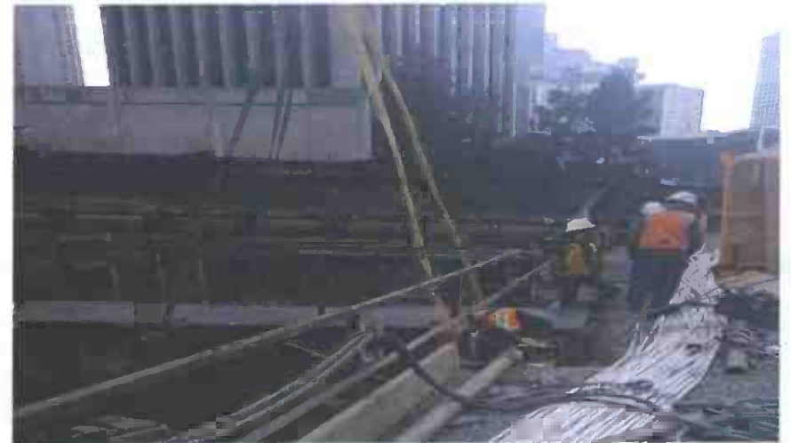
Installation of temporary Alimak manlift system 8
