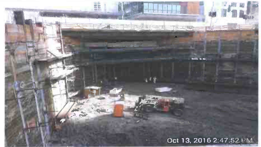
Installation of 3 rd Level walers below Hope Street decking
