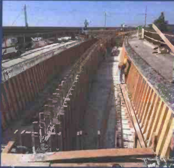
Crenshaw/LAX Transit Project
