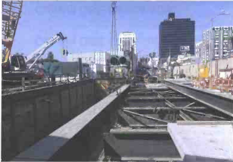
Work at the La Brea Station site - South Muck Shaft
