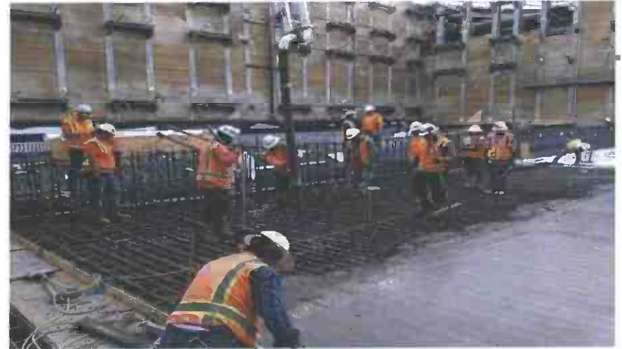
Concrete pours of invert slab
