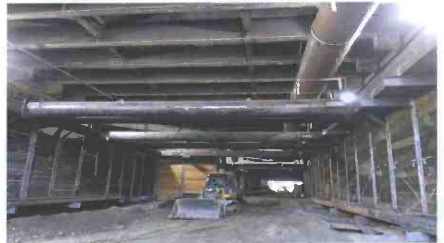
Continued excavation at Wye
