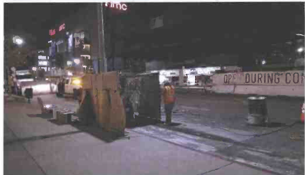
Joint Trench Construction at Constellation Blvd
