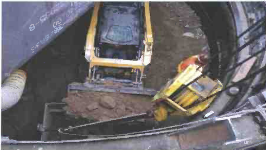
Excavation at Tie-Back Removal Shaft
