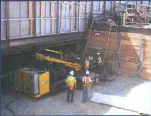
Westside Purple Line Extension Section 1 Project
