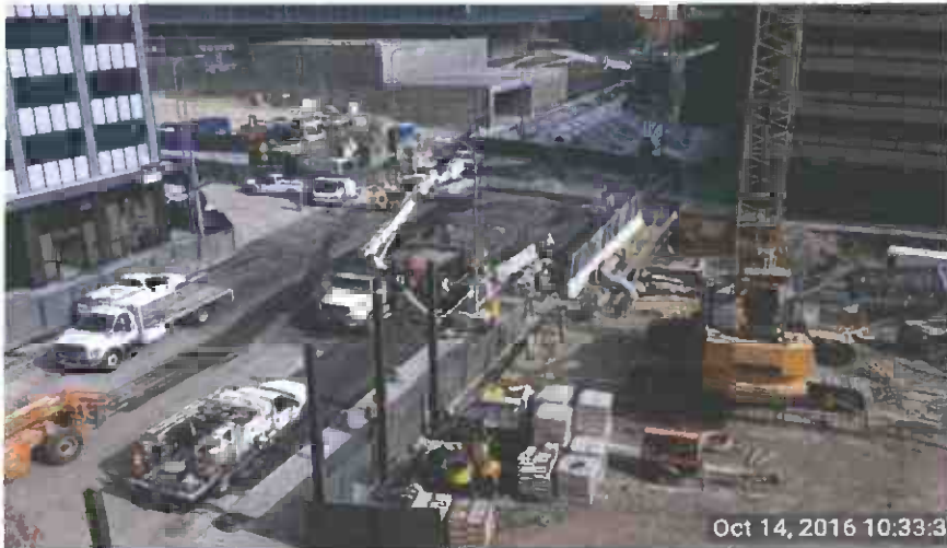
2 nd /Broadway restoration in preparation for street re-opening
