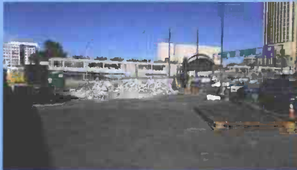
Median Barrier Demolition Debris
