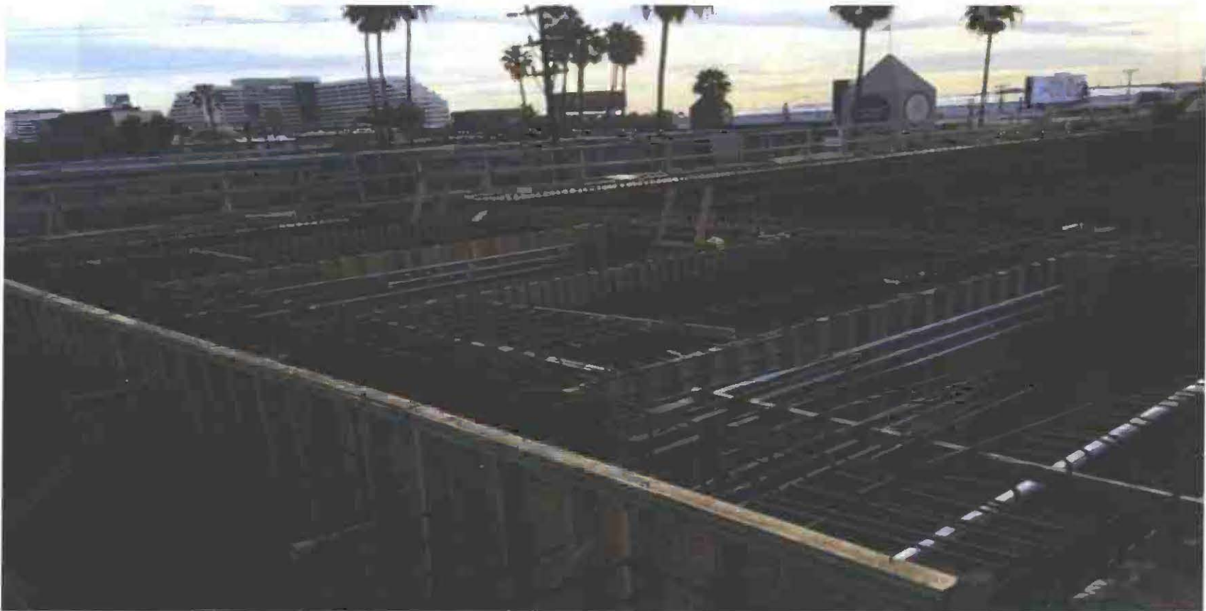
Aviation/Century Bridge – Hinge restrainer sleeves and girder stem formwork installed
