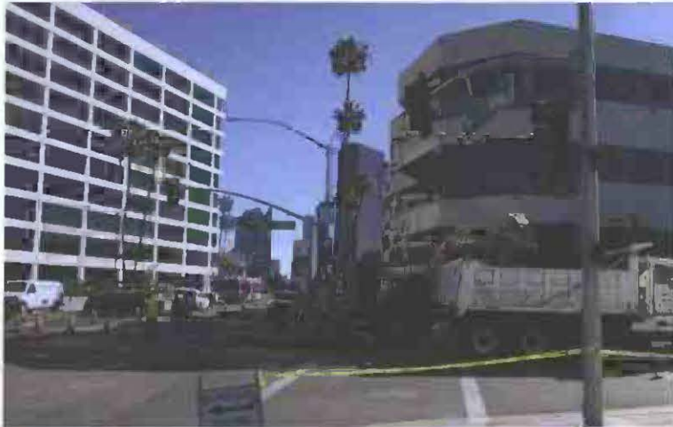
Gas Line Relocation at Wilshire/Gale
