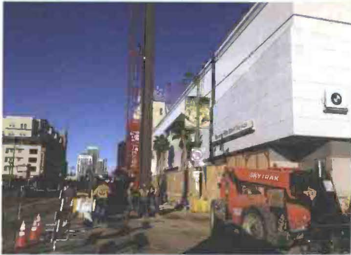
Contractor Lowering Wilshire/La Brea Station Pile #115
