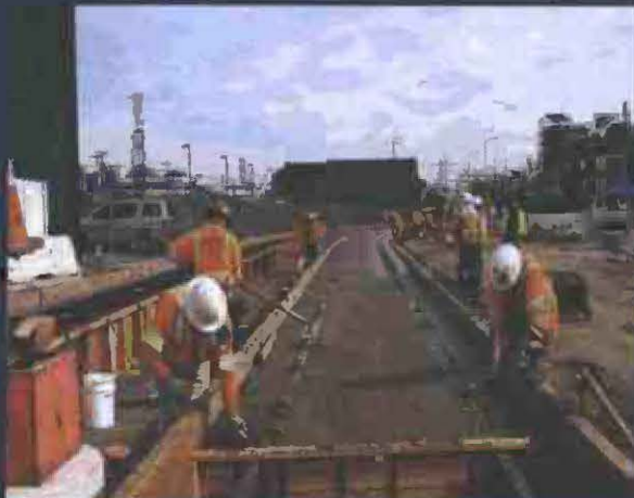
Regional Connector Transit Corridor Project
