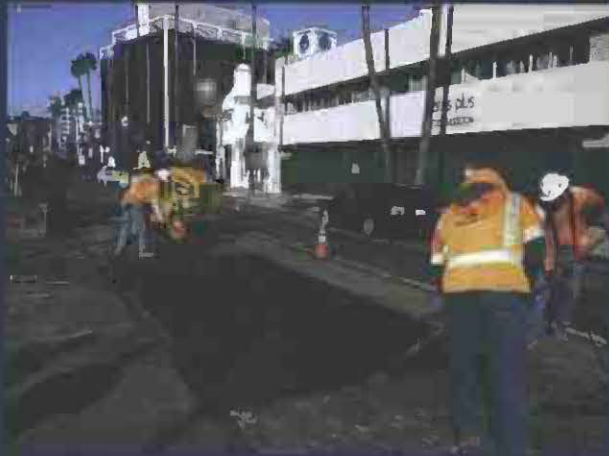
Westside Purple Line Extension Section 1 Project
