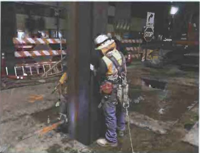
Contractor Lowering Wilshire/La Brea Station Pile #117
