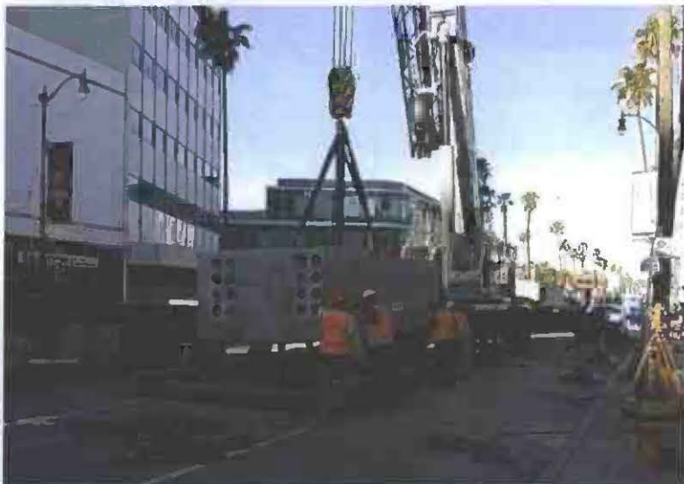
Installing SCE Electrical Vault West of La Cienega Blvd.
