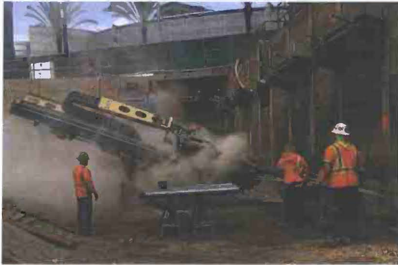
Tie back drilling ↑ and bracing struts ↓
