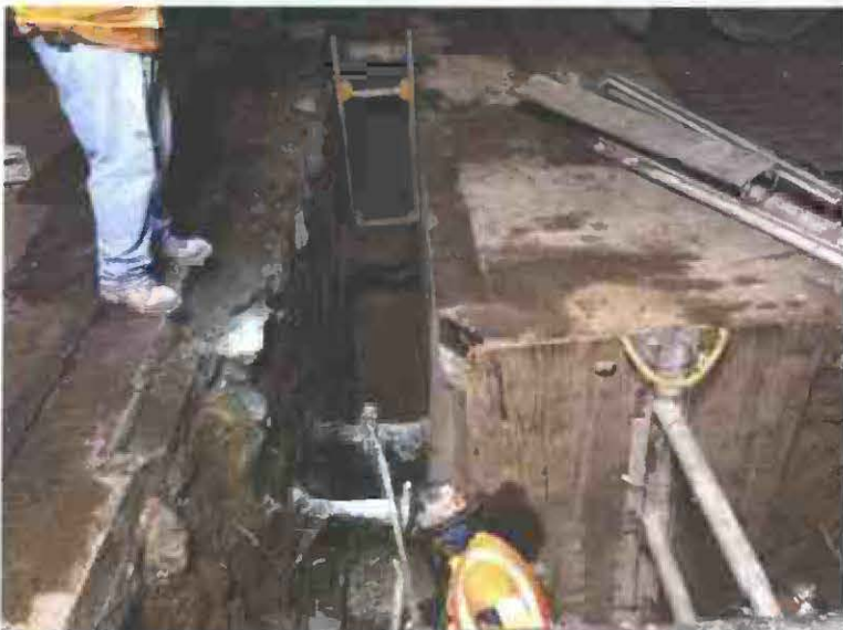
C1056 Contractor potholing sewer lateral
