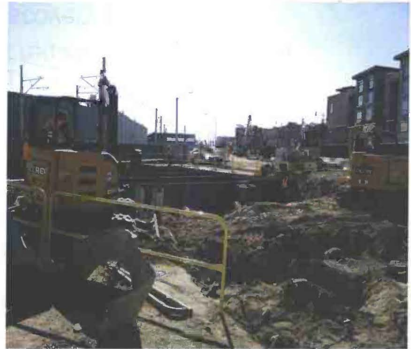
Decking at east of Alameda
