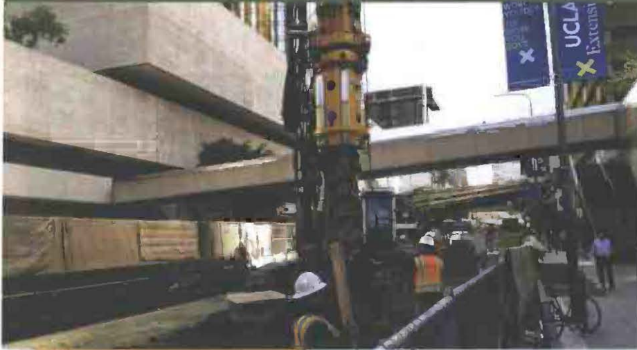
Pile Drilling
