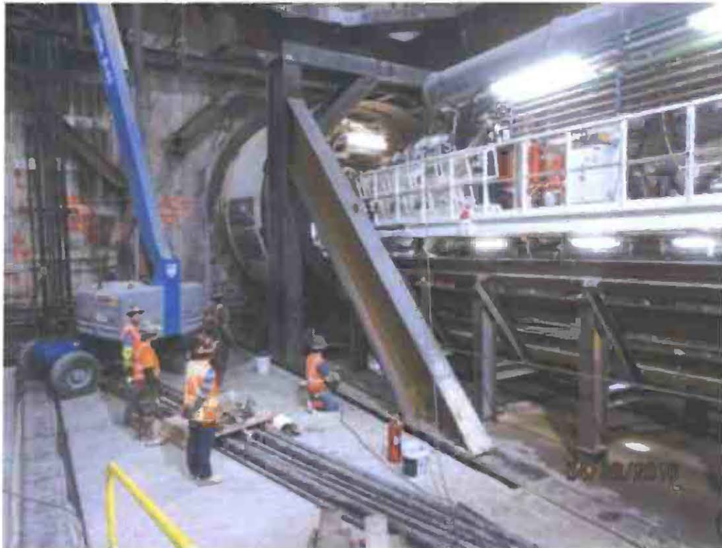
EXPOSITION/CRENSHAW STATION – Advancing TBM and thrust frame
