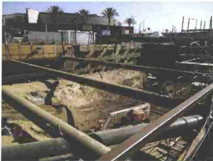
Tie back drilling ↑ and bracing struts ↓
