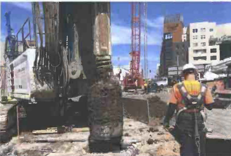
South side Wilshire/La Brea Station Pile installation
