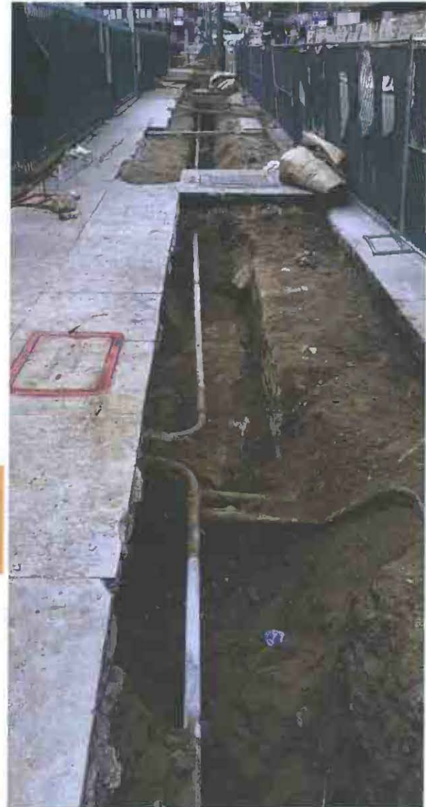
Intercept work and cable pulling
