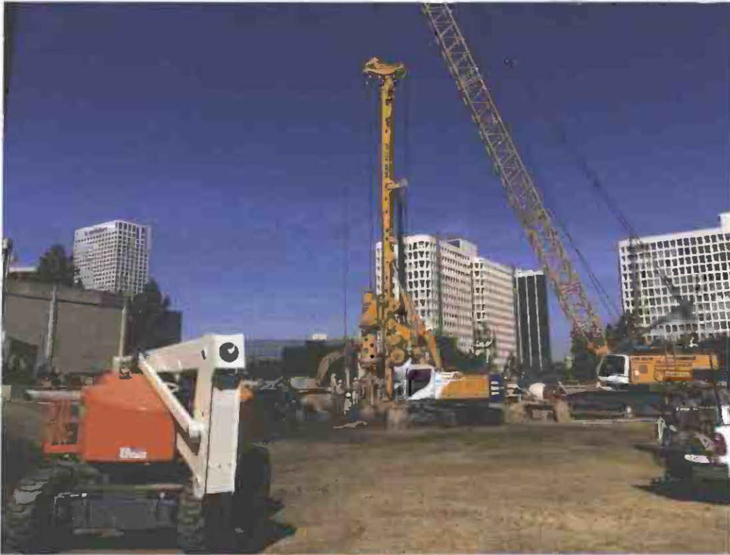
Drilling for Piles
