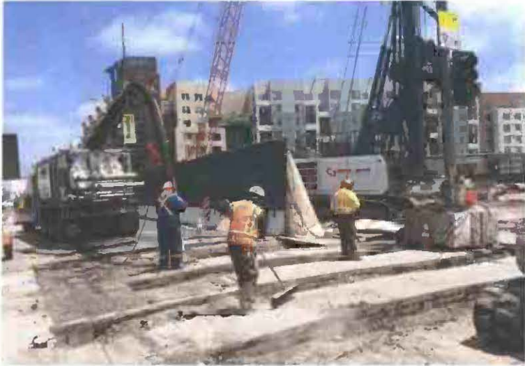
Jet Grouting Preparation at Wilshire/Detroit
