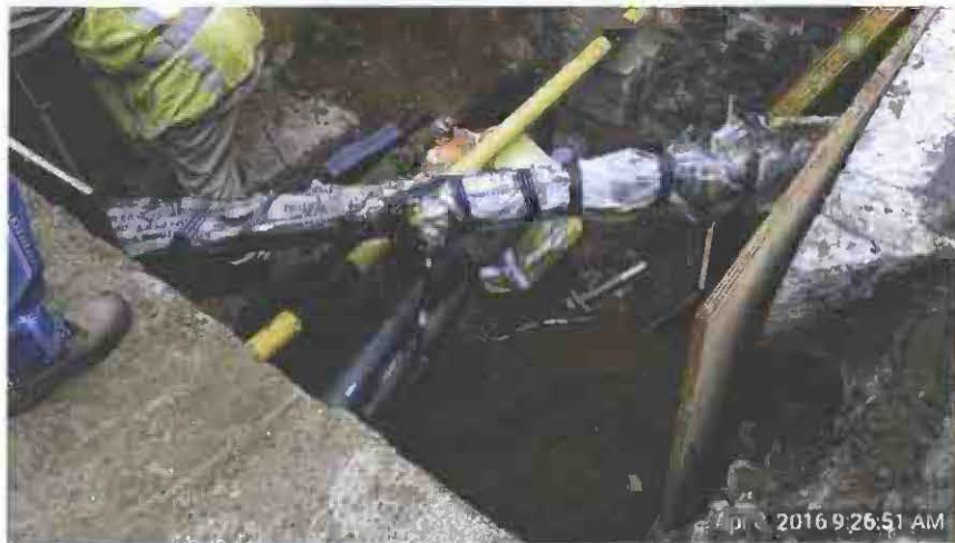
Intercept work and cable pulling
