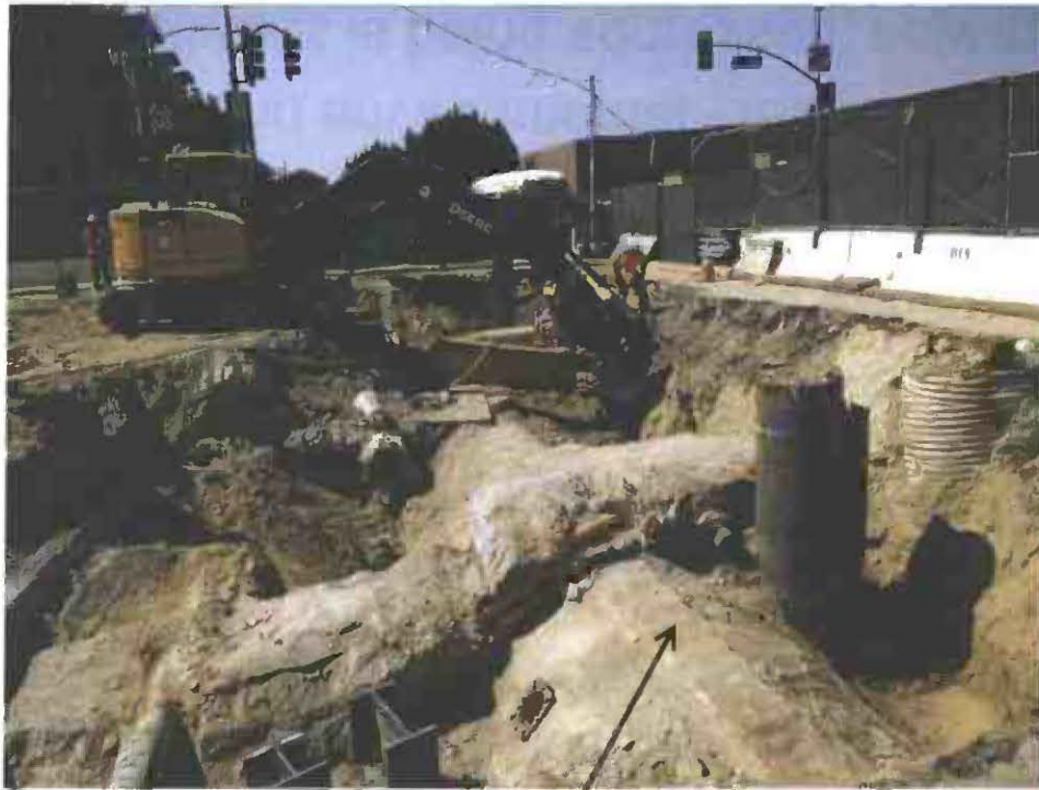
75" storm drain that will be replaced with a new one
