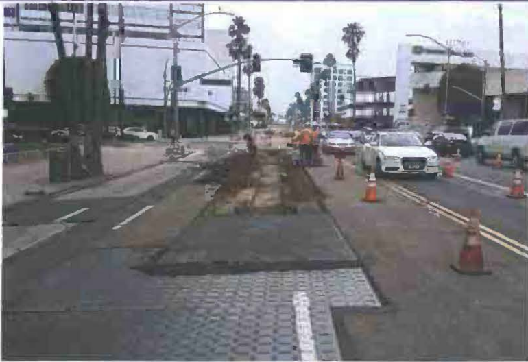
C1056 Contractor preparing waterline trench
