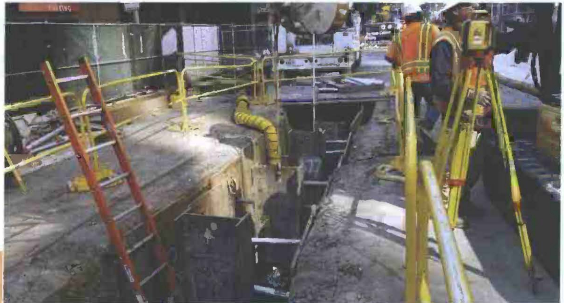
Exposing piles in preparation of cap beam installation
