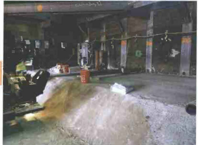
Compensation grouting →
