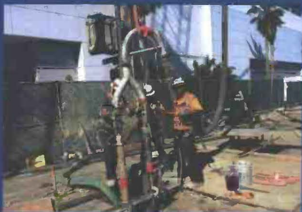
Westside Purple Line Extension Section 1 Project
