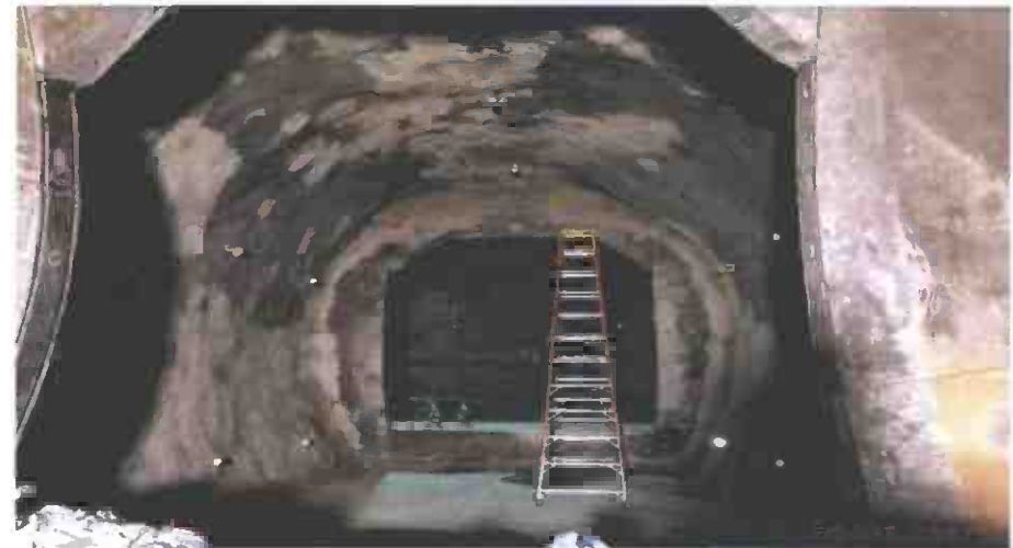
Tunneling – Cross Passage #3 ready for waterproofing
