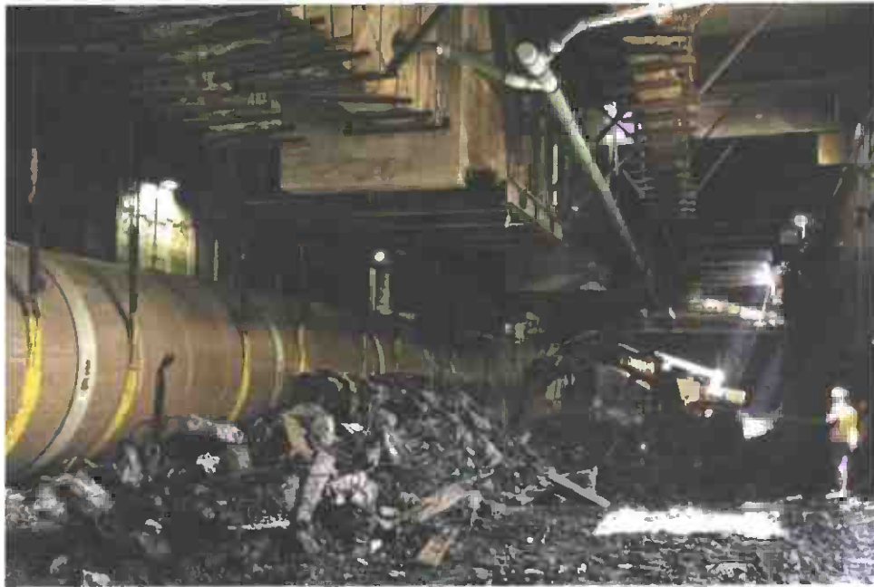
LA County storm drain demolition adjacent to Hobas replacement
