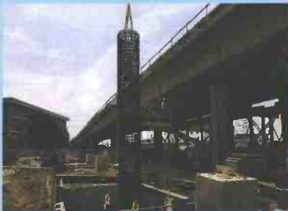
Column cage at Bent 6
