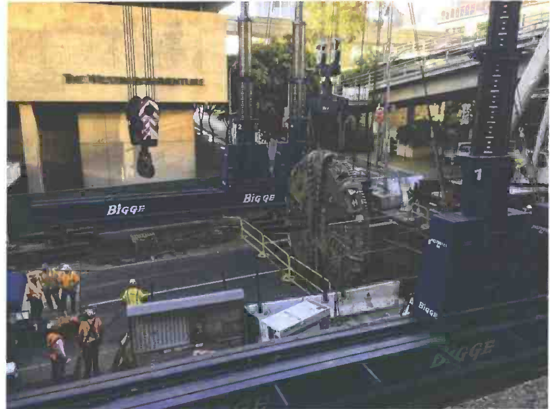
TBM cutter head extraction at TBM Retrieval Shaft
