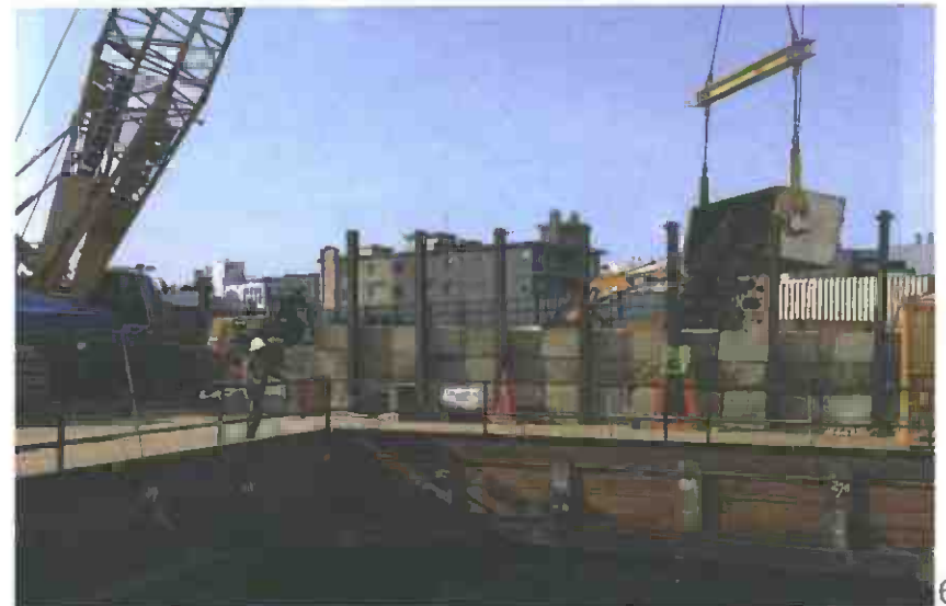
Muck Shaft at Wilshire/Fairfax Station
