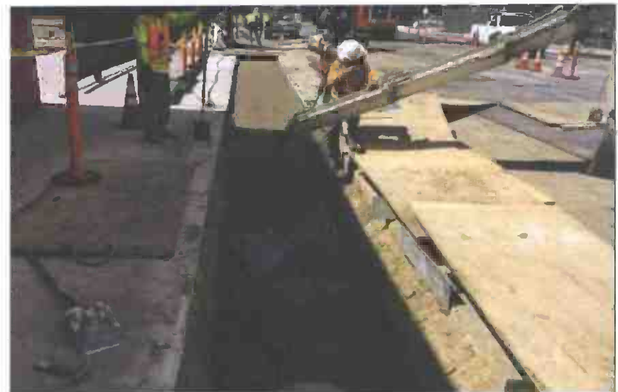
New 24 inch Storm Drain Slurry Backfill
