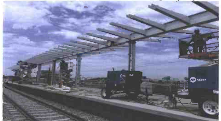
La Brea at Grade Station – Canopy frame erection underway
