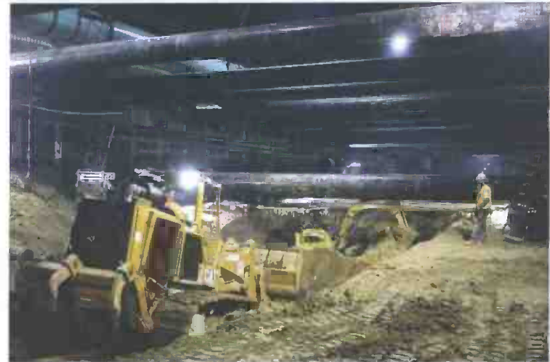
Wilshire/La Brea Station Level C Excavation
