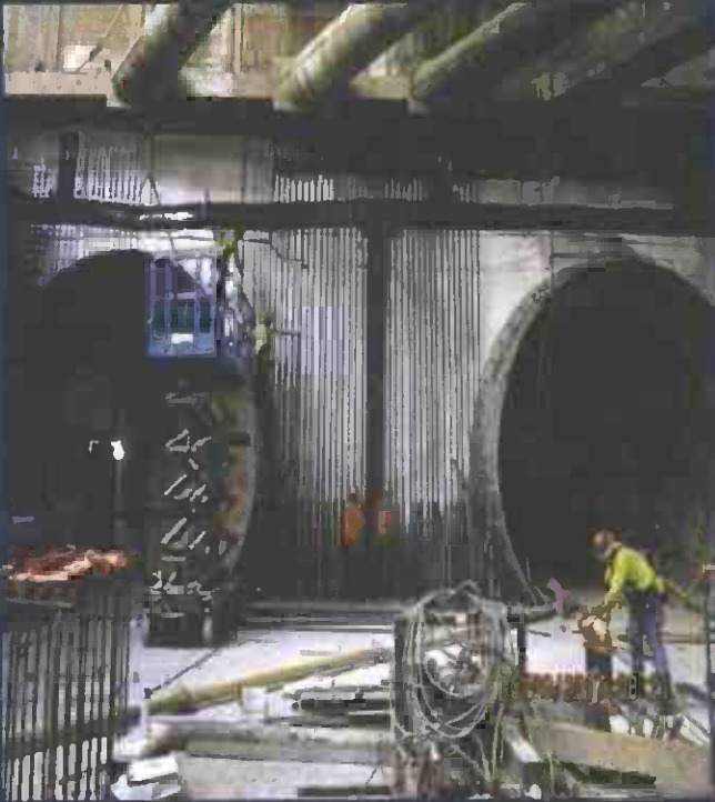
Crenshaw/LAX Transit Project
