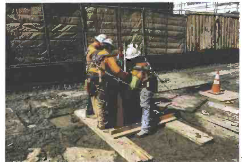
Setting Steel Beam at Wilshire / La Cienega Station
