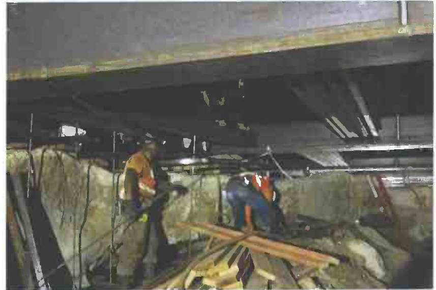
Installing Hanger Supports at Wilshire/Fairfax Station
