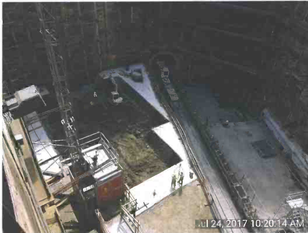
Hope Concourse Level SOG – grade to subgrade
