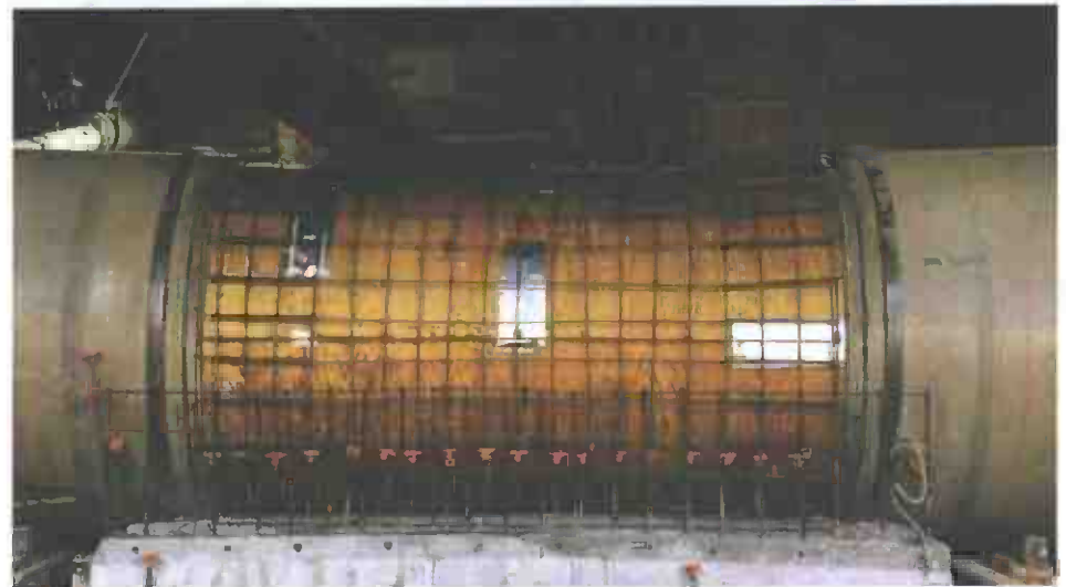
Hobas transition structure rebar Installation
