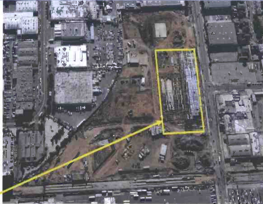
Aerial view of Southwestern Yard construction site as of mid-July 2017
