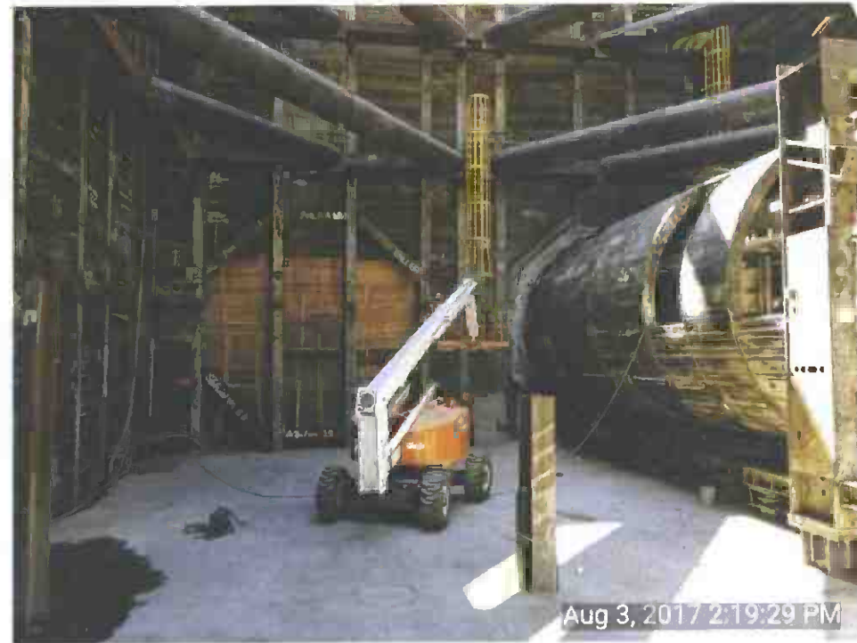
Welding barrel ladder at west end of station
