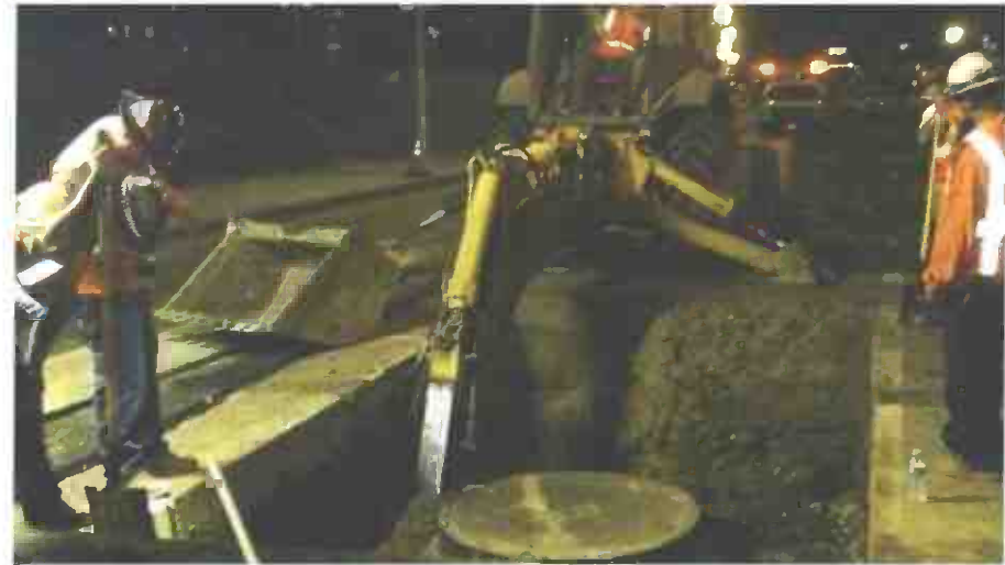
Excavating Main Line at XO Vault
