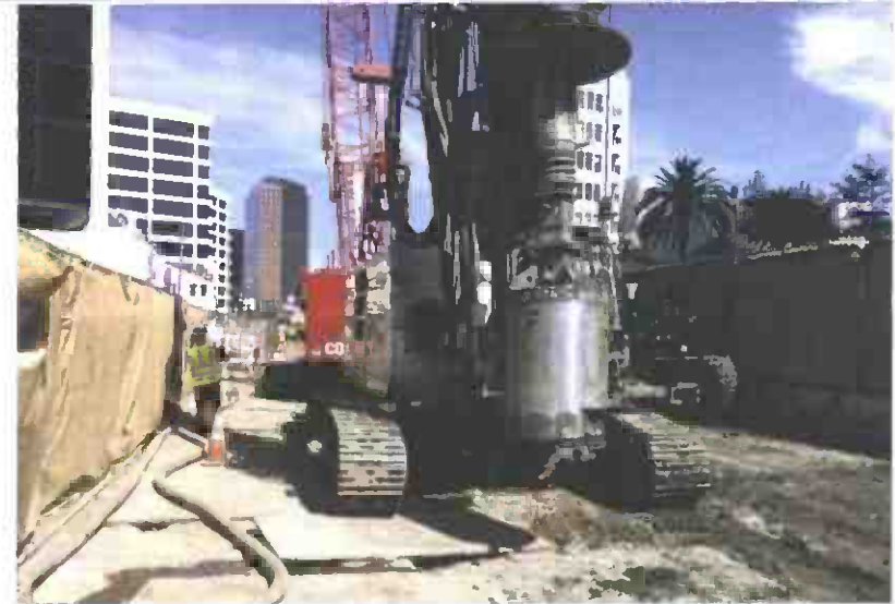
Drilling Piles at Wilshire/La Cienega Station
