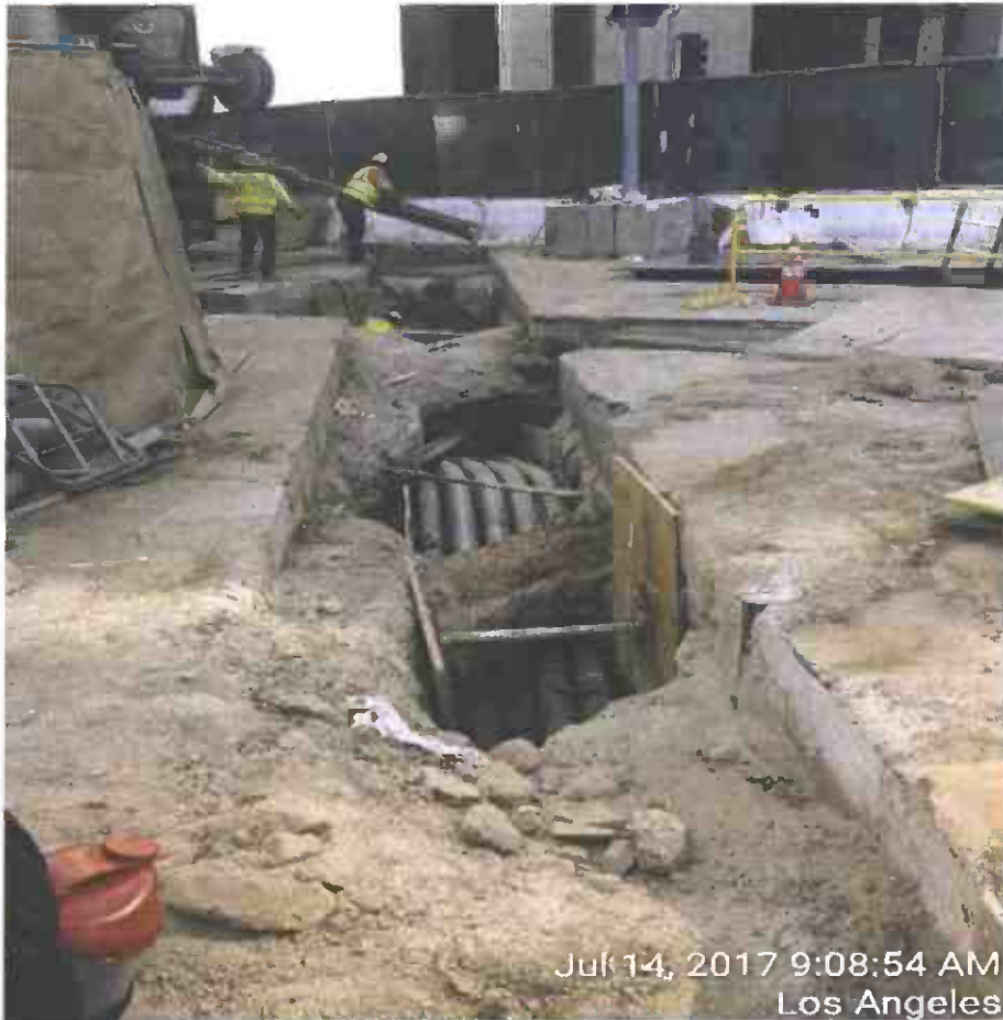
Pouring concrete encasement for Lateral 5, Mainline 8, and Lateral 5-1 junction
