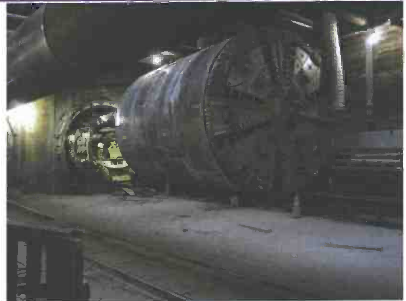
Metro Gold Line TBM
