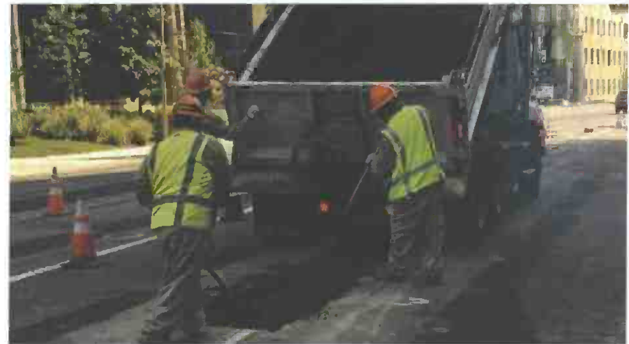
LADWP Power relocation work in Century City
