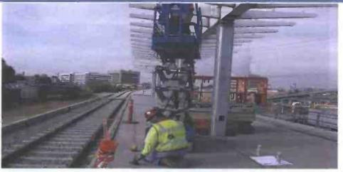
LA BREA AT GRADE STATION – Completed canopy outrigger welding and electrical and plumbing installations
