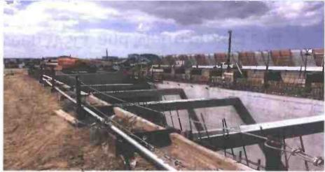
UG#1- Concrete barrier formwork installation on the west U-wall STA 50+00 to 50+38
