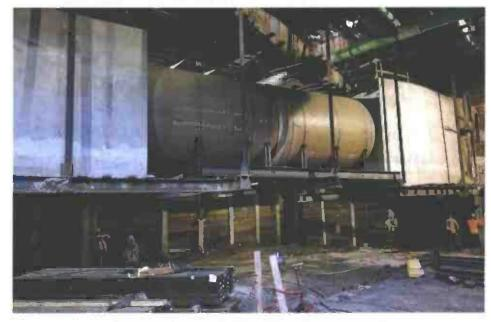
Bracing of storm drain pipe near Spring Street
