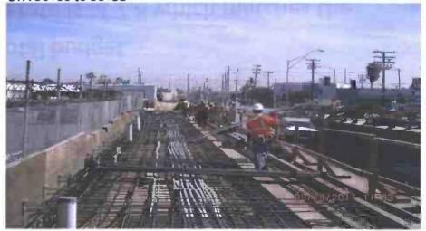
WESTCHESTER/VETERANS STATION – Crew worked on installation of anchor bolt and blockouts
