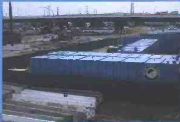
Industrial Waste Tanks
