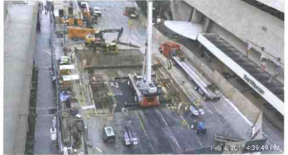
Installation of deck beams across Flower Street
