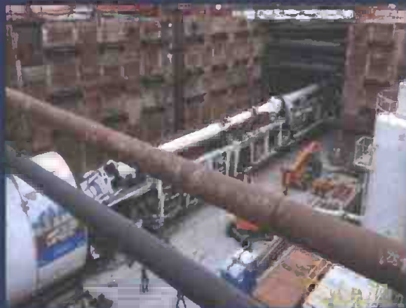
Regional Connector Transit Corridor Project
