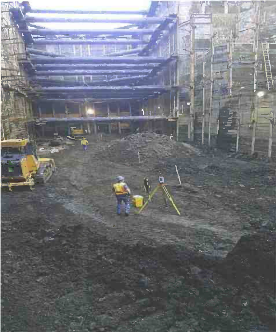
Surveying grades to invert at west end of station
