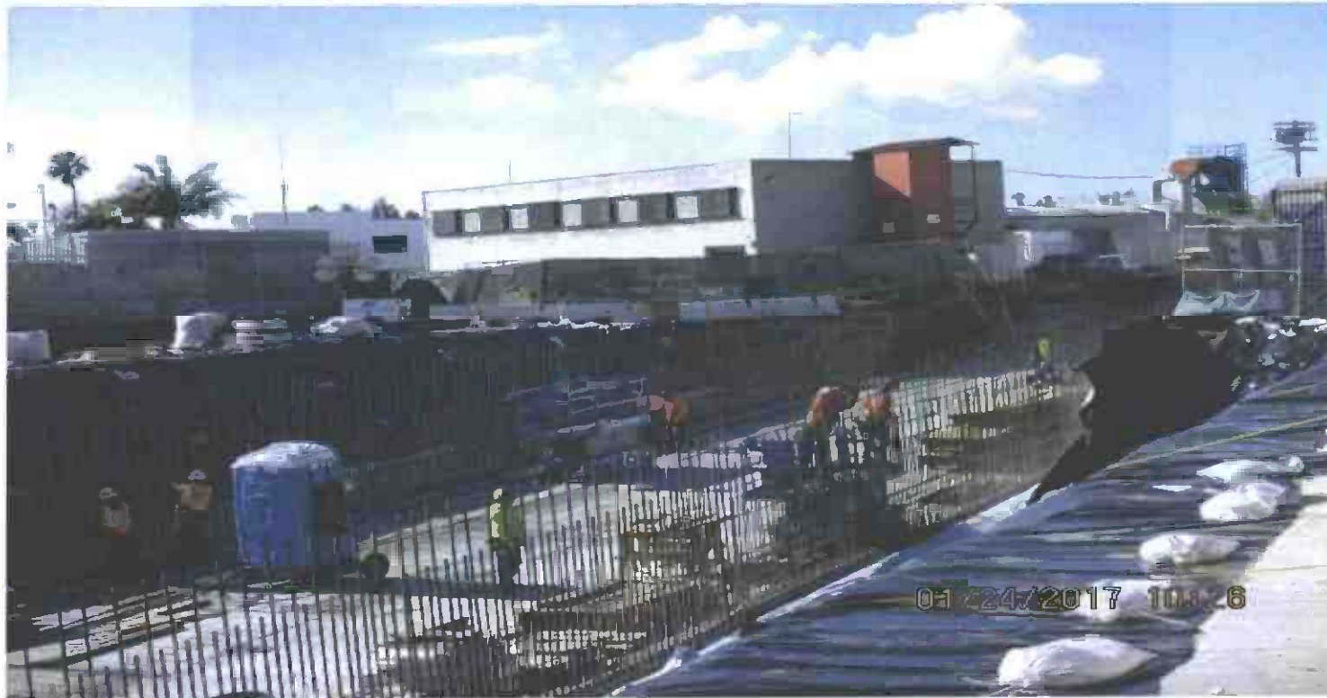
Underground Structure #3: Installation of rebar for u-channel walls at south portal.
