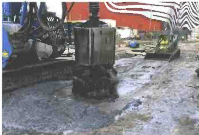
Pile operations at Wilshire/Fairfax Station along south Wilshire Boulevard
