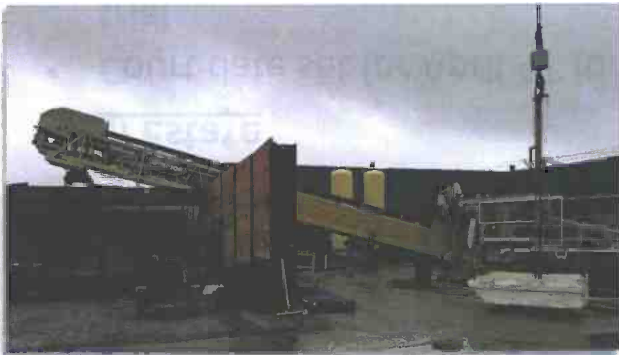
Muck conveyor at Mangrove/Launch Pit
