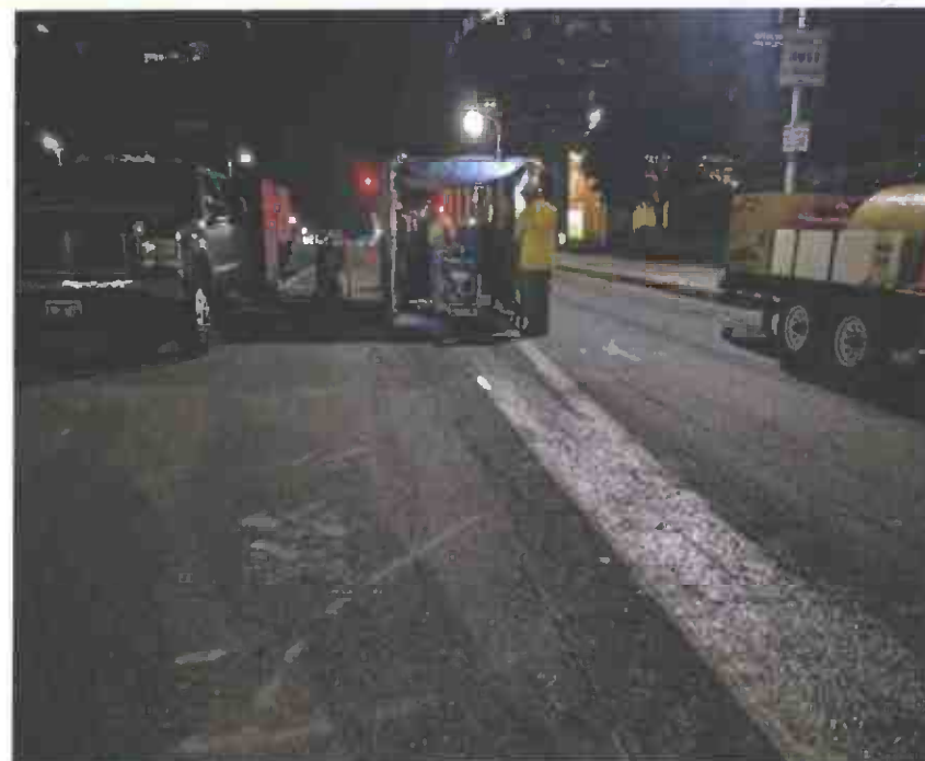
Joint Trench Construction at Constellation Blvd / Avenue of the Stars
