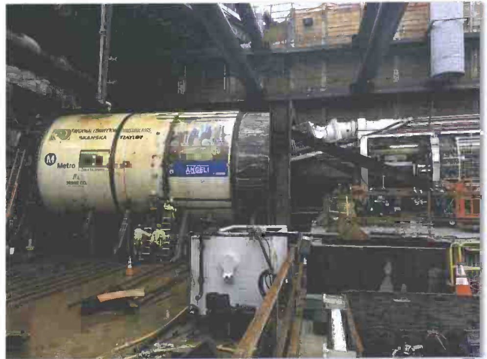
TBM final preparations for launch
