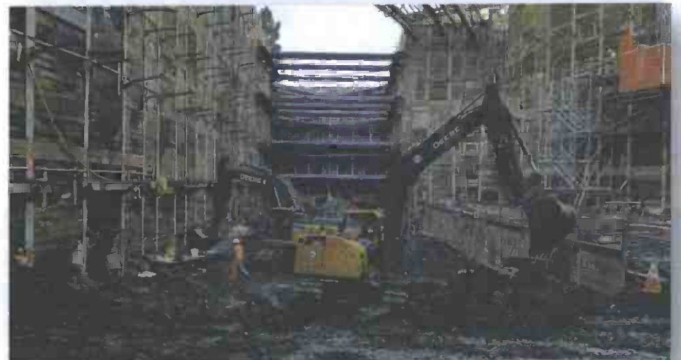
Excavation and lagging at station center
