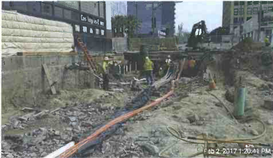
Excavation and utility exposure on 2 nd Street
