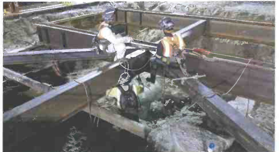
Welding of deck beams
