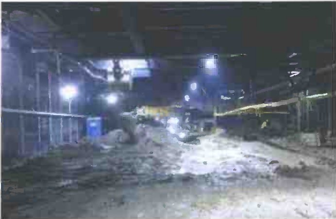
Wilshire/La Brea Station excavation under the deck
