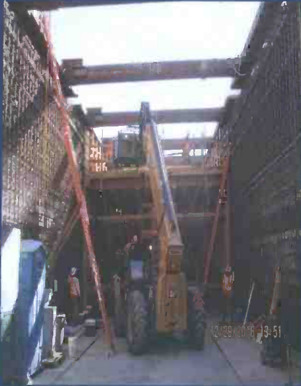
Crenshaw/LAX Transit Project
