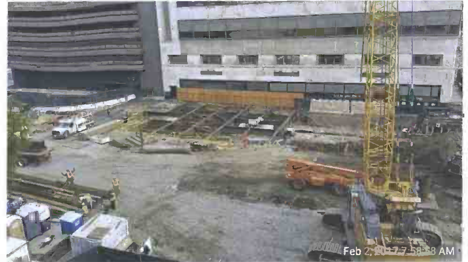
Deck beam installation on 2 nd Street
