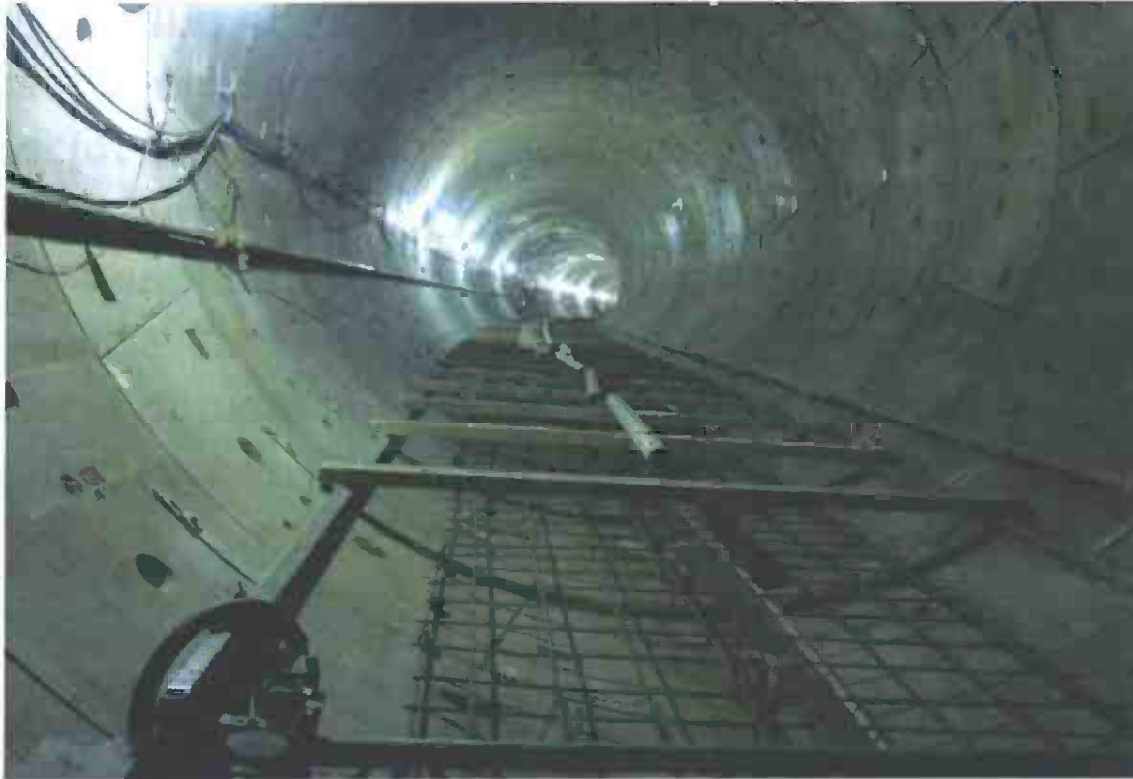
Installation of electrical conduits south bound tunnel invert rebar.
