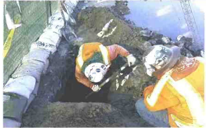
Clark Construction Group/Gruen Associates 30% Design Submittal Clark Murray Potholing Waterline for proposed Storm Drain
