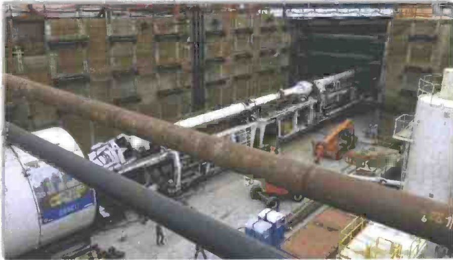
TBM assembly
