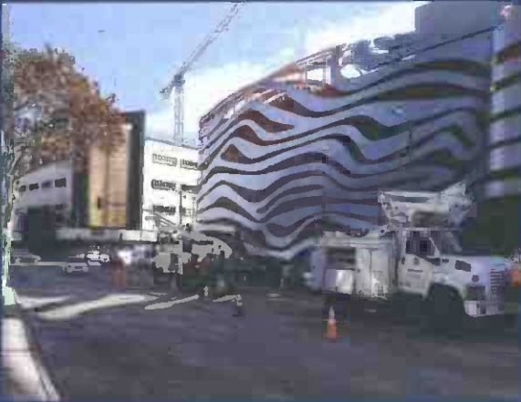
Westside Purple Line Extension Section 1 Project
