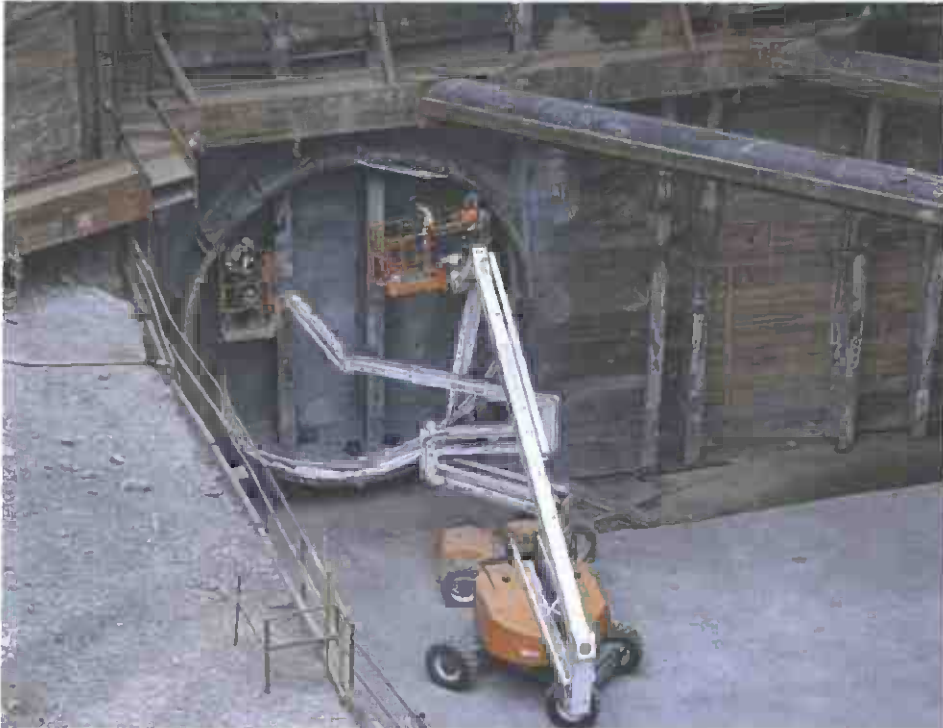
Applying Shotcrete on East Tunnel Eye Left Track
