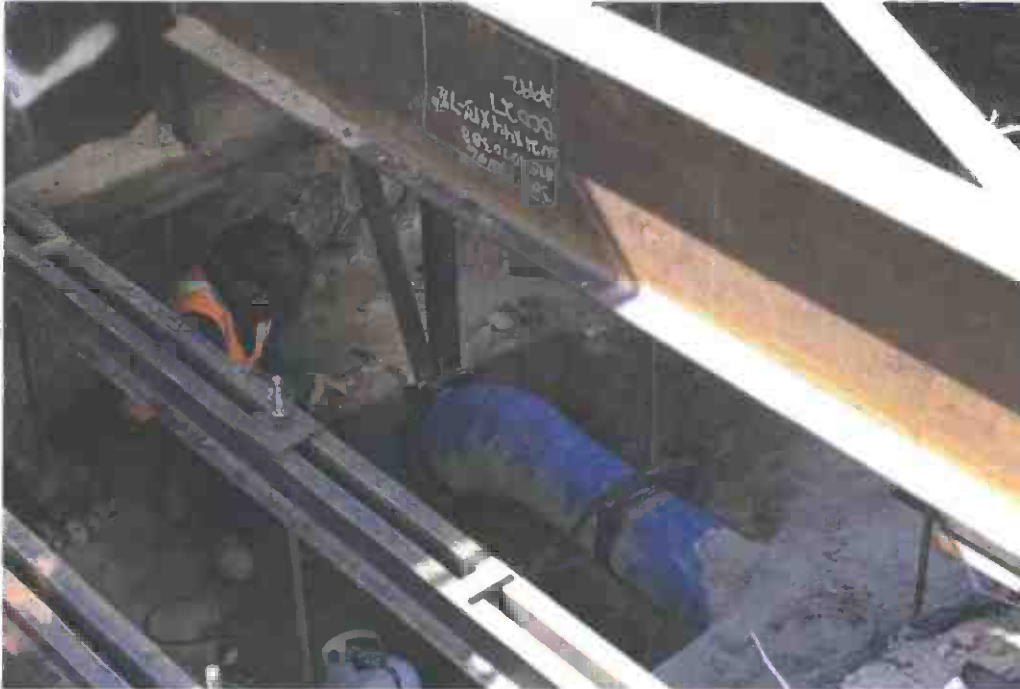
Utility hanging along the north side of Broadway SOE
