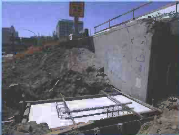
Abutment 1 Foundation Poured
