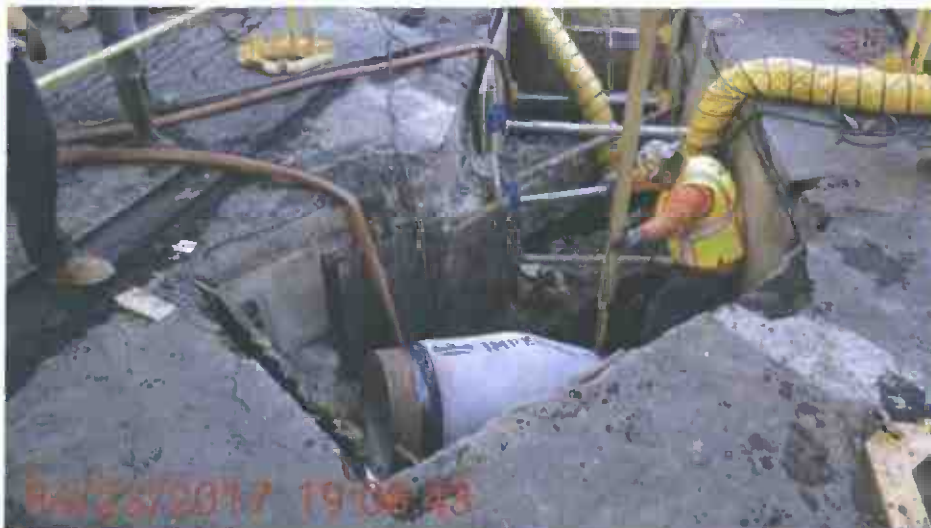
Water-line tie-in work on Flower Street
