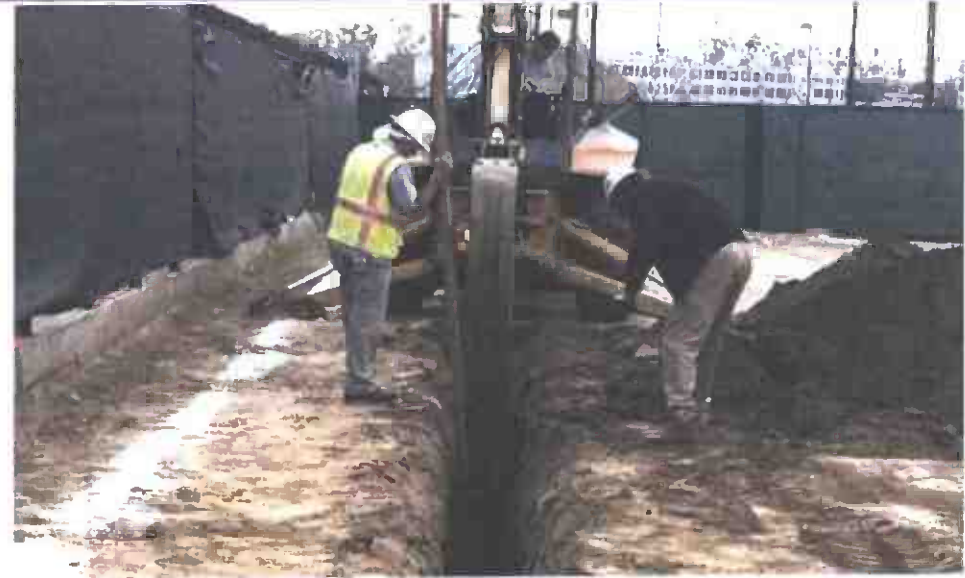
Sewer Line Excavation for 6 inch PVC Pipe
