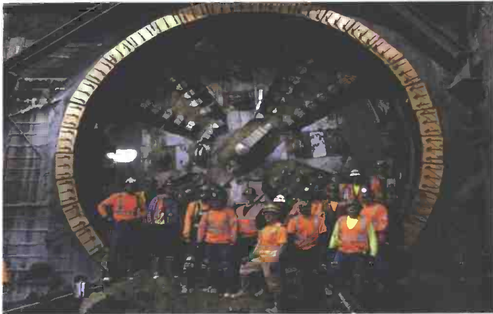
Tunnel boring machine hole thru at Leimert Park Station.
