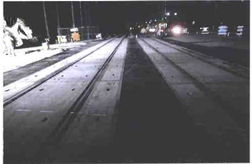
Completed first grade crossing at Centinela Avenue.
