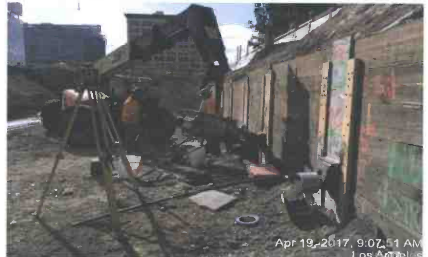
Tie-back installation in Broadway Station
