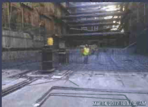
Regional Connector Transit Corridor Project
