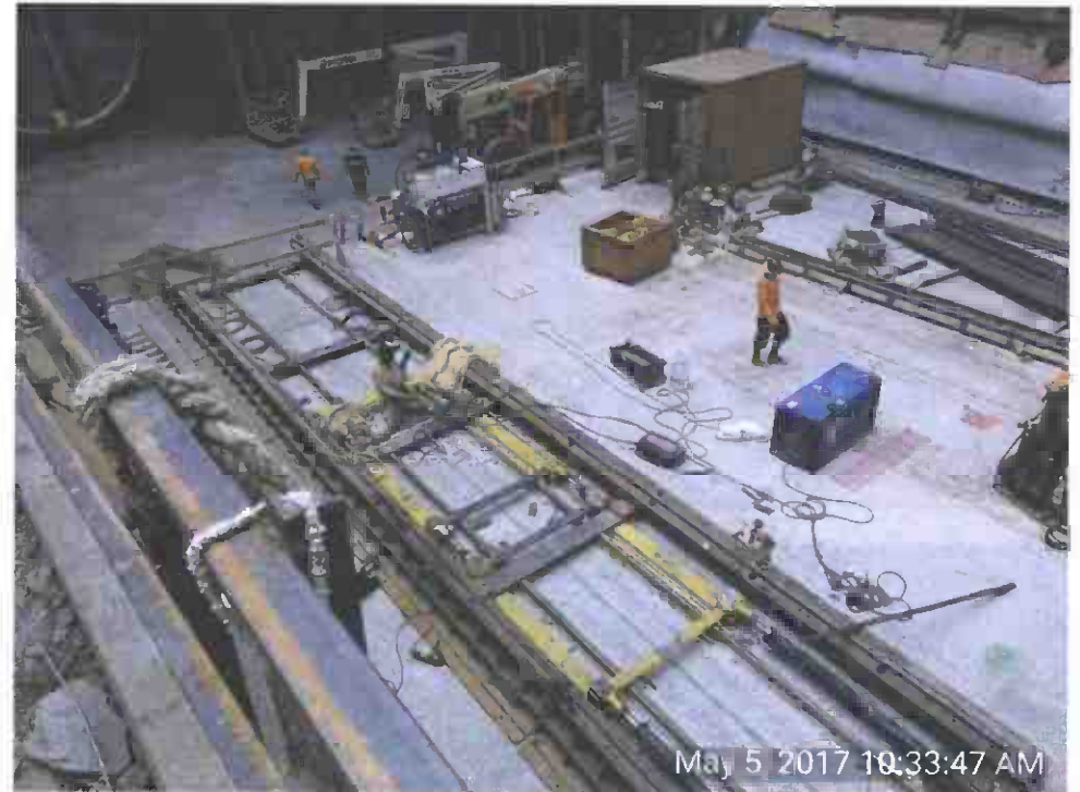
Installing/Staging Reception Cradles (walking frame)
