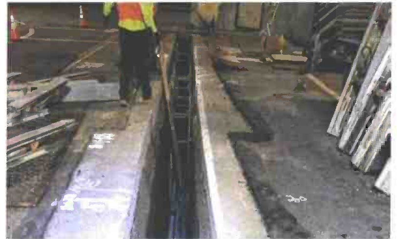
Joint Trench Construction at Constellation Blvd / Avenue of the Stars
