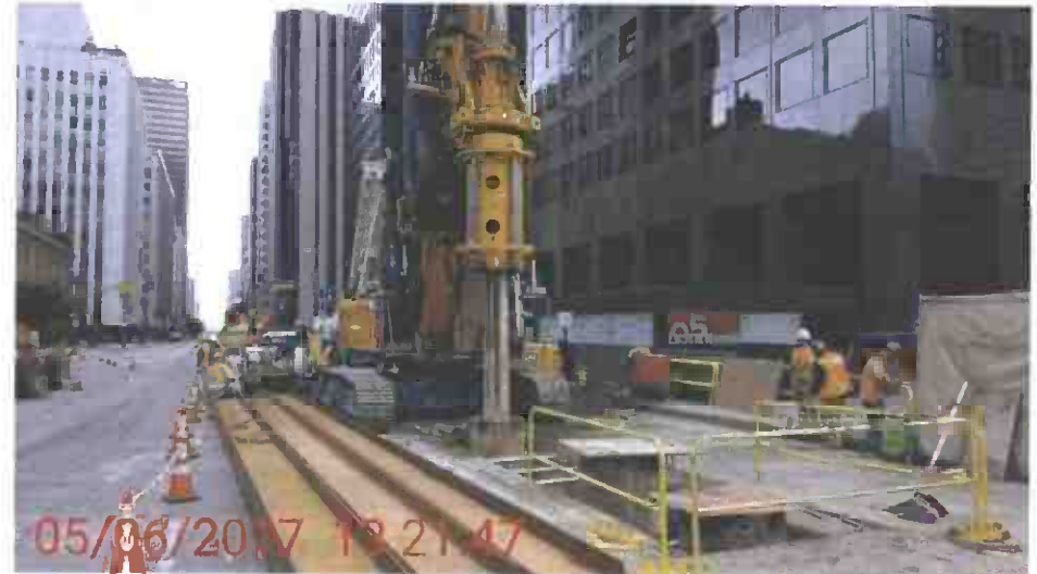
Pile installation at 5 th /Flower
