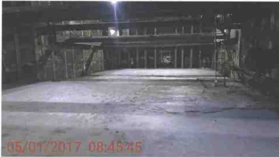
Finished Sub-Invert slab at TBM Retrieval Shaft
