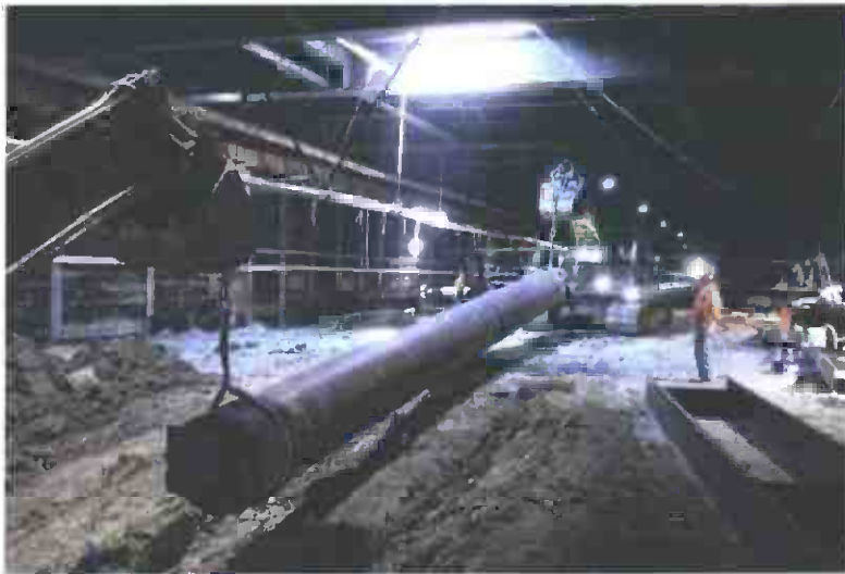
Installing Strut at Wilshire/La Brea Station
