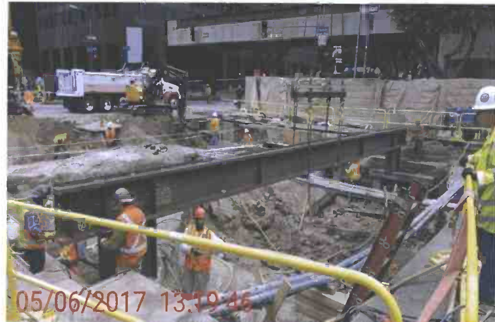
Deck beam Installation at 5th and Flower
