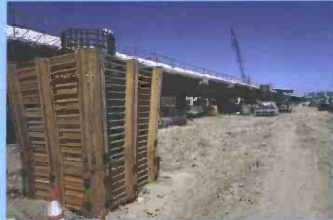
Bent 2 forming with Bents 3 and 4 in the background
