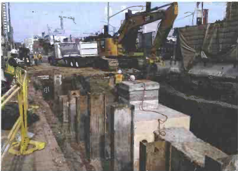
Decking Operation at Wilshire/Fairfax Station
