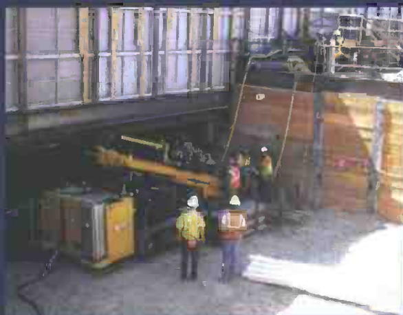
Westside Purple Line Extension Section 1 Project
