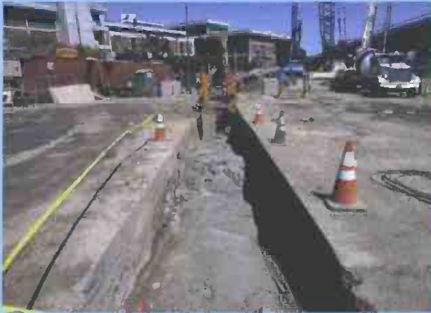
Sanitary sewer relocation along Vignes
