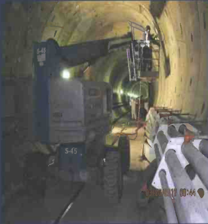
Crenshaw/LAX Transit Project
