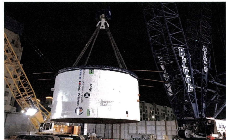
Delivery of TBM Shield to Wilshire/La Brea Station
