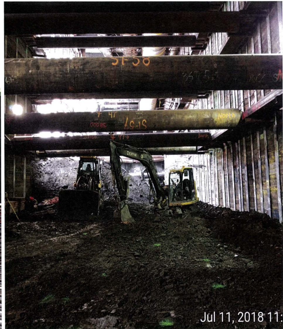
Excavation in center station box
