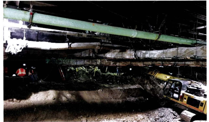
Wilshire/La Cienega Station Excavation
