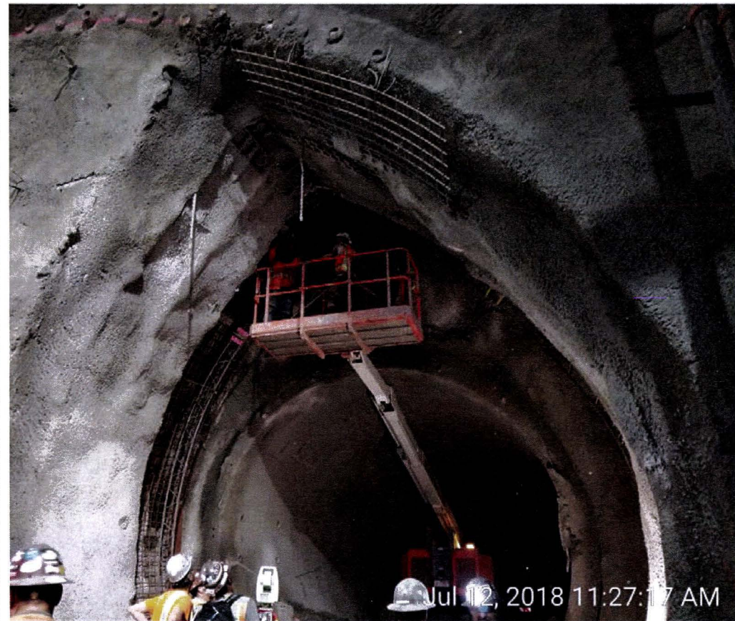
Installation of top head girder, right drift
