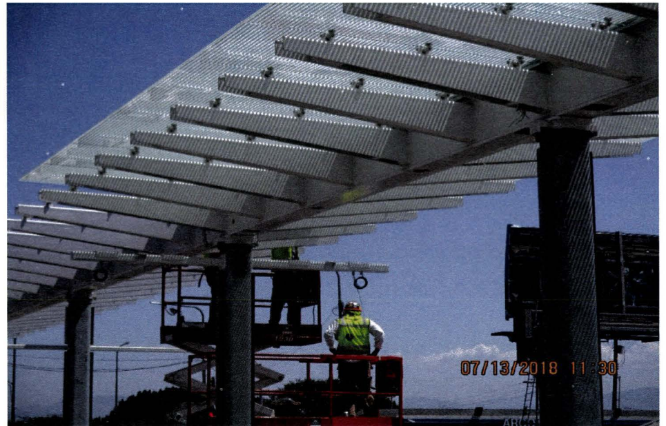
HYDE PARK STATION – Installation of glass canopy.
