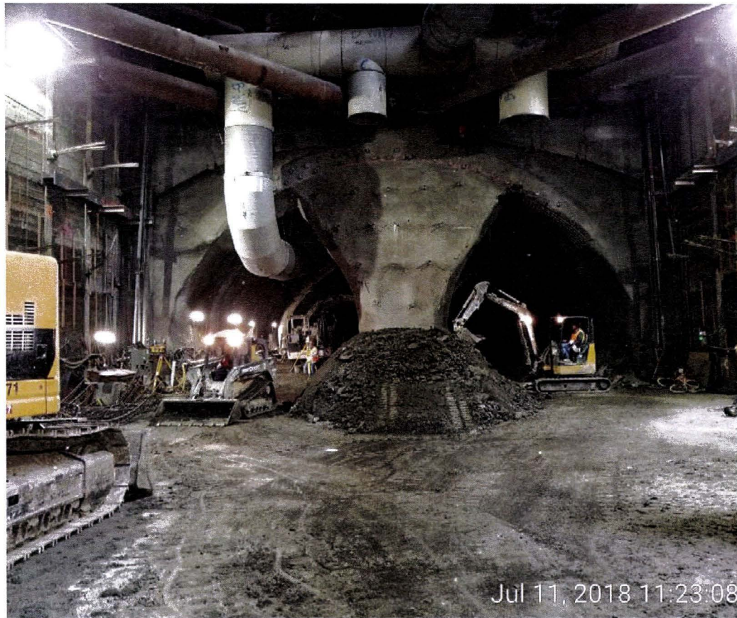
Placing shotcrete, left drift / Excavation of invert, right drift
