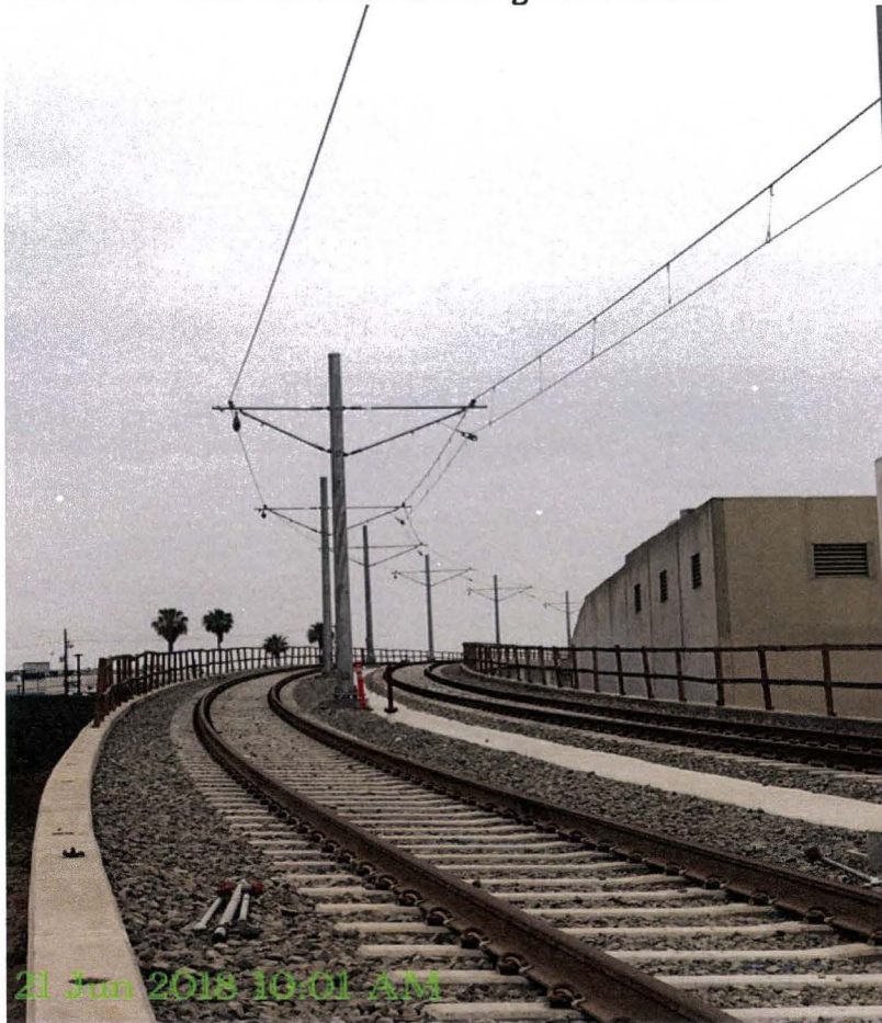
MSE 111 – Crew continue installing contact wire.
