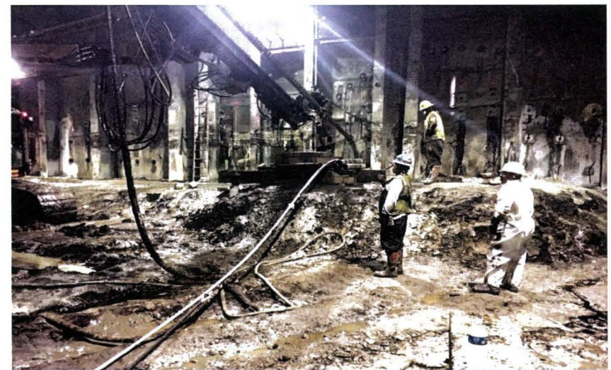
Wilshire/Fairfax Station at Canopy Pipe
