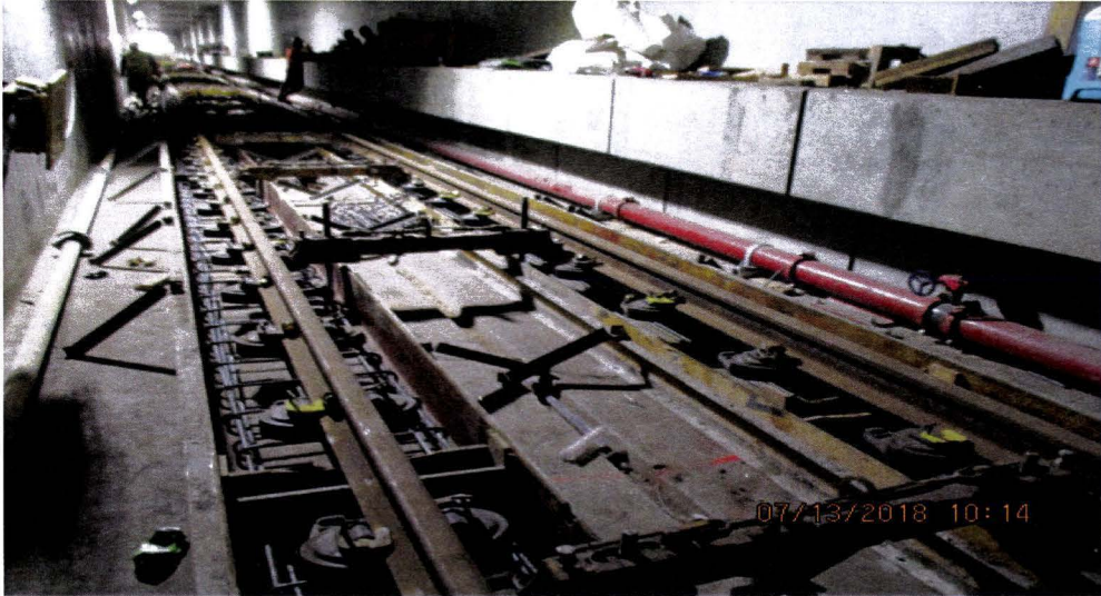
UG#3 – Installation of plinth rebar in the Southbound tunnel.
