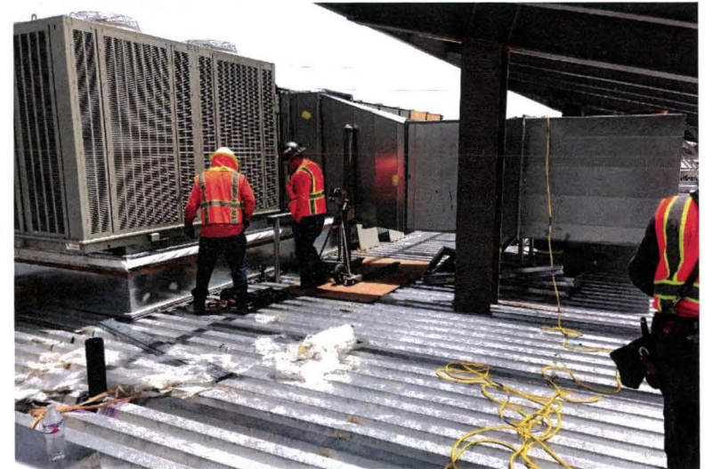
Division 20 Building – HVAC work on the Upper Roof
