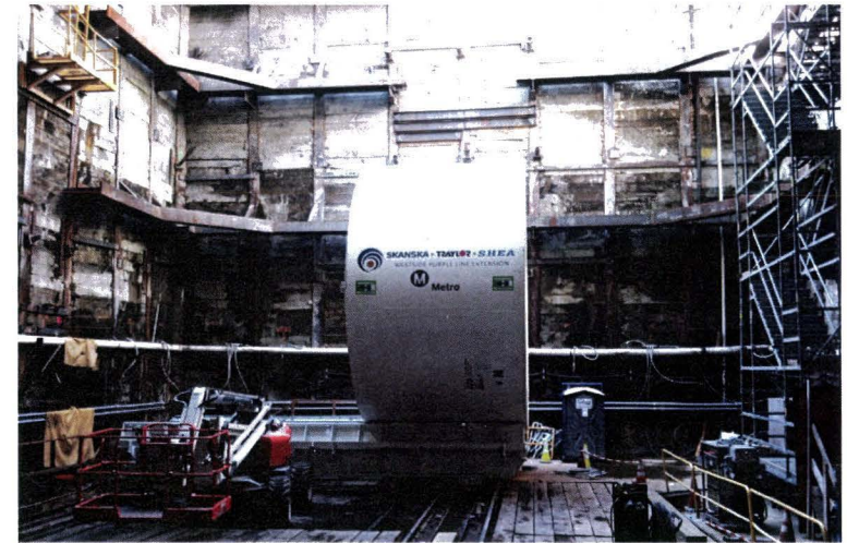
TBM Assembly at Wilshire/La Brea Station
