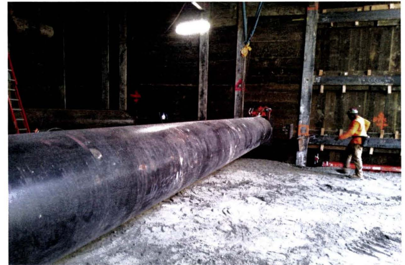
Level B Strut Installation at Wilshire/Western
