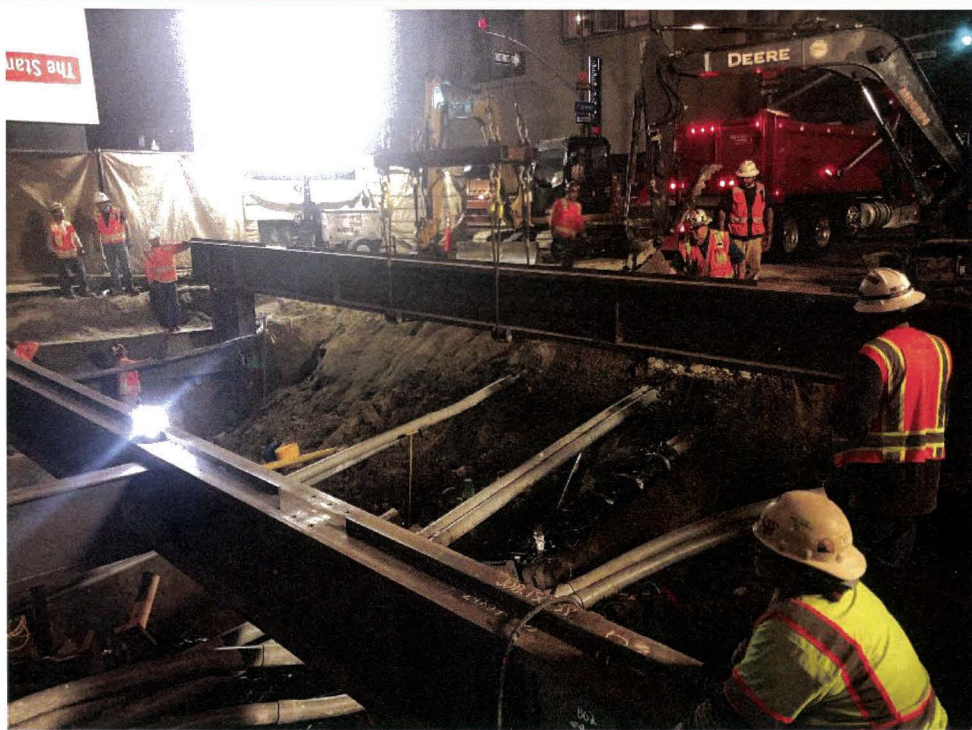
Decking installation at 6th/Flower
