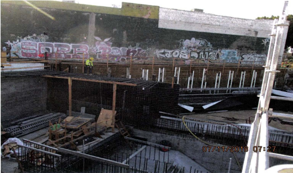
LEIMERT PARK STATION – Installing rebar at the entrance structure.
