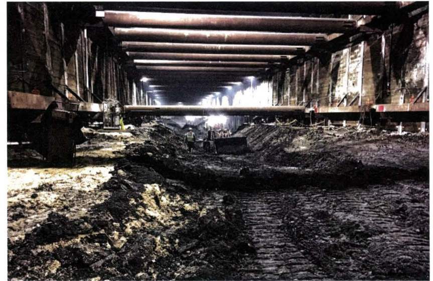
Wilshire/Fairfax Station Excavation
