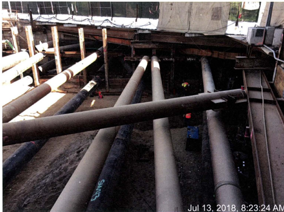
Bracing installation at Central
