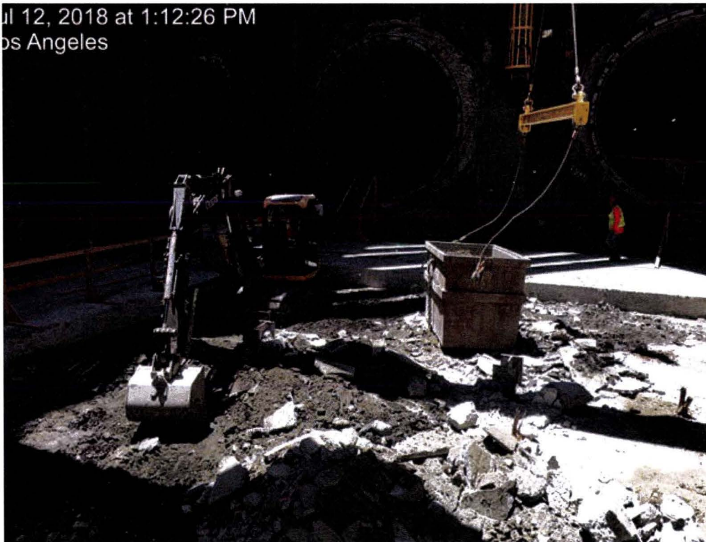
Excavation of west hammerhead deep sump
