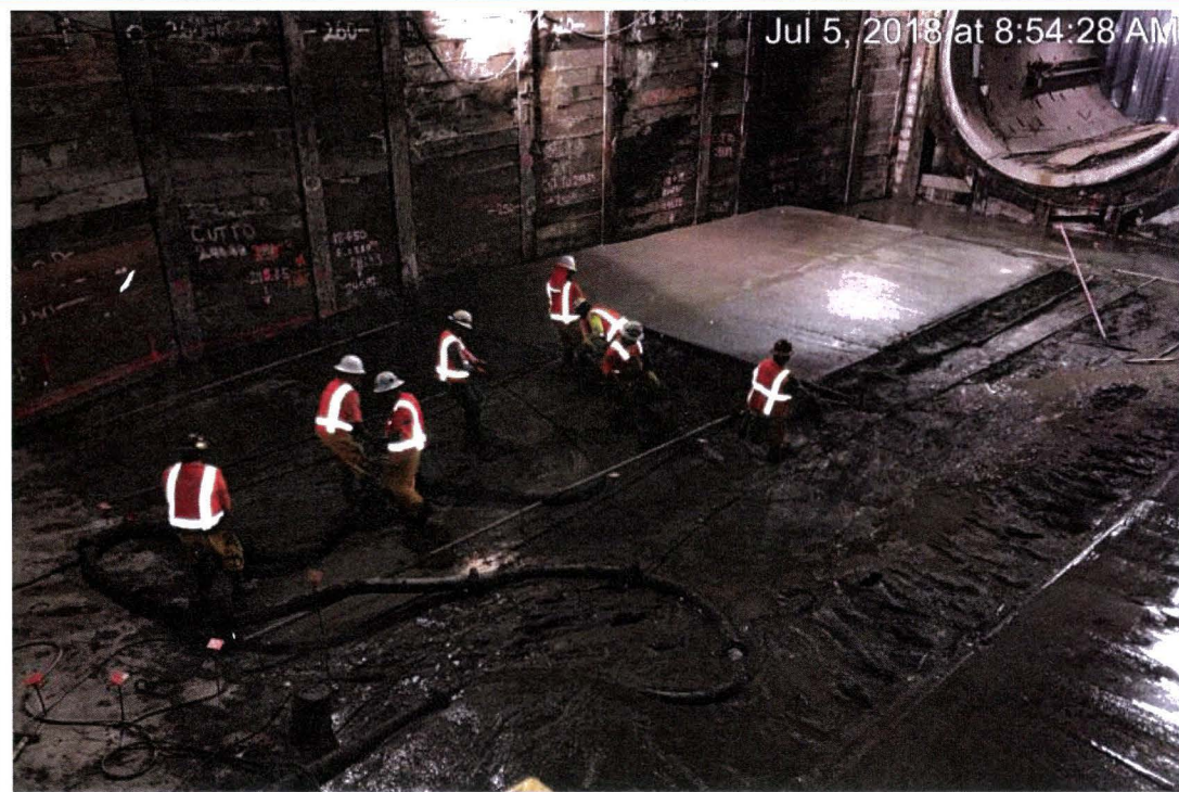
Pouring mud slab in TBM Retrieval Shaft
