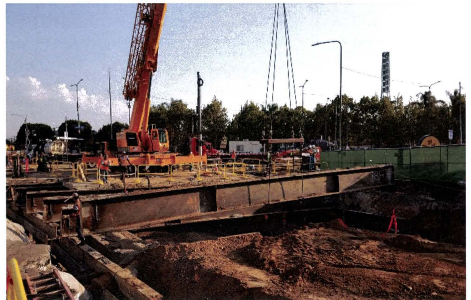
LEIMERT PARK STATION – Deck beam removal (restoration work) during 43-day closure.
