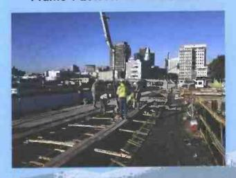
Pouring Stems and Soffit Frame 2 Left
