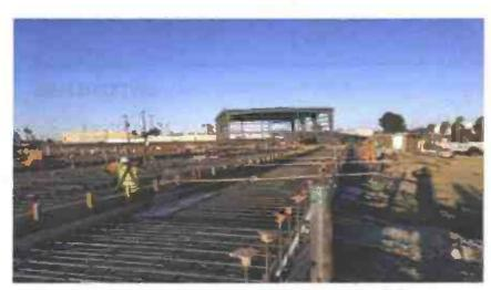
Placing reinforcement for car wash slab
