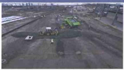
**Dumping ballast at underdrains**
