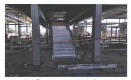
Installing stairs to service platform
