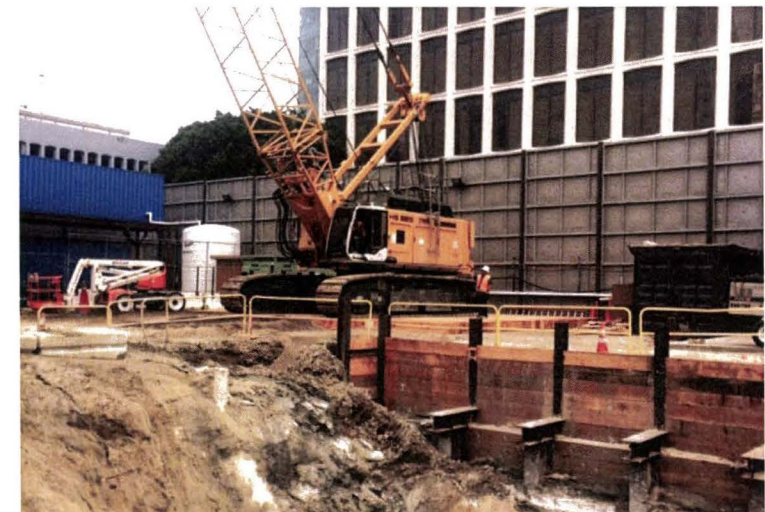
Wilshire/Western Site Crane Mobilized
