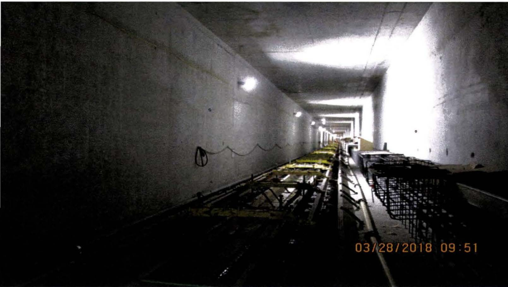
UG#3 – Ironhorse direct fixation plinth construction alongside walkway reinforcement
