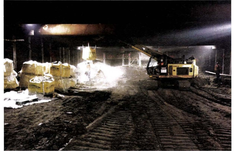
Shotcrete Placement at Wilshire/Fairfax Station
