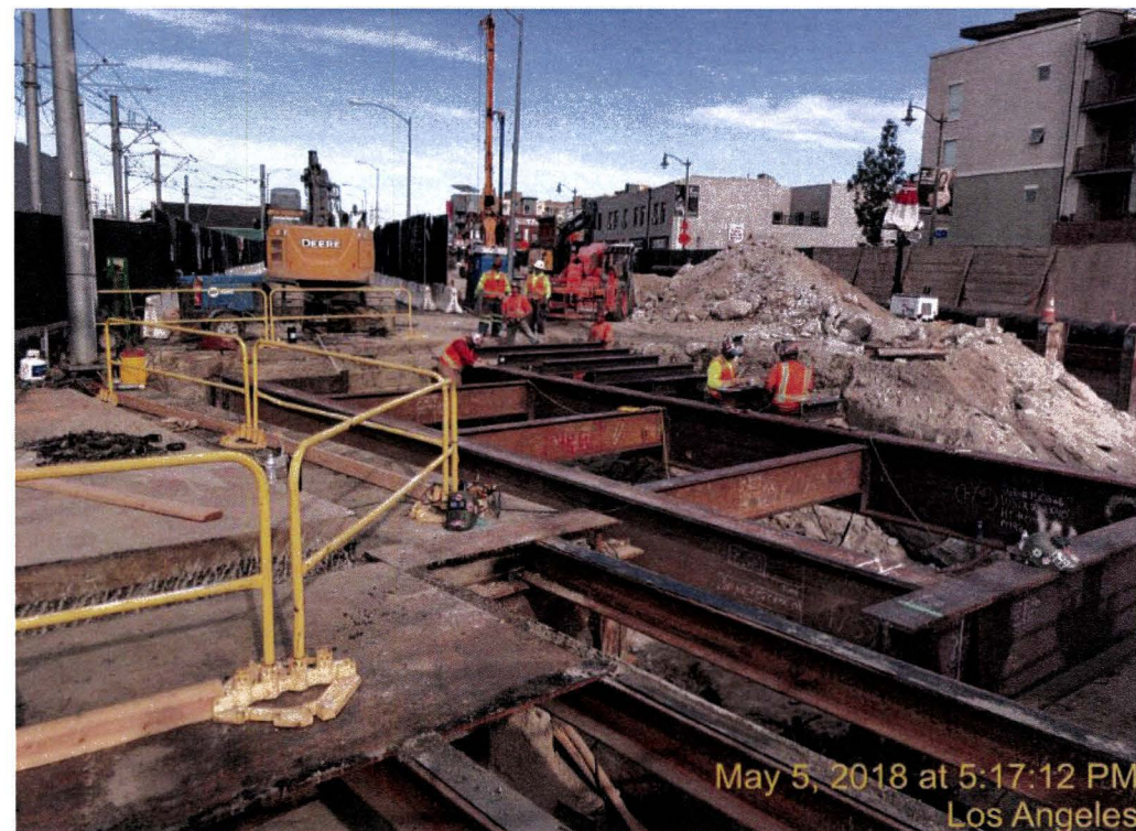
Decking work near 1st/Alameda intersection
