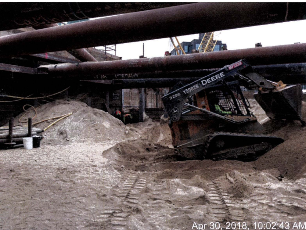
Excavation and lagging at Central SOE
