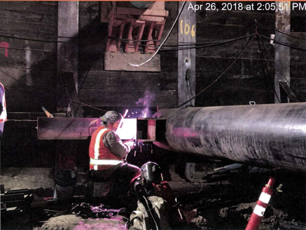
Installing middle level strut
