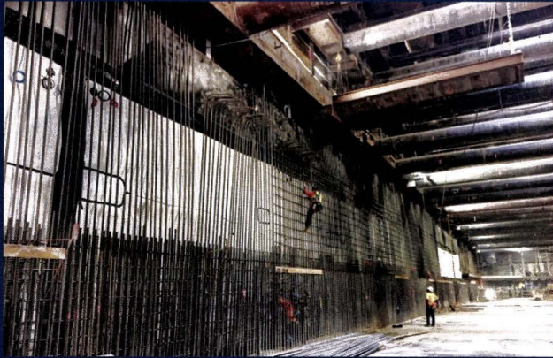
Westside Purple Line Extension Section 1 Project
