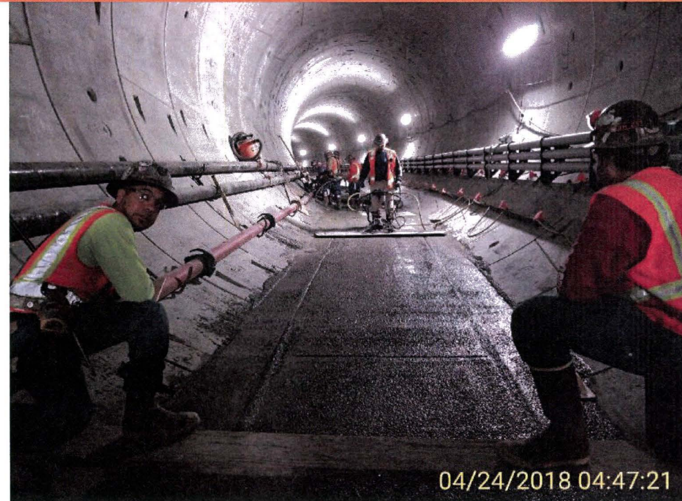
Tunnel crews beginning pour for right tunnel, Hope to Flower
