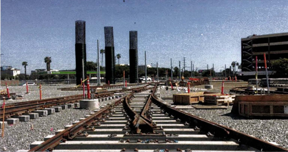
Southwestern Yard – Looking south showing yard and automated people mover columns
