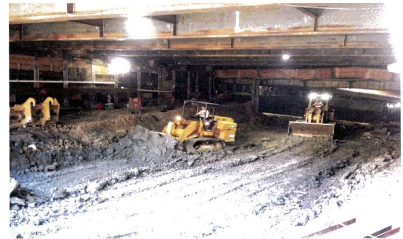
Wilshire/La Cienega Station Level A Excavation
