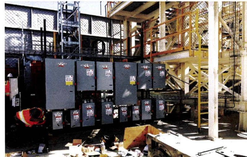
Conveyor Tower Belt Assembly at Wilshire/La Brea Station 9
