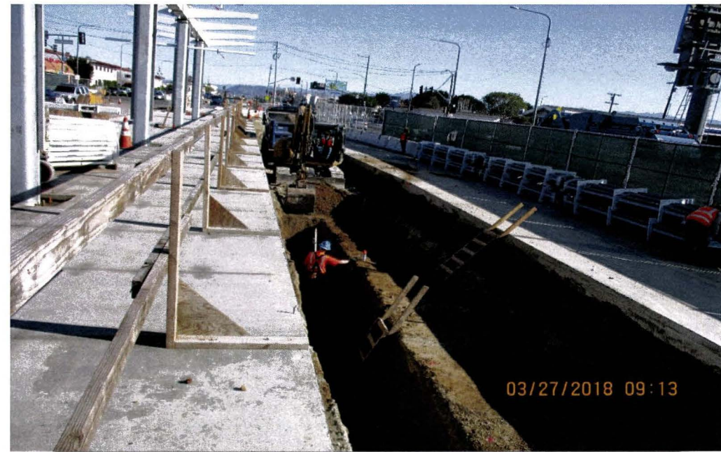
Hyde Park Station – Trenching for systems duct bank
