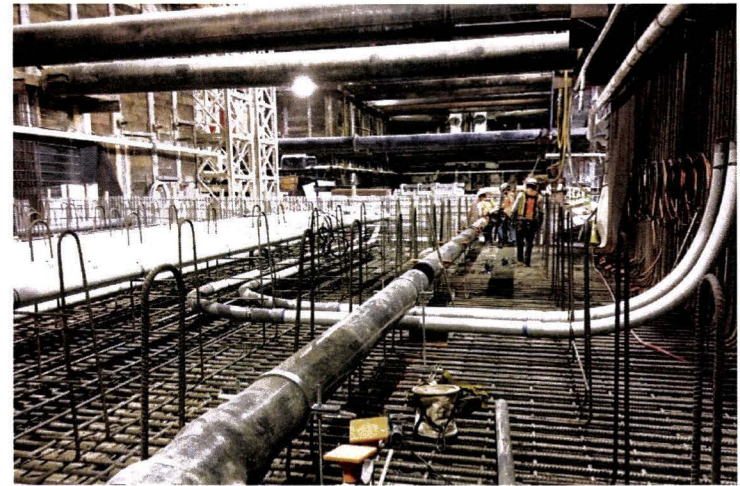
Drain installation at Wilshire/La Brea Station
