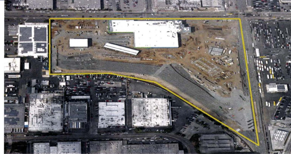
Southwestern Yard – Aerial view as of 04/2018
