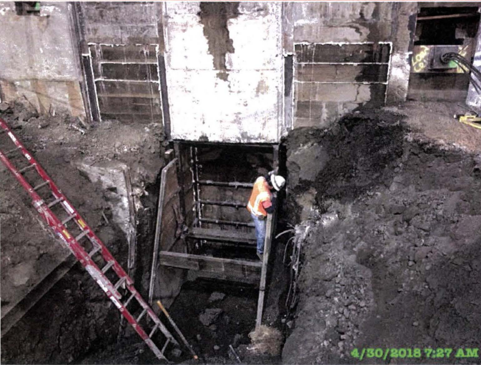
Form underpinning columns at LA Times Building
