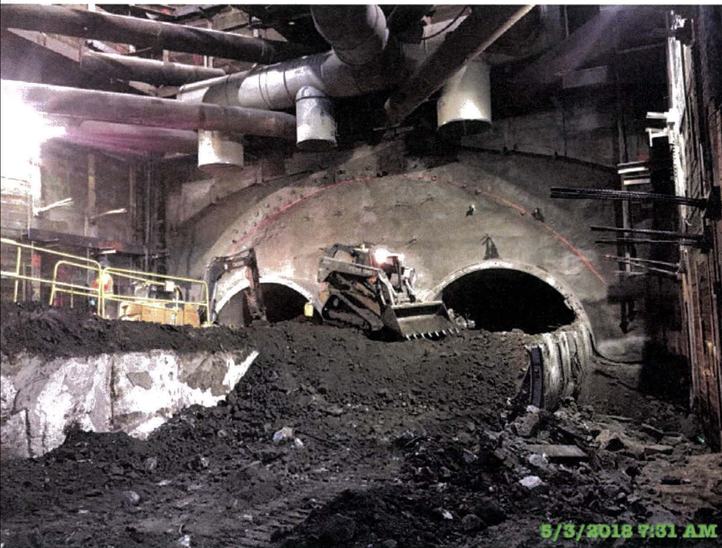
Excavation and breakout of tunnel segments in Spring Street hammerhead
