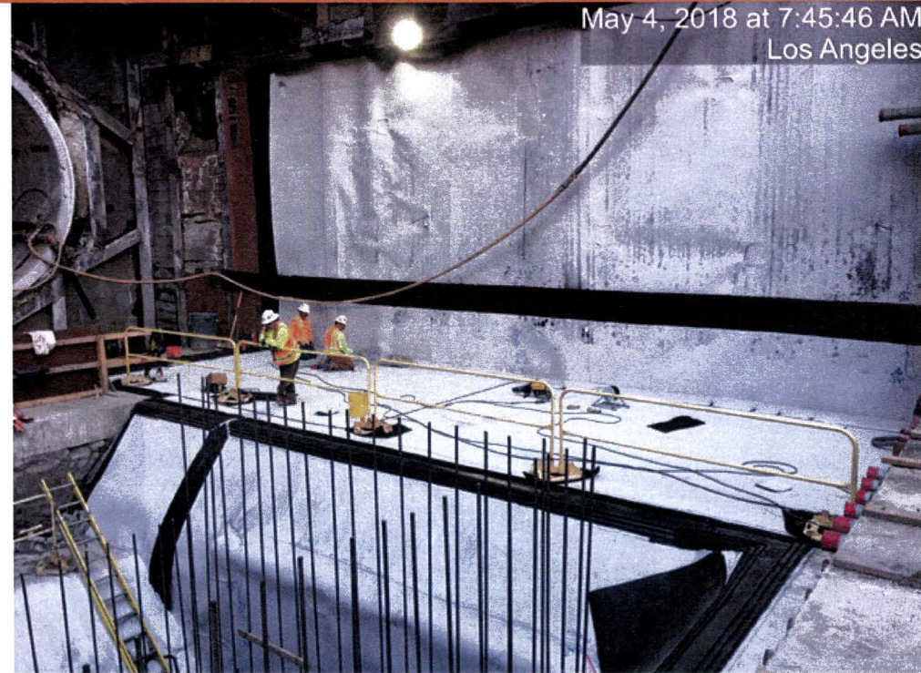
HDPE East Hammerhead
