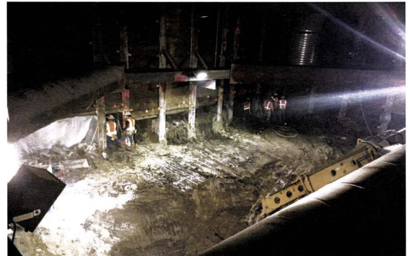
Excavation at West End of Wilshire/Fairfax Station
