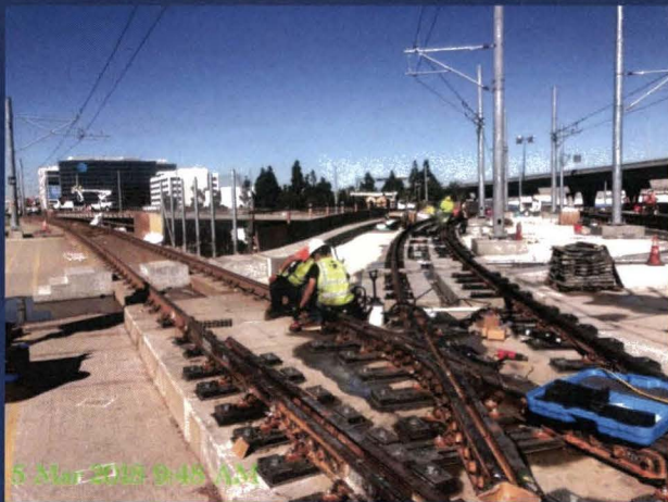
Crenshaw/LAX Transit Project
