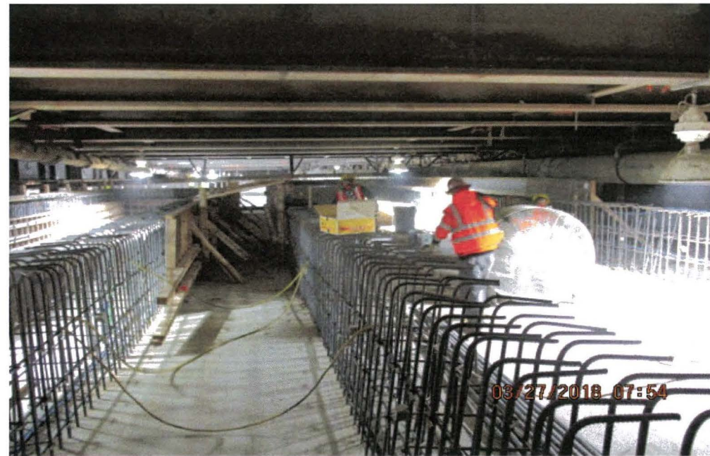
Leimert Park Station – Installation of formwork for roof plenum walls.
