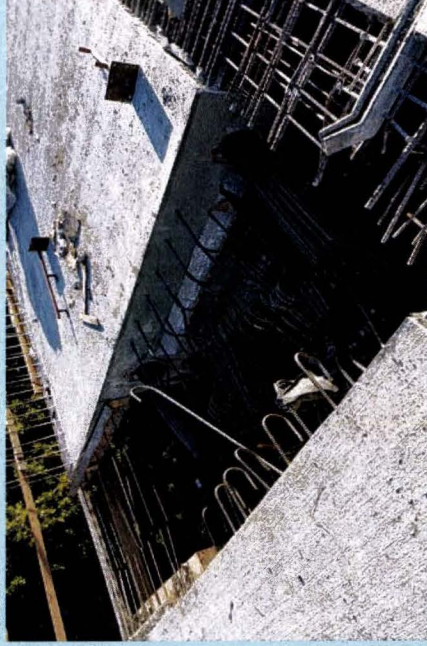
Frame 4 Left Post Tensioning
