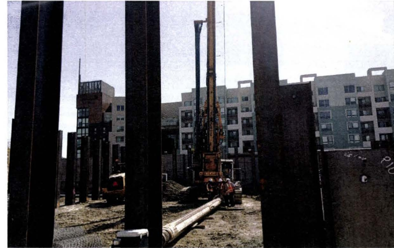
Muck Bin Pile Installation at Wilshire/La Brea Station
