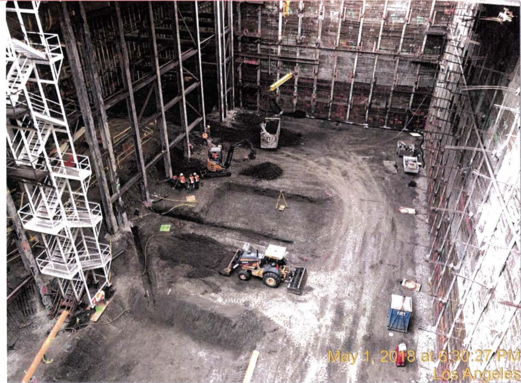
Fine grading ancillary station structure
