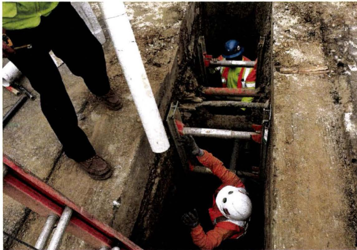
SCG utility work
