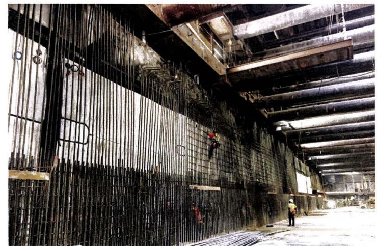
Wall Rebar Installation at Wilshire/La Brea Station 5
