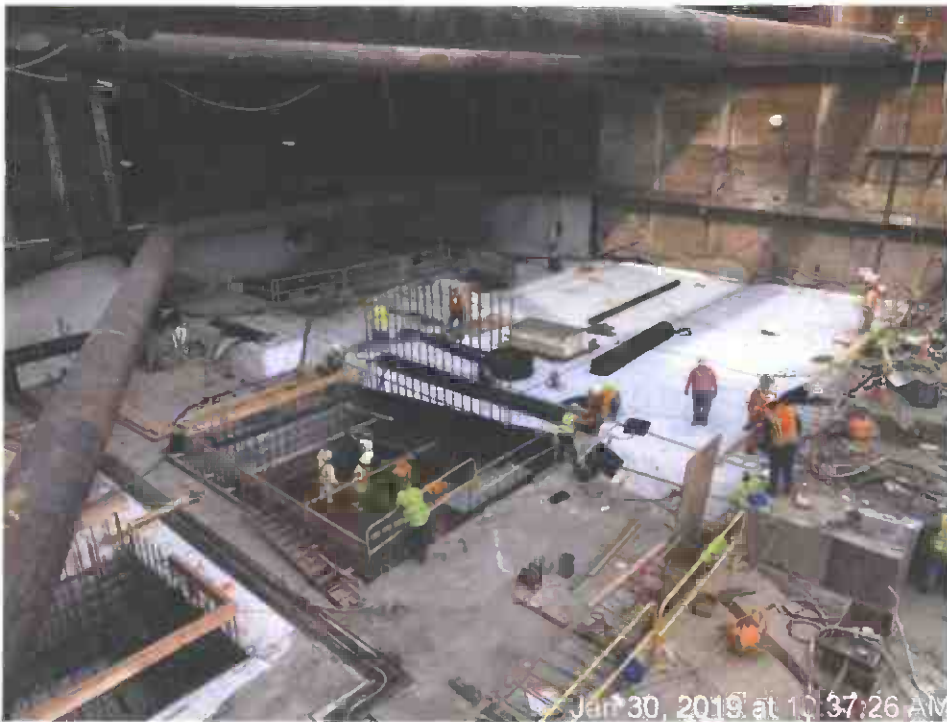
Sump/Ejector pit invert placement HDPE
