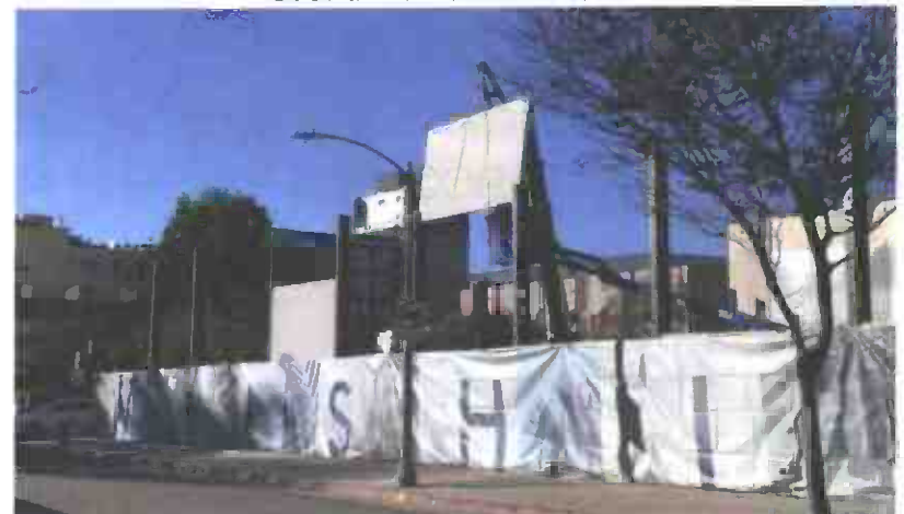
Sound Wall Installation
