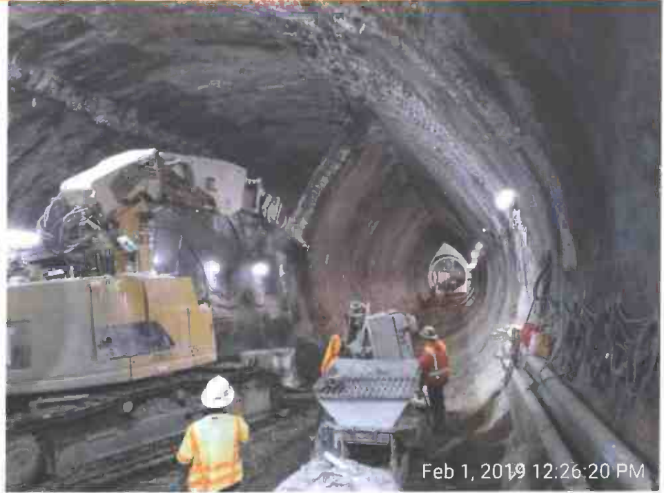
Right center wall demolition
