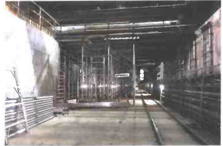
Concourse Deck Shoring
