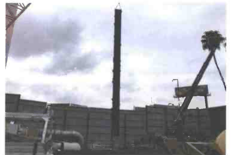
Lifting Waler out of the Western Shaft
