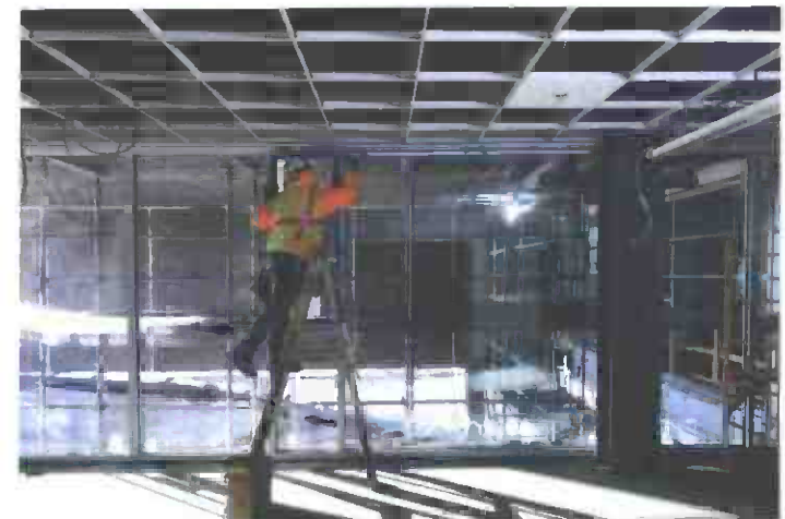
Division 20 MOW Building – Glazing Installation
