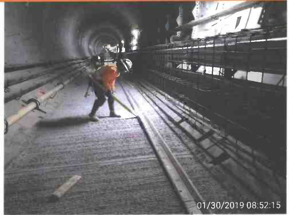
Setting walkway form rails and guides in tunnels, Reach 2
