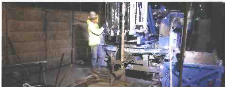
Seismic Borings
