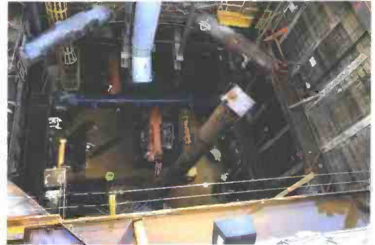
Lifting Strut out of the Western Shaft
