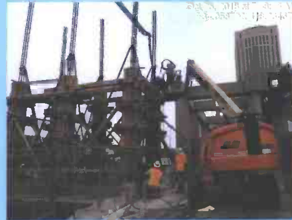
Pouring Plaza level elevator enclosure columns
