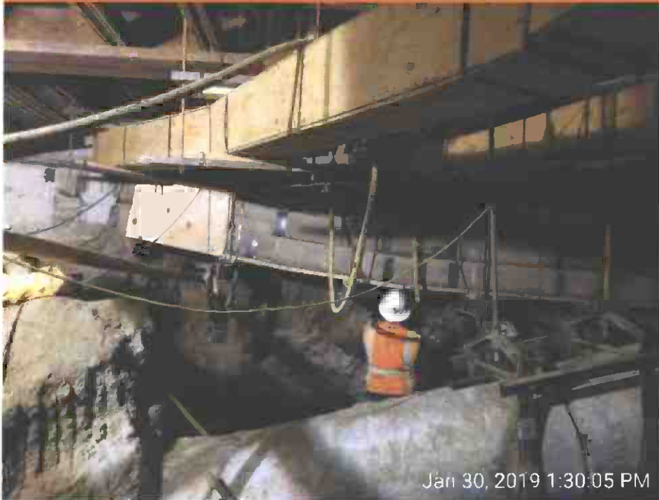
Support of communication duct banks near 6th/Flower
