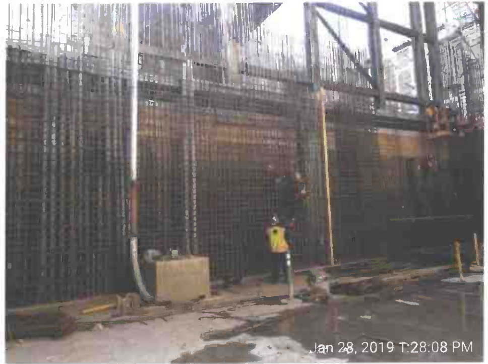
Front face rebar installation at Wall D
