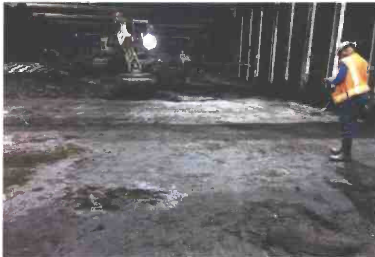
Fairfax Station Fine Grading
