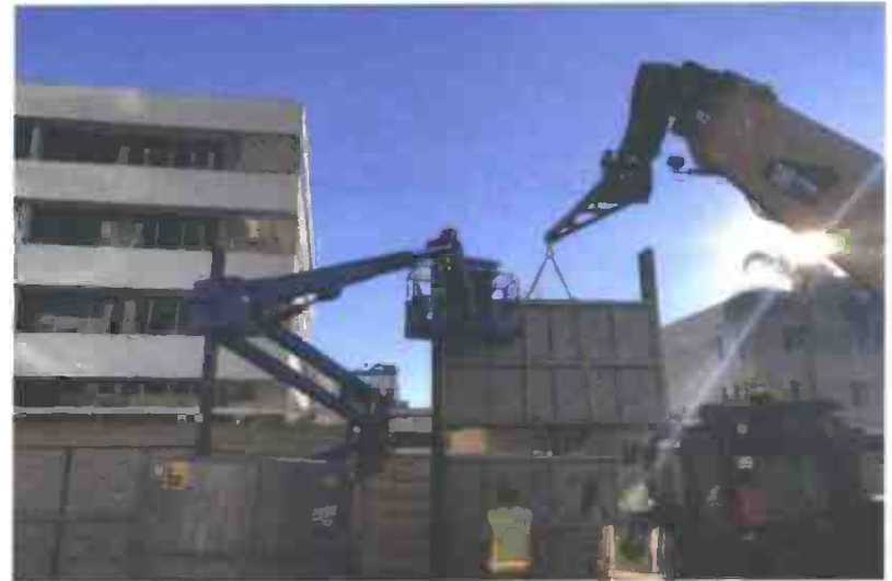
Sound Wall Installation
