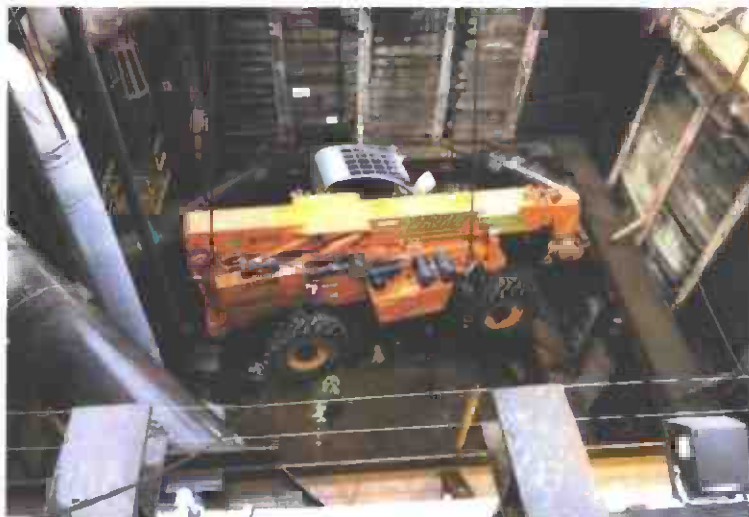
Lifting Forklift out of the Western Shaft
