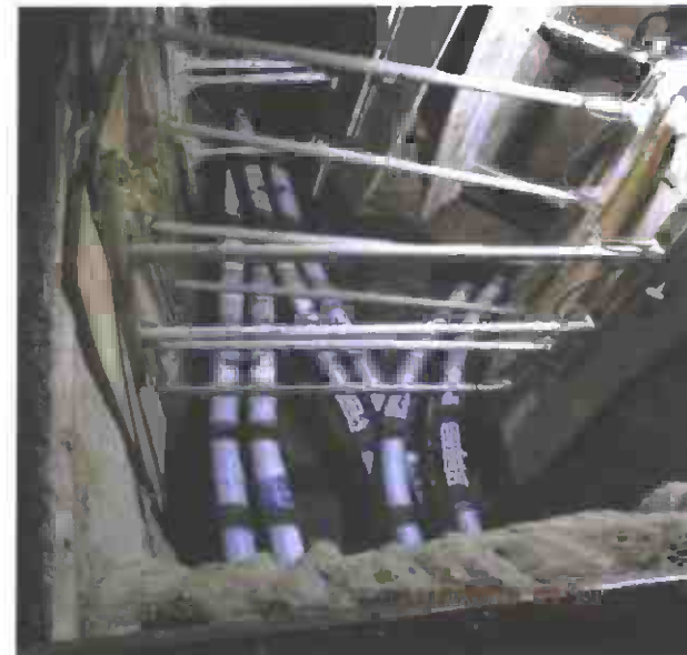
Conduit Installation on Wilshire Blvd.
