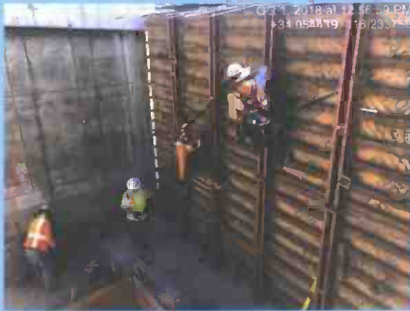
Setting elevator enclosure forms
