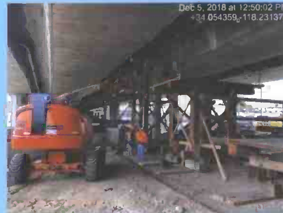
Setting falsework for the emergency stairway exit
