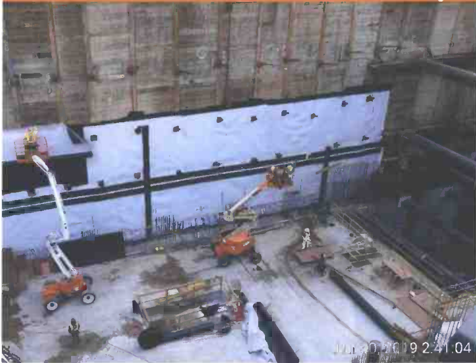
HDPE and water bar installation at south exterior wall
