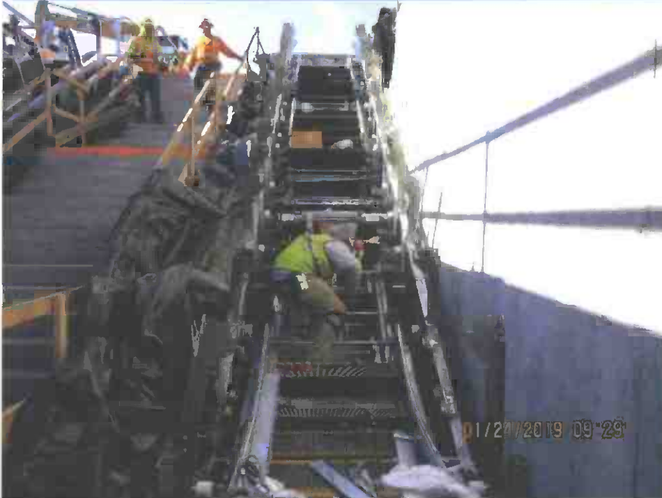
LEIMERT PARK STATION – Installation of escalator 1 and 2 at the entrance
