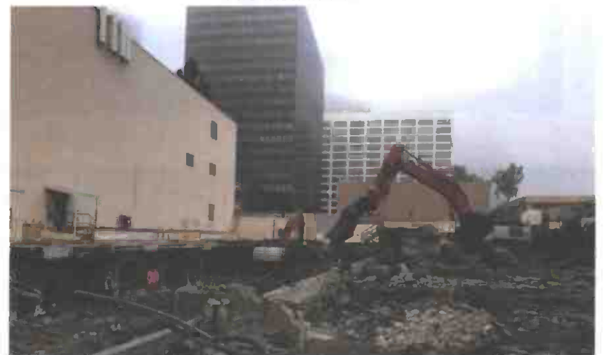
AT&T Parking Lot Demolition
