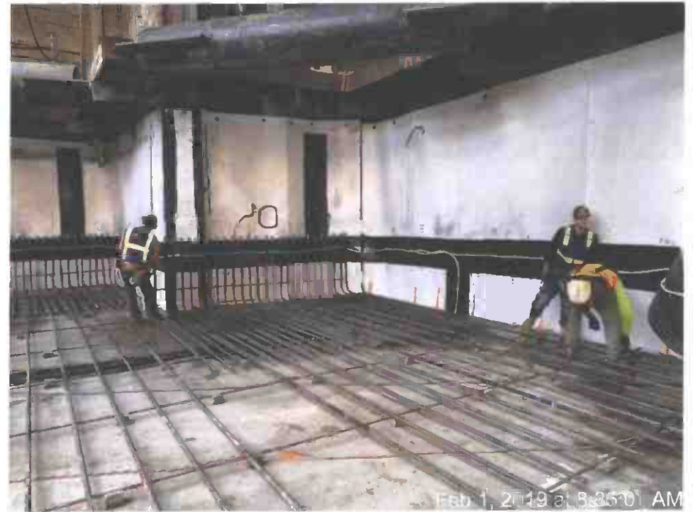
Bottom mat rebar installation at west end
