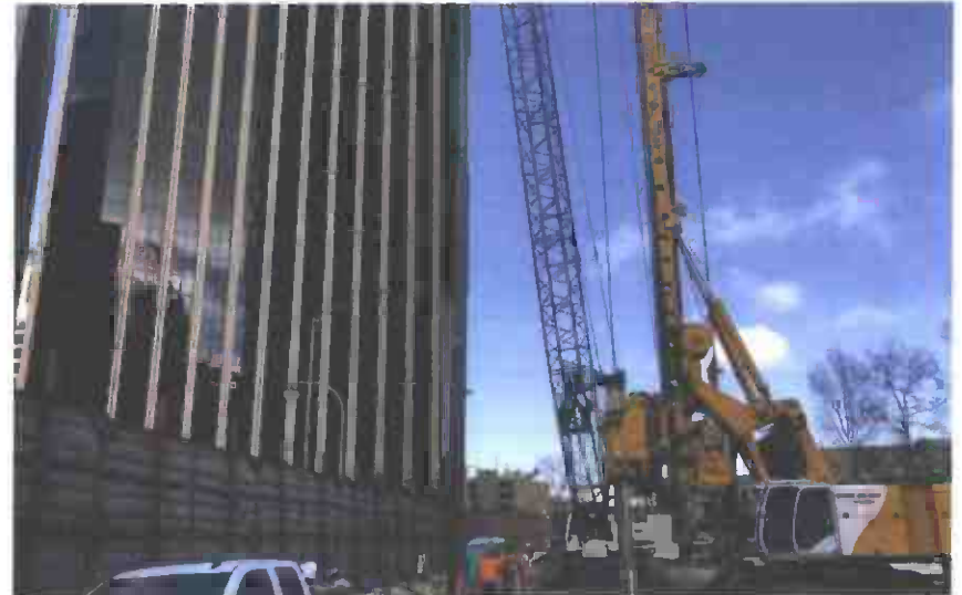
Pile Installation
