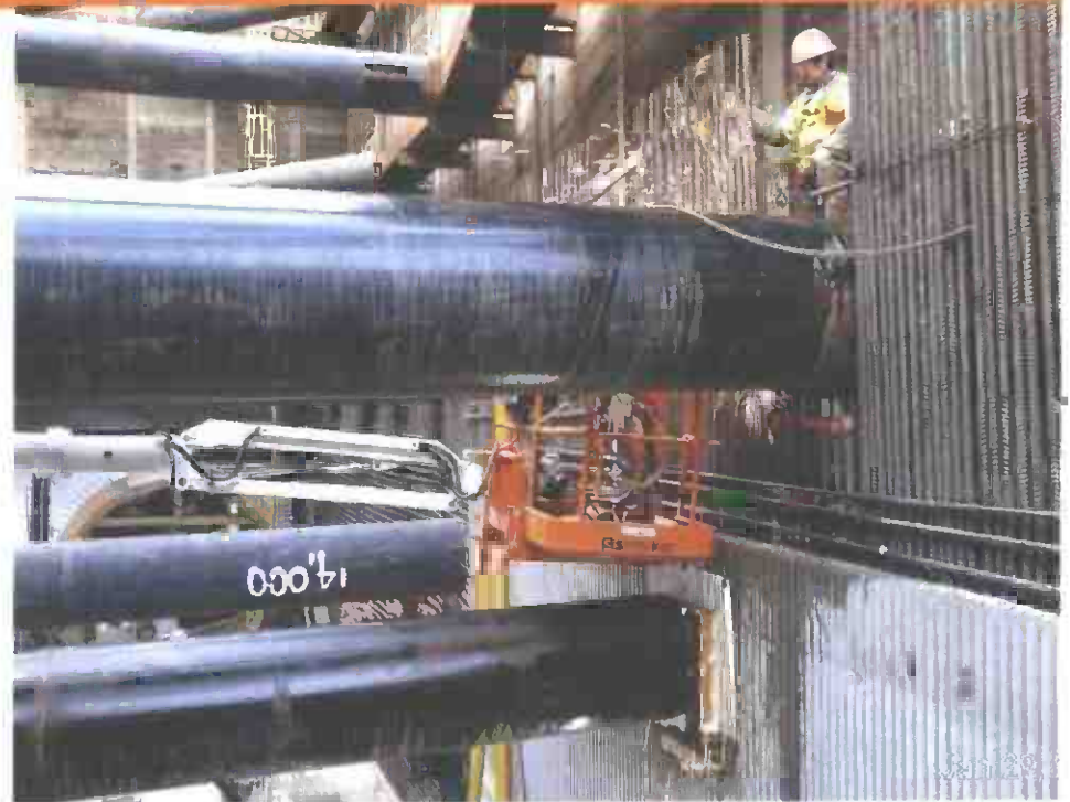
Strut removal at west hammerhead
