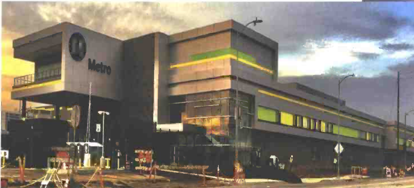
SOUTHWESTERN YARD – Main building
