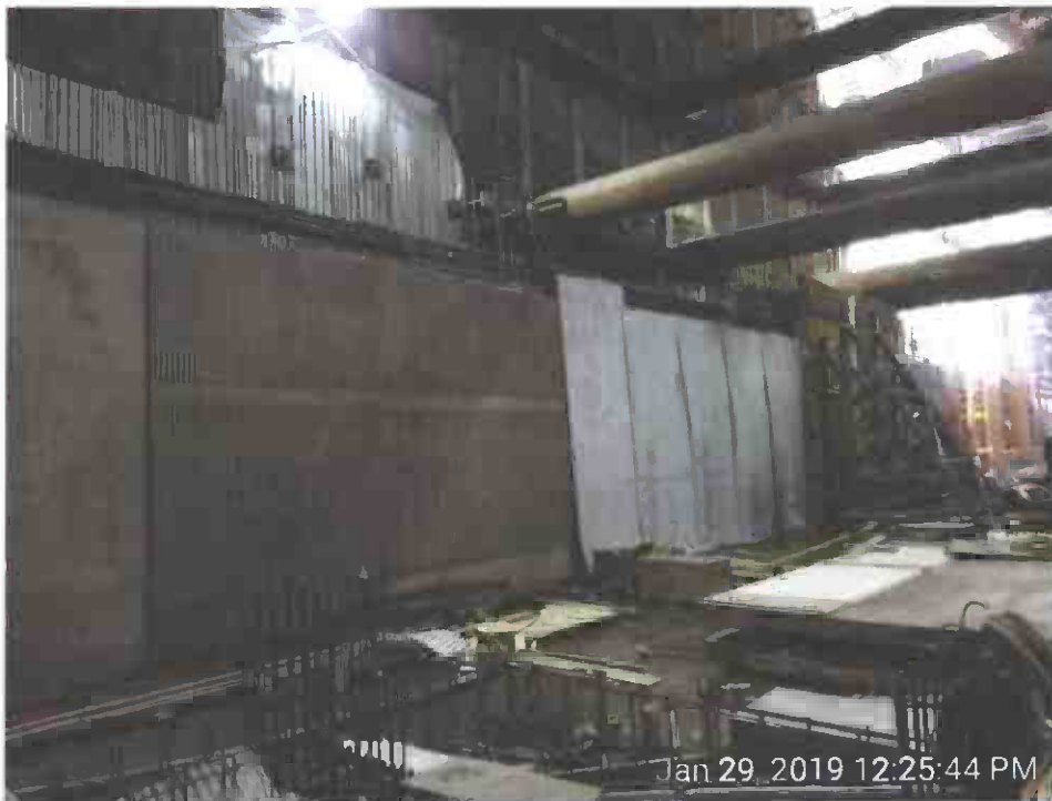
Wall D concrete curing
