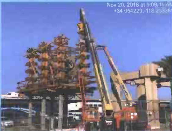
Pouring second level elevator enclosure columns
