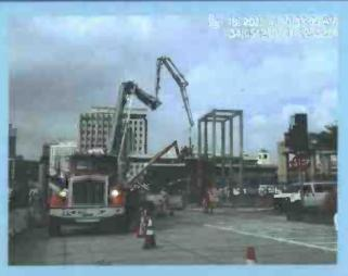
Pouring columns for the elevator structure
