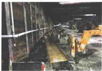
Installing Level D Walers at La Cienega Station
