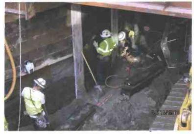
Installation of TBM Launch Box Lagging
