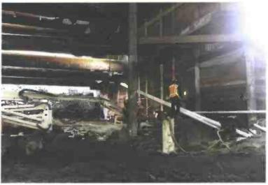
Installed Dewatering System at La Cienega Station
