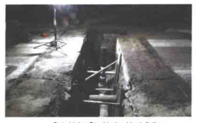
Gate Valve Steel Lateral Installation
