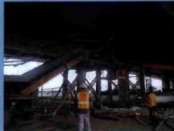
Stripping Forms from the Emergency Stairway Exit
