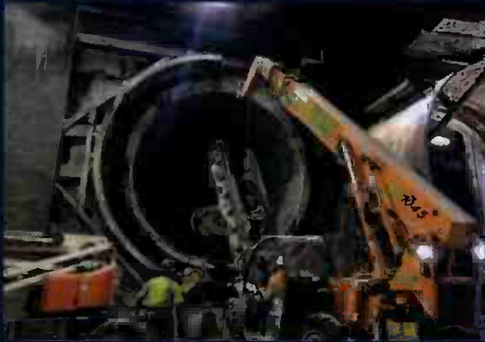
Westside Purple Line Extension Section 1 Project
