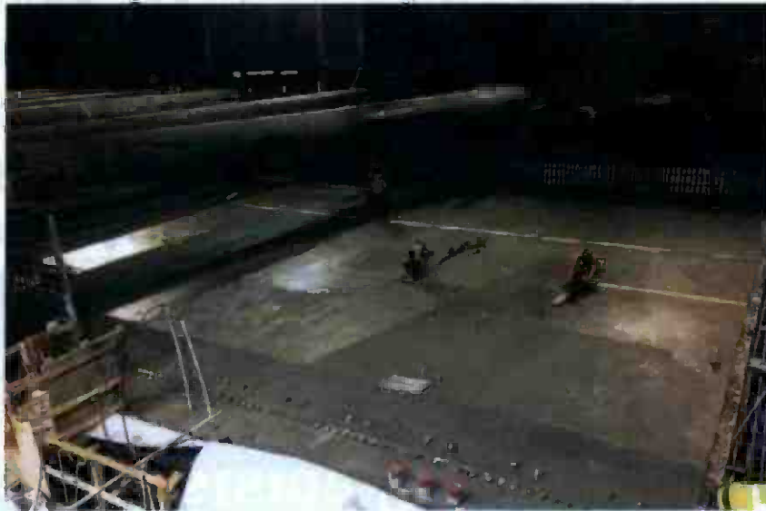
Invert Slab Concrete Placement at Level D, Block 10
