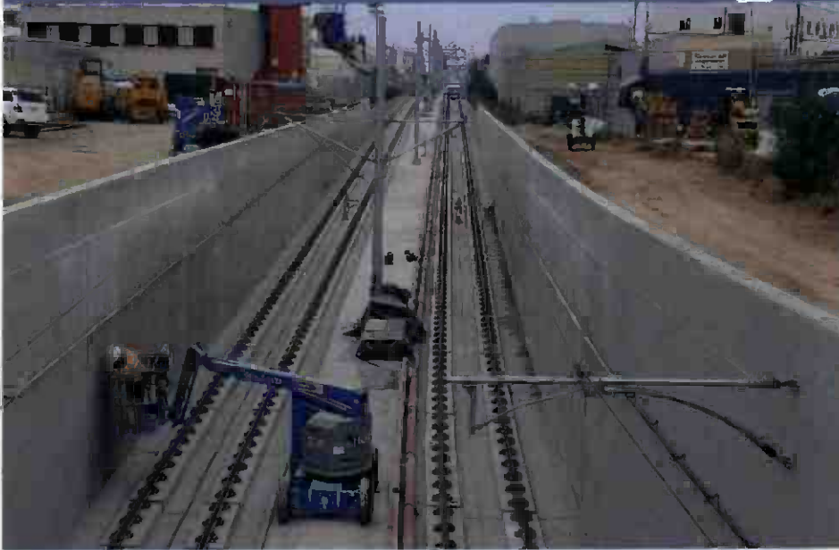
UG3 – Continued finish work on U-channel walls of southbound portal
