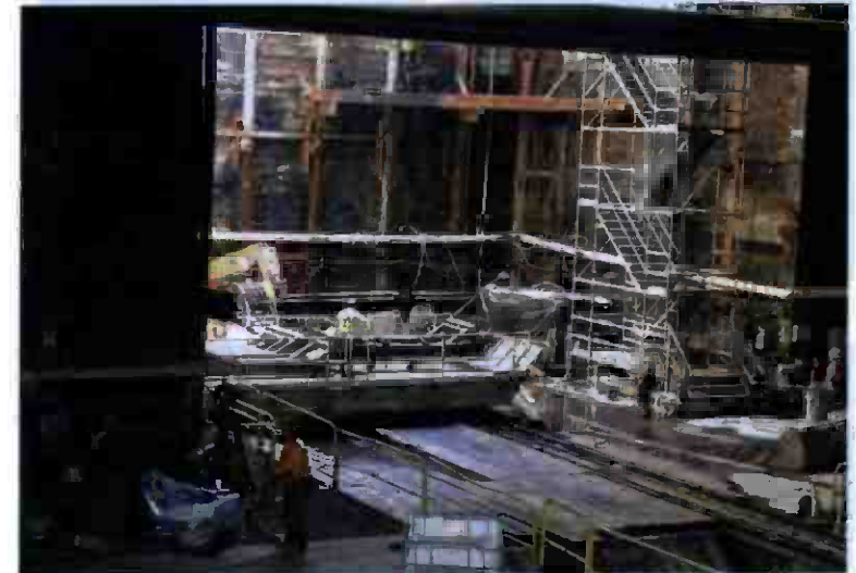
Lowering TBM Cradle
