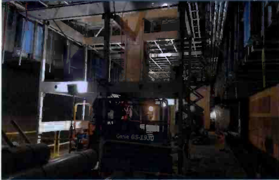
Exposition/Crenshaw Station – Continued installation of elevator frames 3 & 4 at the platform level
