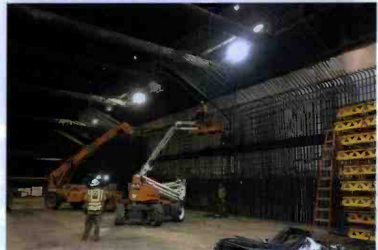
Rebar Installation at Concourse Exterior Walls
