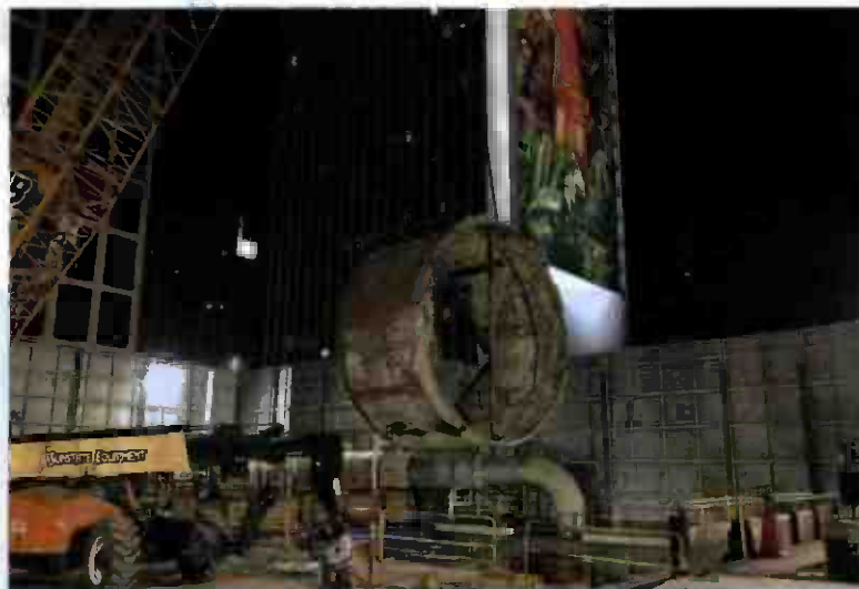
TBM Gantry Shield at Western Shaft
