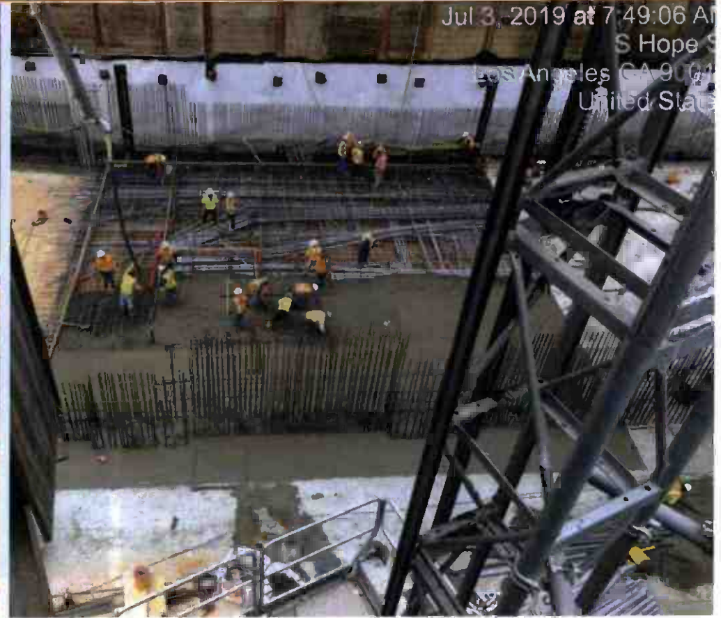
Concrete placement at Ancillary Deck
