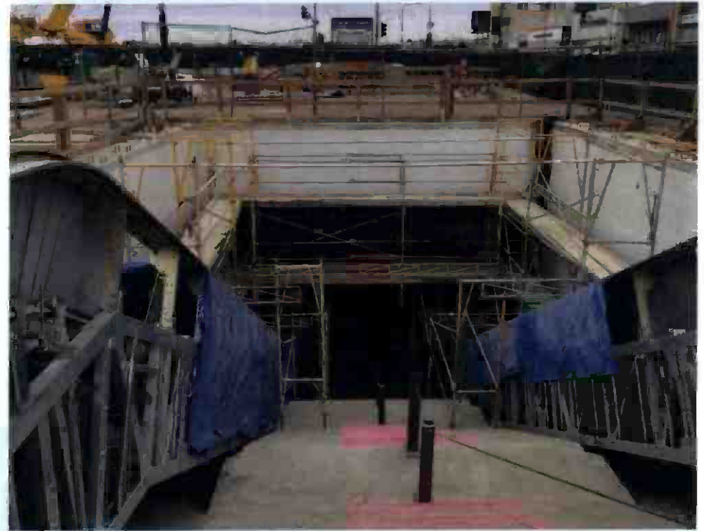
Leimert Park Station – Continued tile installation from mid-landing to plaza
