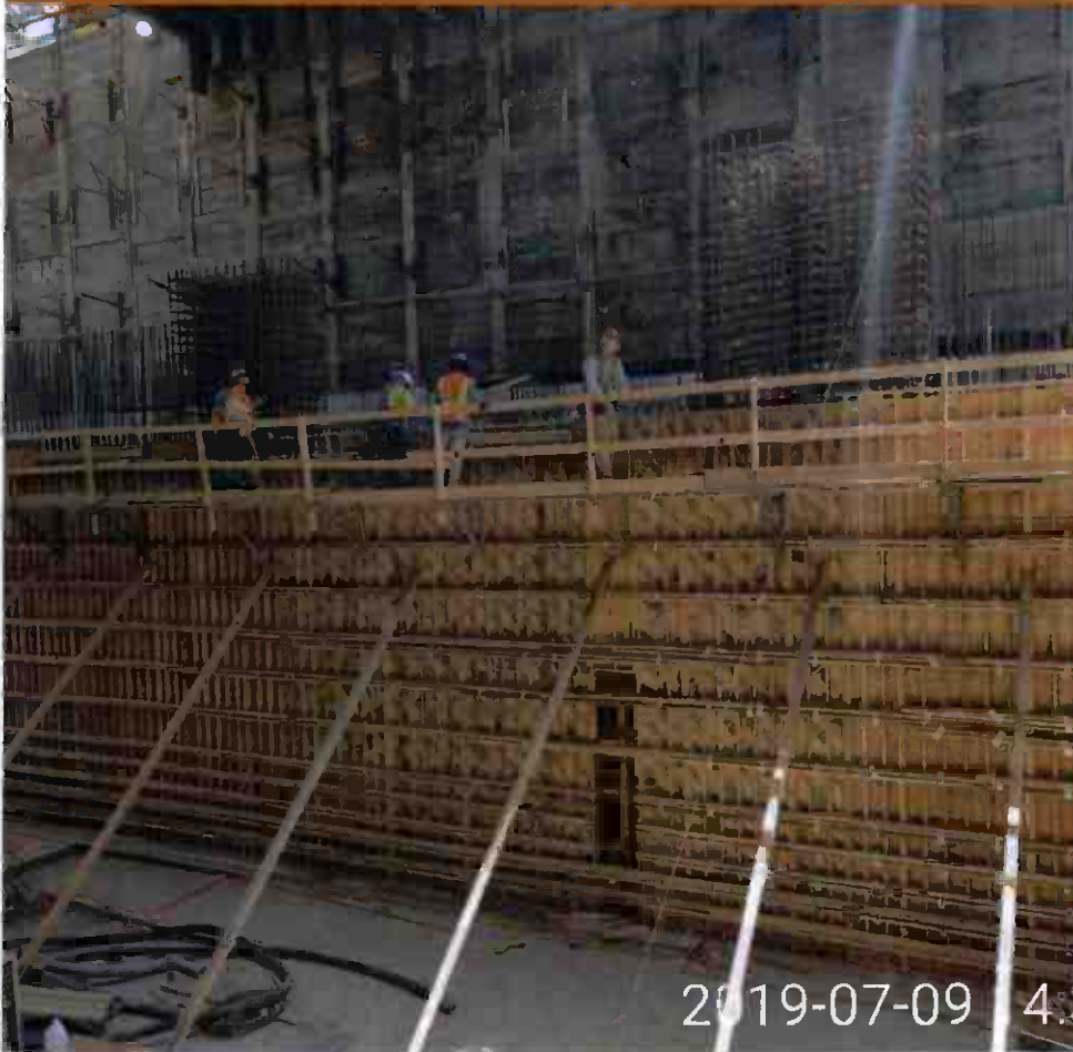
Interior wall formwork at Entrance Structure
