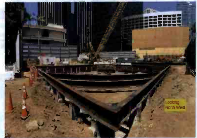
Tunnel Shaft Excavation
