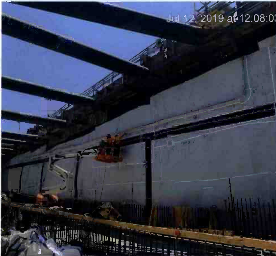
1st Street Cut & Cover HDPE installation
