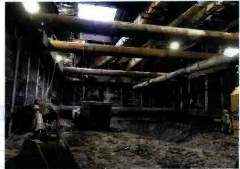
TBM Launch Box Excavation
