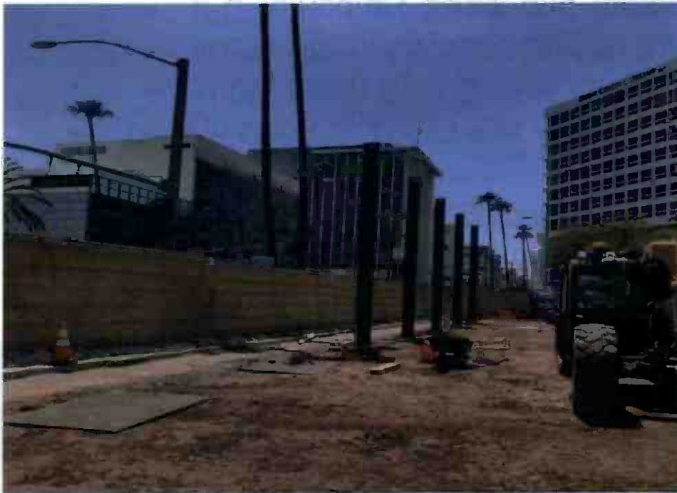
Sound Wall Piles
