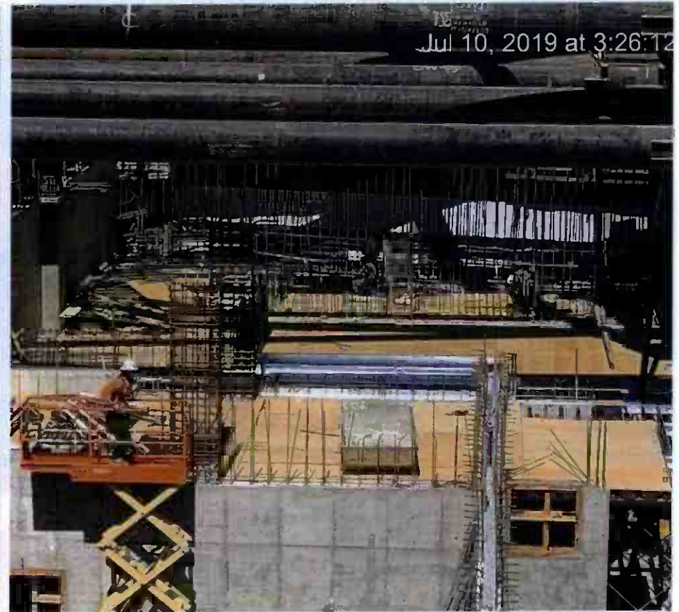
Decking installation at Central Station
