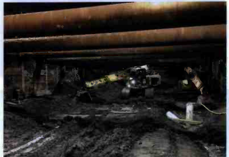
La Cienega Station Facing East
