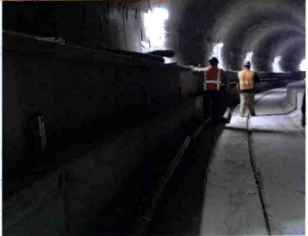
Installing water standpipe in Right Tunnel, Reach 2
