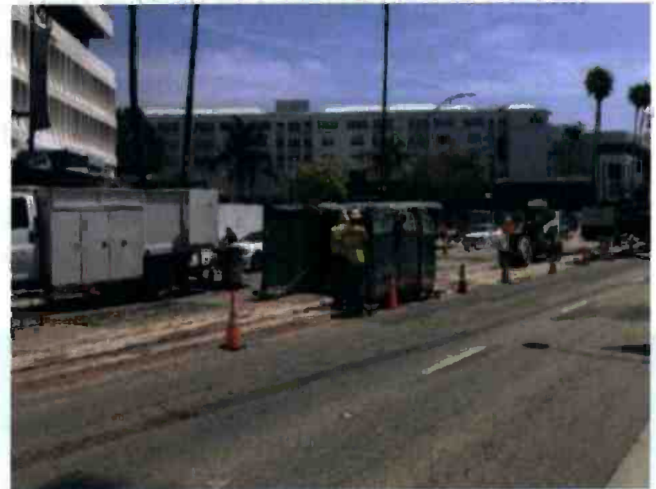
Utility Potholing Activities
