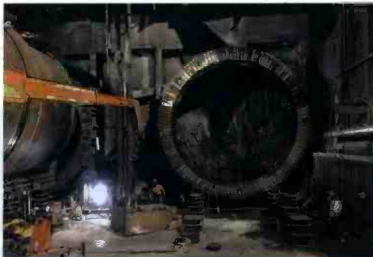
TBM Cradle at Reach 2 Tunnel
