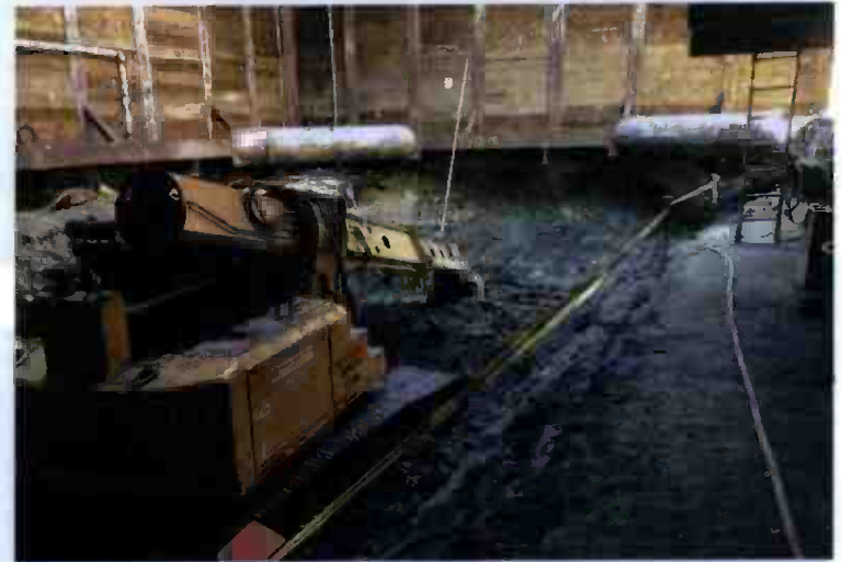
Level D Excavation / Removal of Crane Mats
