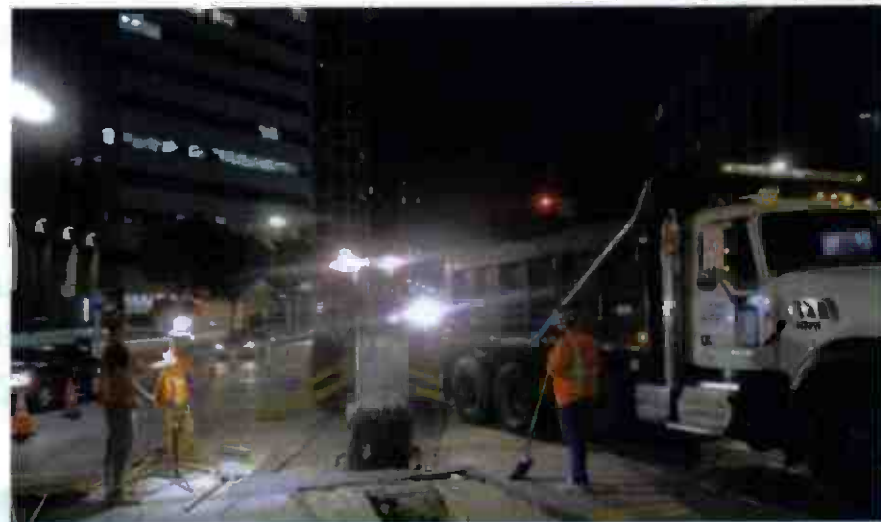
Westwood Blvd. at Wilshire Blvd. Main Line A Excavation and Potholing
