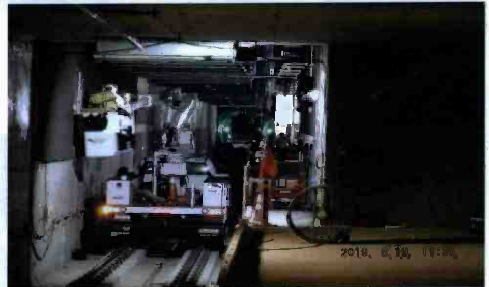
UG4 – Systems installation work looking north toward Leimert Park Station
