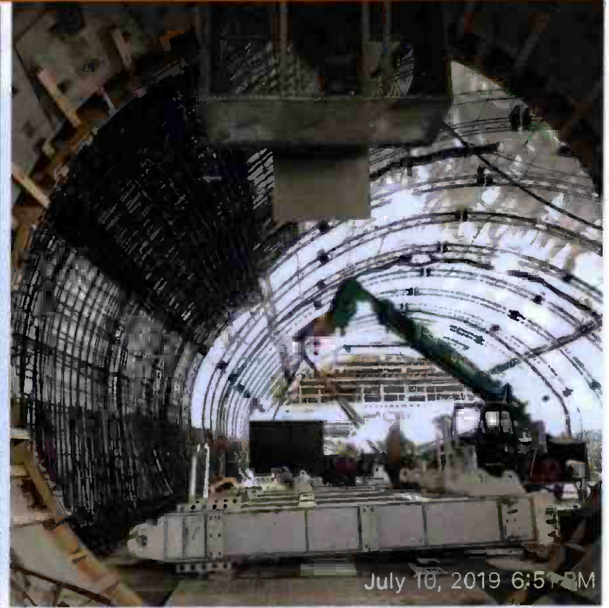
Wall form installation at right track
