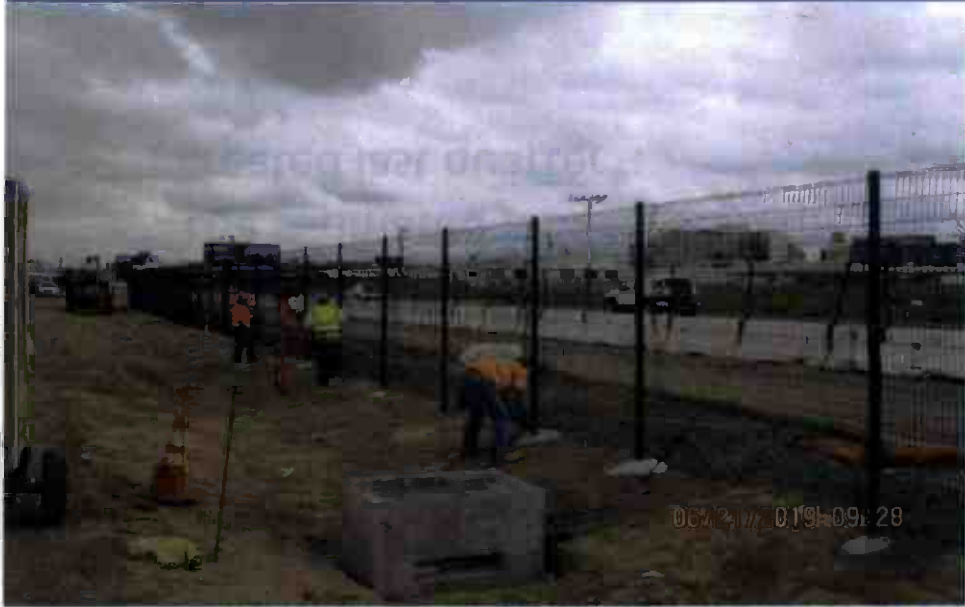
Guideway Between UG1 and 104 th St. – Installing wire fence
