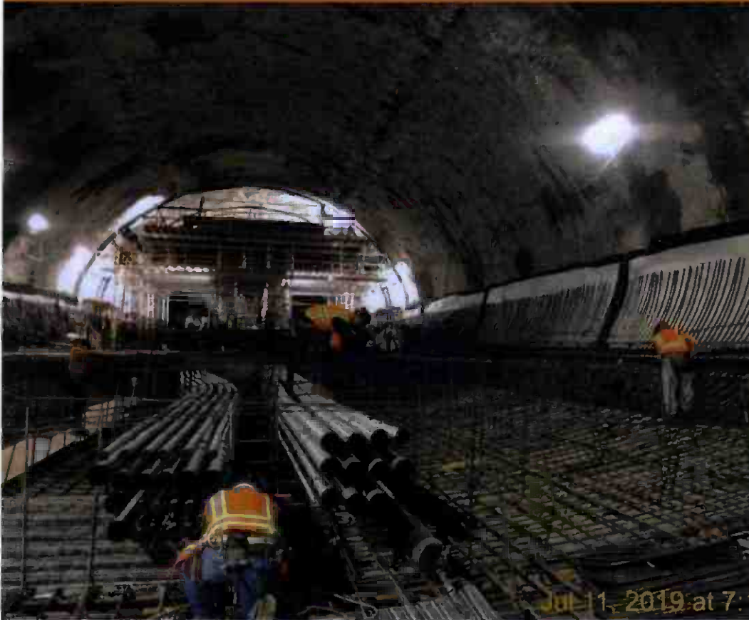
Top mat rebar installation at SEM Cavern invert
