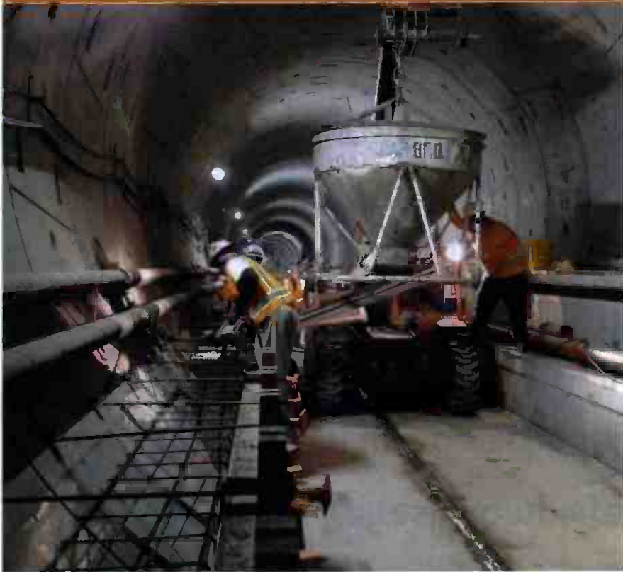
Concrete pour in progress for Floating Slab Track curb
