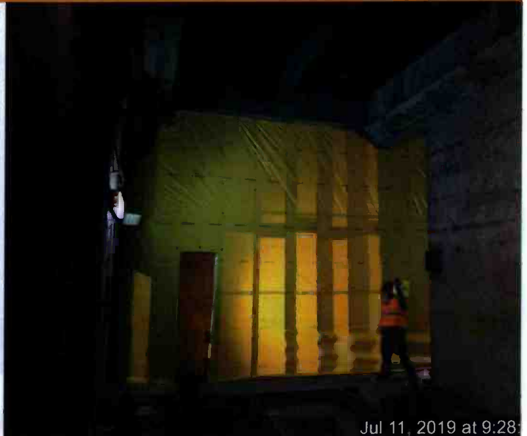
Dust barrier installed at 7th/Metro bulkhead
