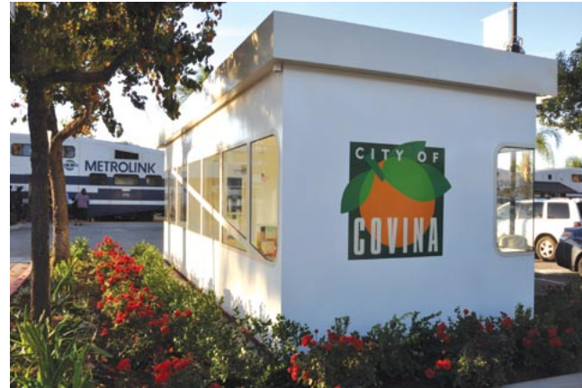
This new modular Bikestation is located in the parking lot of the City of Covina Metrolink Station at 600 N. Citrus Avenue.
