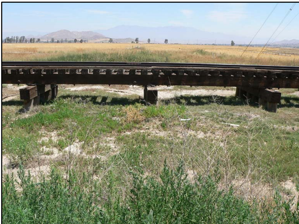
SAN JACINTO RIVER OVERFLOW CHANNEL BRIDGE MP 20.80
