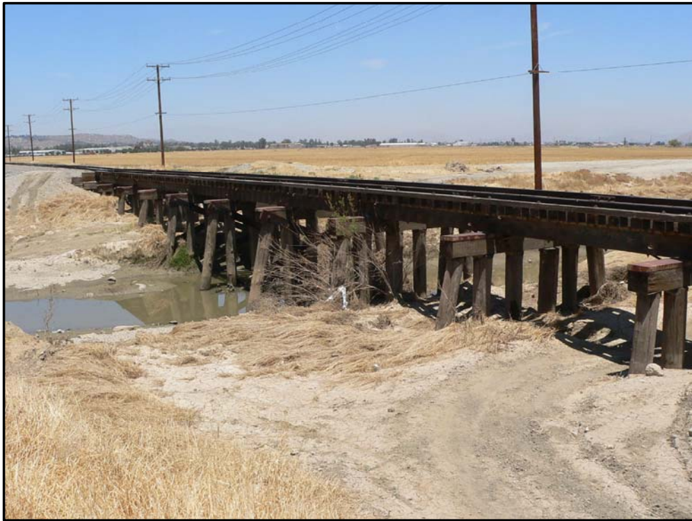
SAN JACINTO RIVER BRIDGE MP 20.70
