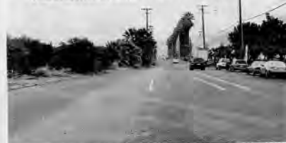
These trees will be gone when Palmyrita is widened to match the existing width of the street. Notice how the trees extend into the right-of-way where the road narrows? Palmyrita is wider at both ends of this small orange grove.
