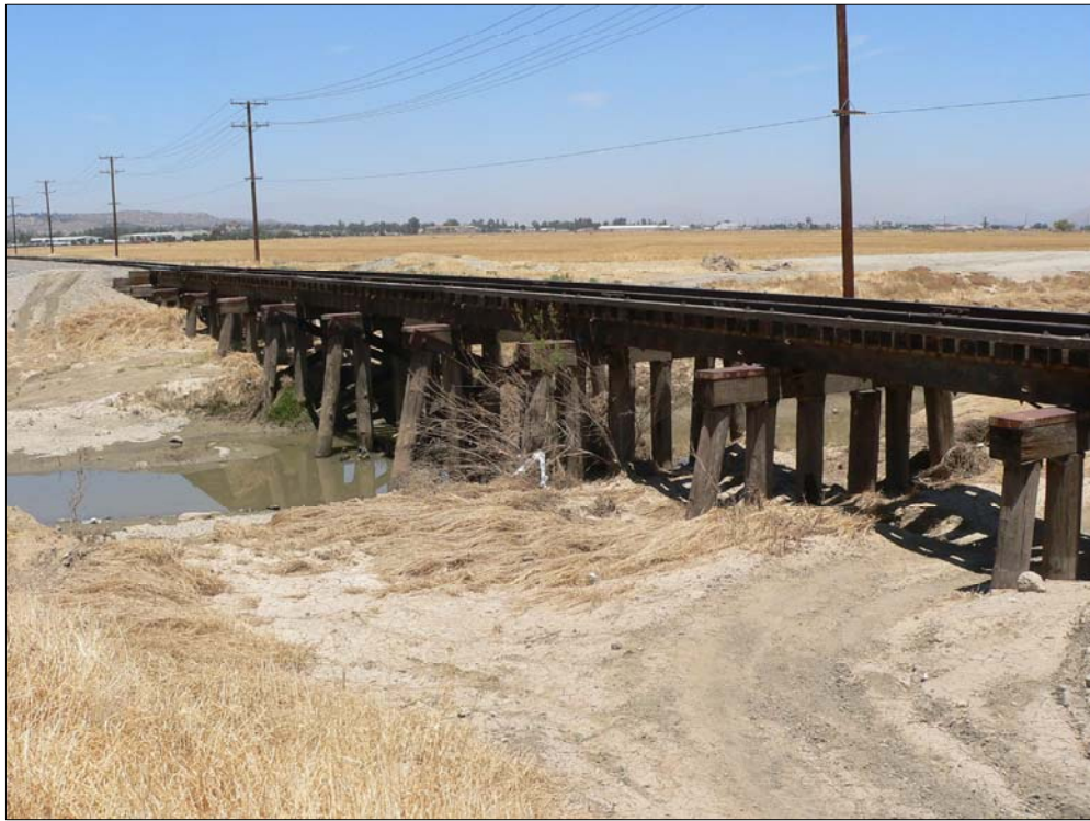
SAN JACINTO RIVER BRIDGE MP 20.70
