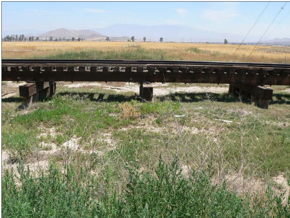
SAN JACINTO RIVER OVERFLOW CHANNEL BRIDGE MP 20.80
