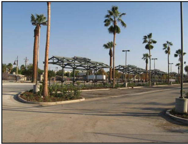
SITE PHOTOGRAPH (VIEW NORTH)
