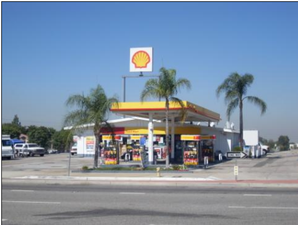
Photo 7: Shell Service Station with closed leaking underground storage tank (LUST) case onsite (Map Code U). View is toward the west.
