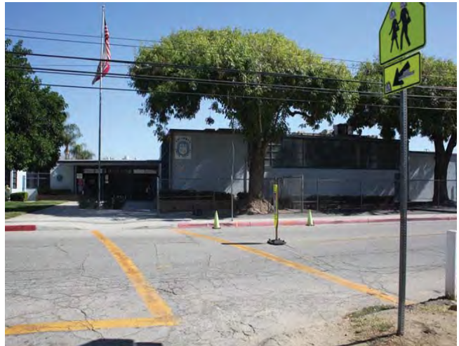
West elevation, looking east
