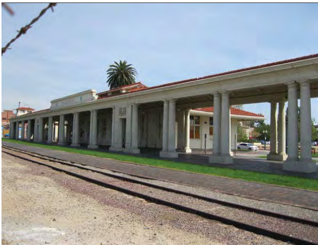
North elevation looking southeast
