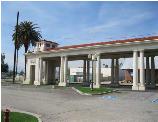
South elevation looking northwest
