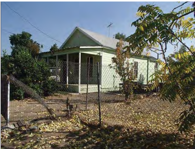
North and west elevations, looking southeast
