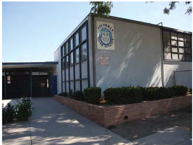
North and west elevations, looking southeast
