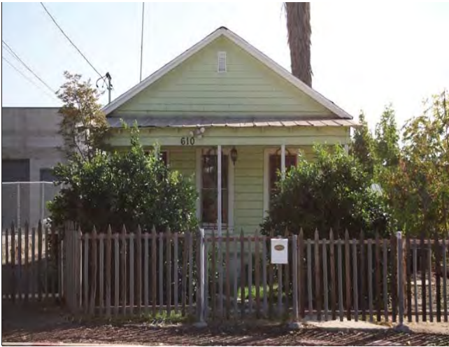
North elevation, looking south
