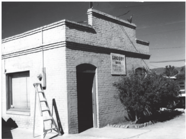
1991 photo. East and south elevations lkg northwest
