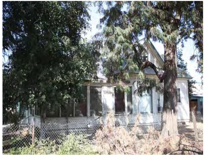
South elevation, looking north
