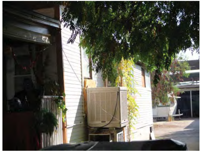
West elevation, looking southeast
