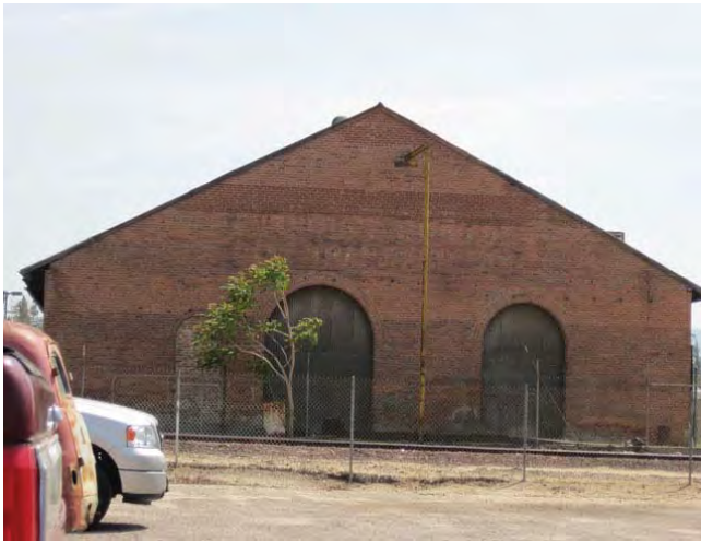
North elevation, looking south
