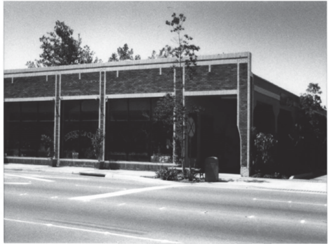
1991 photo. East and north elevations lkg southwest
