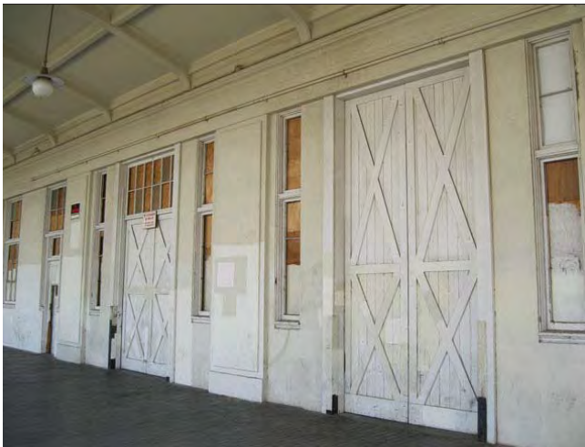
North elevation looking southeast
