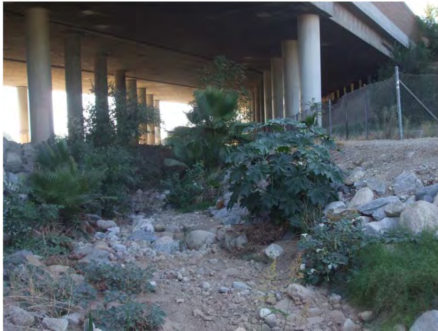
Photograph 4: Zanja underneath 1-10, view to west
