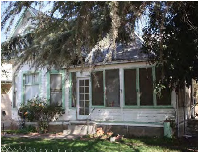
West elevation, looking east
