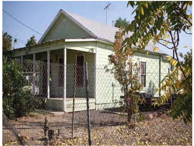
North and west elevations, looking southeast
