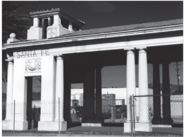
1991 photo. South elevation looking north
