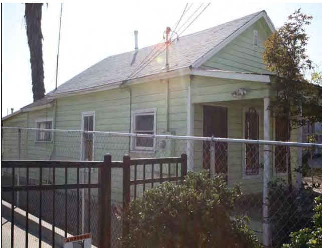
North and east elevations, looking southwest
