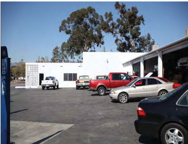
Looking north, rear elevation and attached building
