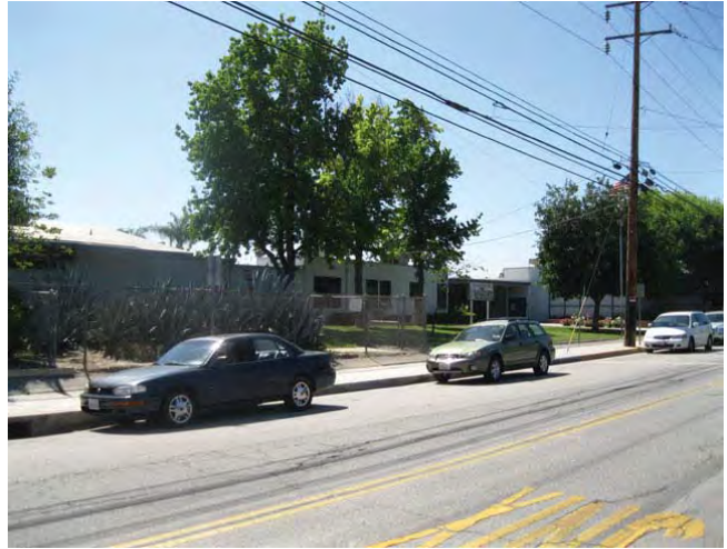
Street view, west elevation, looking southeast
