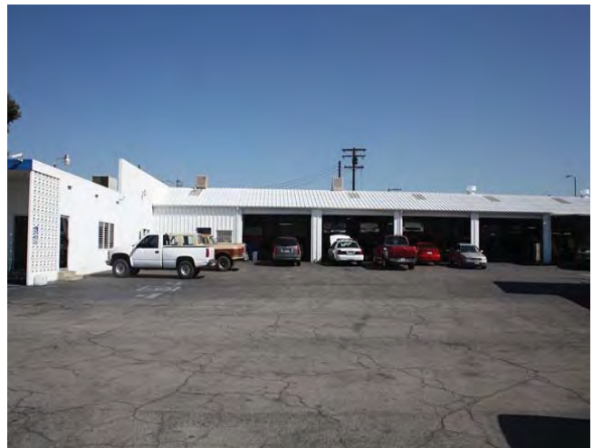
Looking east, rear elevation and attached building
