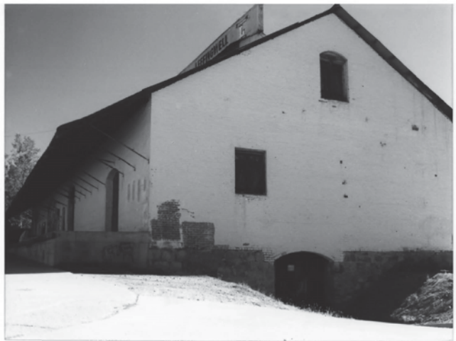
1991 photo. West and north elevations lkg southeast
