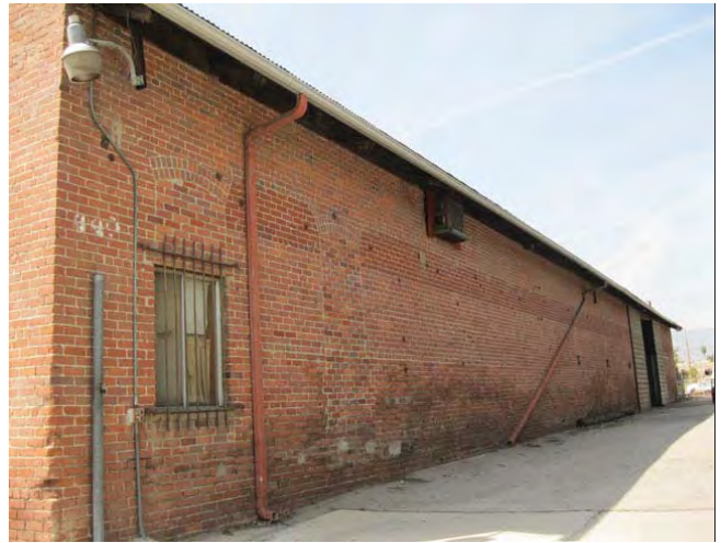
East elevation, looking northwest
