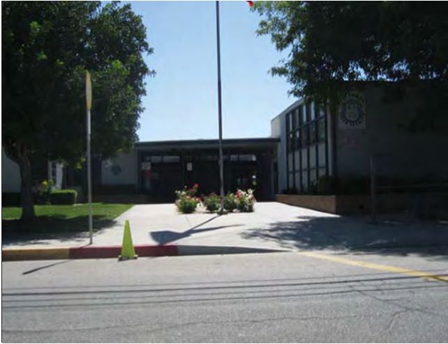
West elevation, looking east
