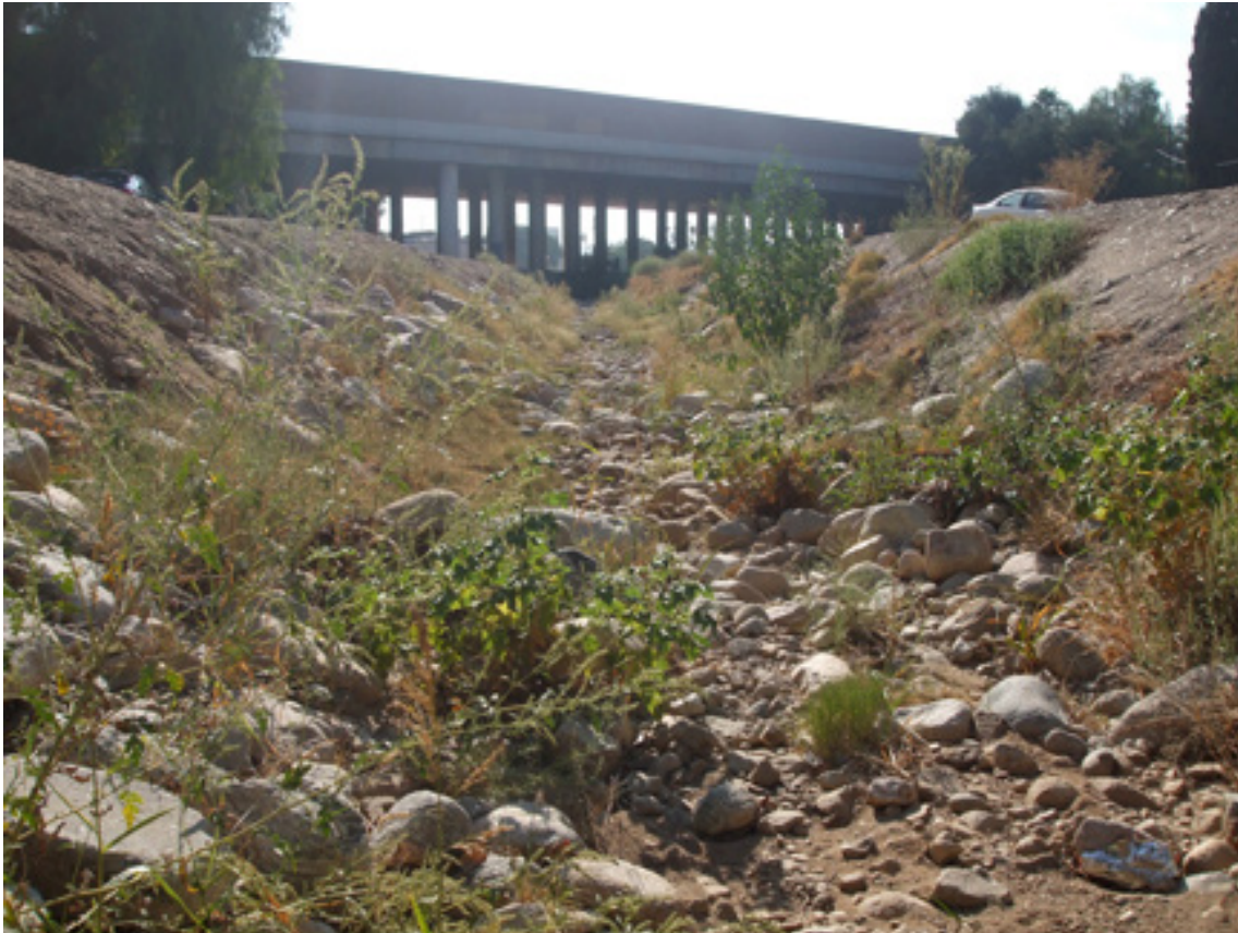
Figure 3-3. Mill Creek Zanja West of Division Street, View West.
