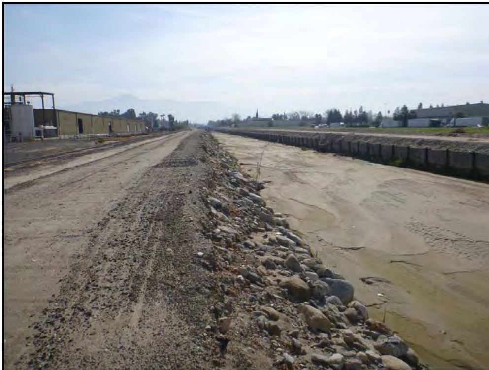
Photograph 4. View of the artificially levied Zanja channel. Throughout the channel rodent burrows form along the earthen berm, in the large rock and concrete riprap.
