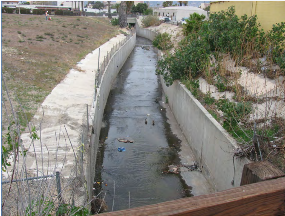
Photograph 5. Northerly view of Warm Creek a non-vegetated channel.
