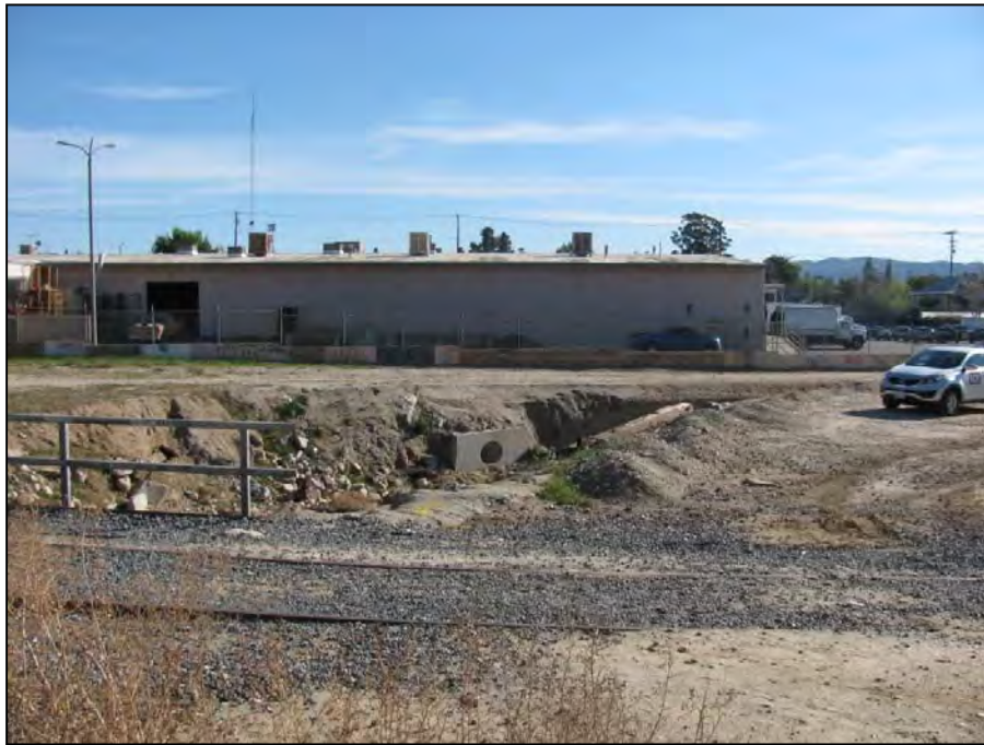
Photograph 13. Mill Creek Zanja. Westerly view.
