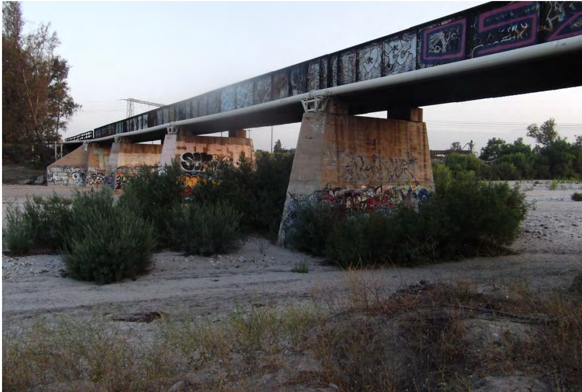
Photo 1. Standing on west side of bridge looking north/northeast.
