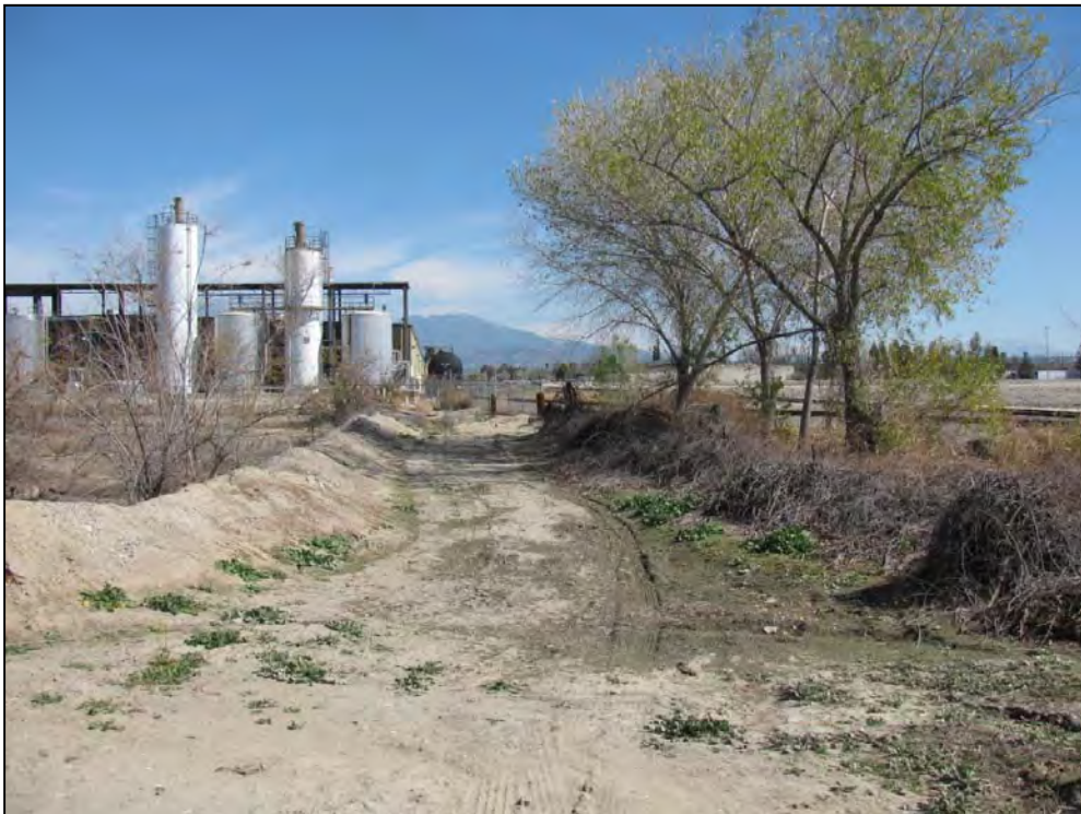
Photograph 18. Manufactured earthen berm separating the storm water runoff (soil pits #1 and #2) from Zanja Channel .
