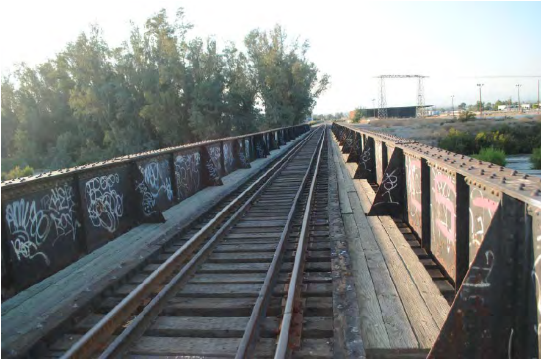
Figure 2: Existing AT&SF Bridge 3.4
