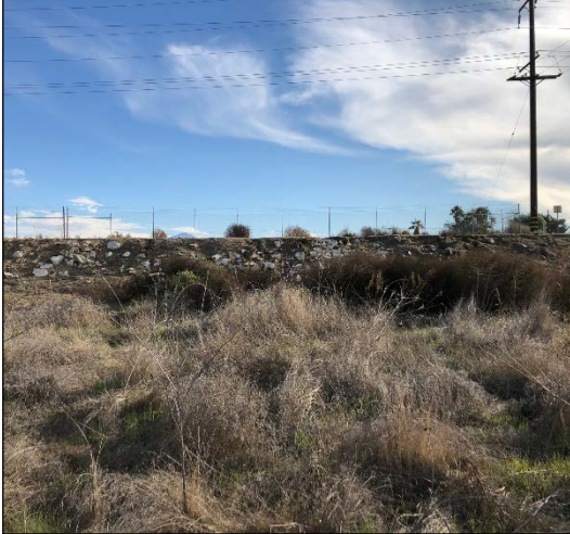
Photograph 1. View east towards railroad tracks and proposed connection outfall structure.
