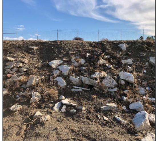
Photograph 2. View of bank where proposed connection outfall structure would be located.
