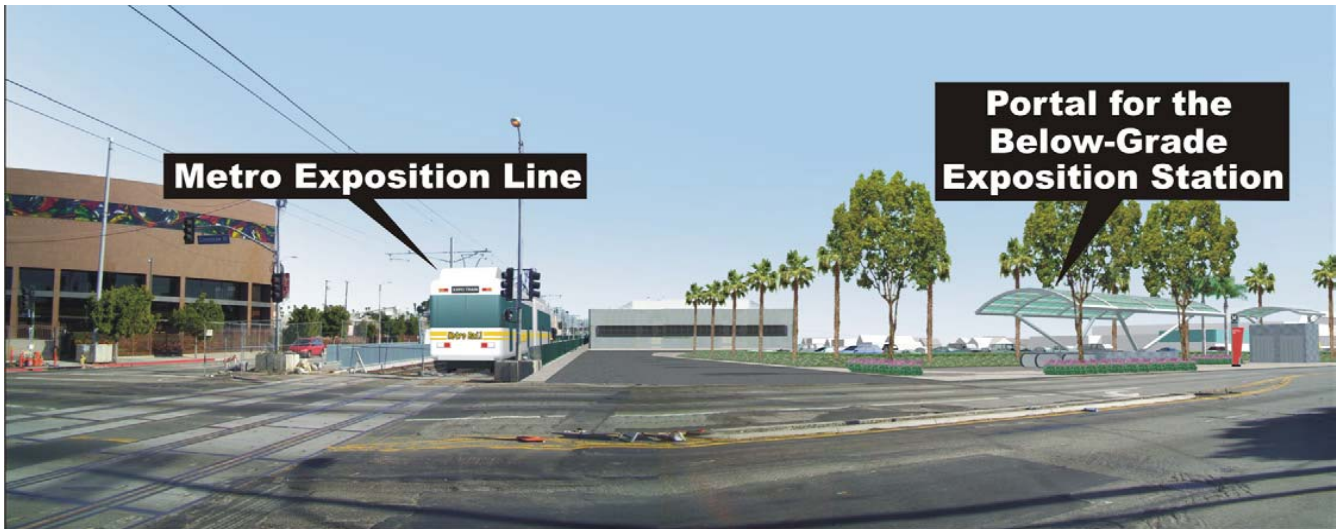
Rendering of portal for the below-grade Crenshaw/Exposition Station that is adjacent to the operation of the at-grade Exposition Line.
