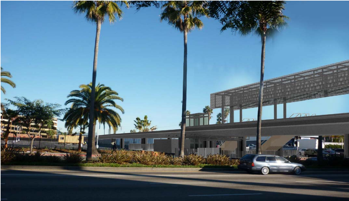
Typical Aerial Station.
