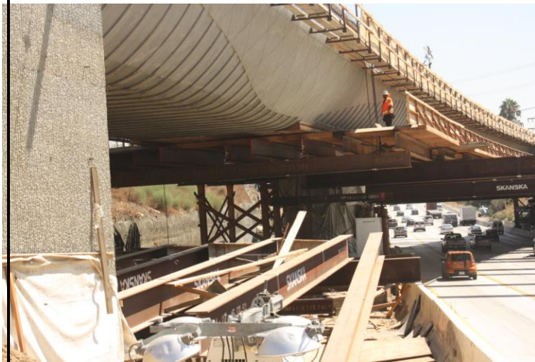
Falsework removal in process
