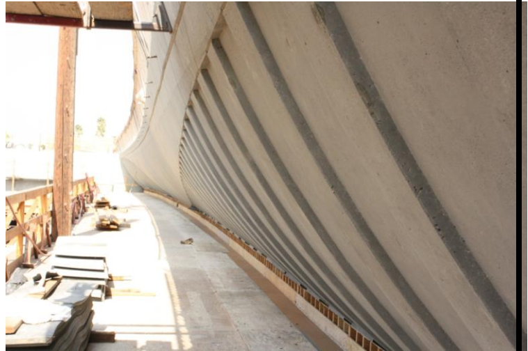
View of removed exterior formwork
