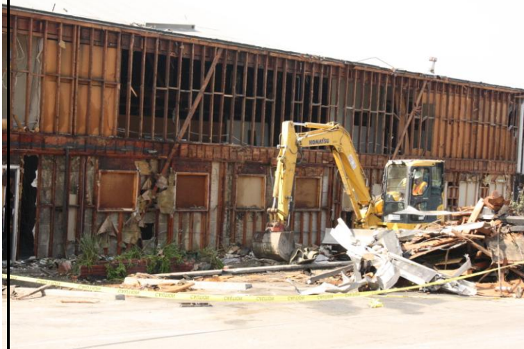
Abatement work at M&O Facility existing buildings
