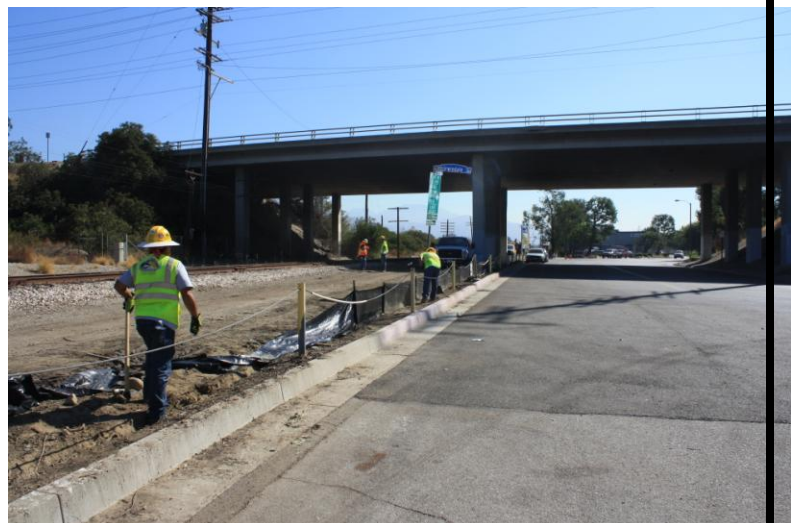
Clearing and grubbing work in Irwindale
