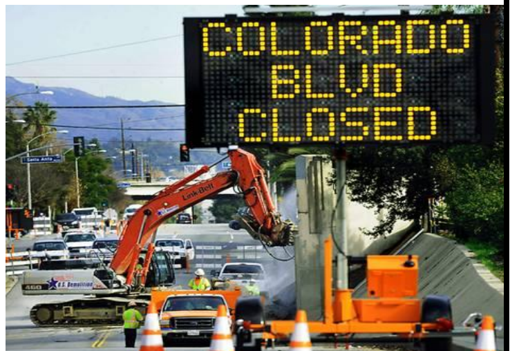
Example of Notices for Colorado Bridge Work
