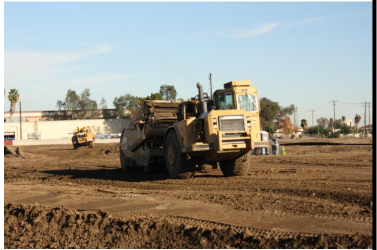
Grading work at Gold Line Operations Campus
