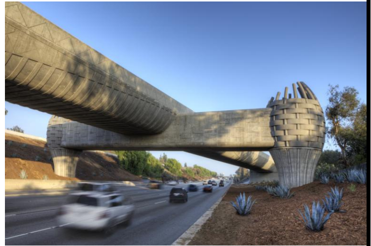
View of finalized bridge
