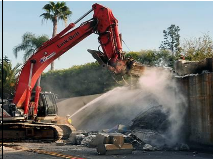
Work at Colorado Bridge
