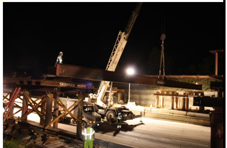
Nighttime freeway closure for Falsework erection
