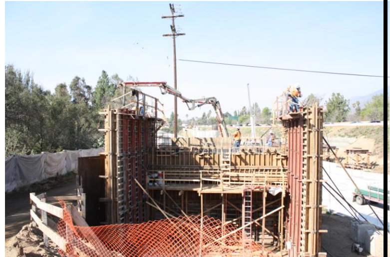
Concrete pour at South Abutment
