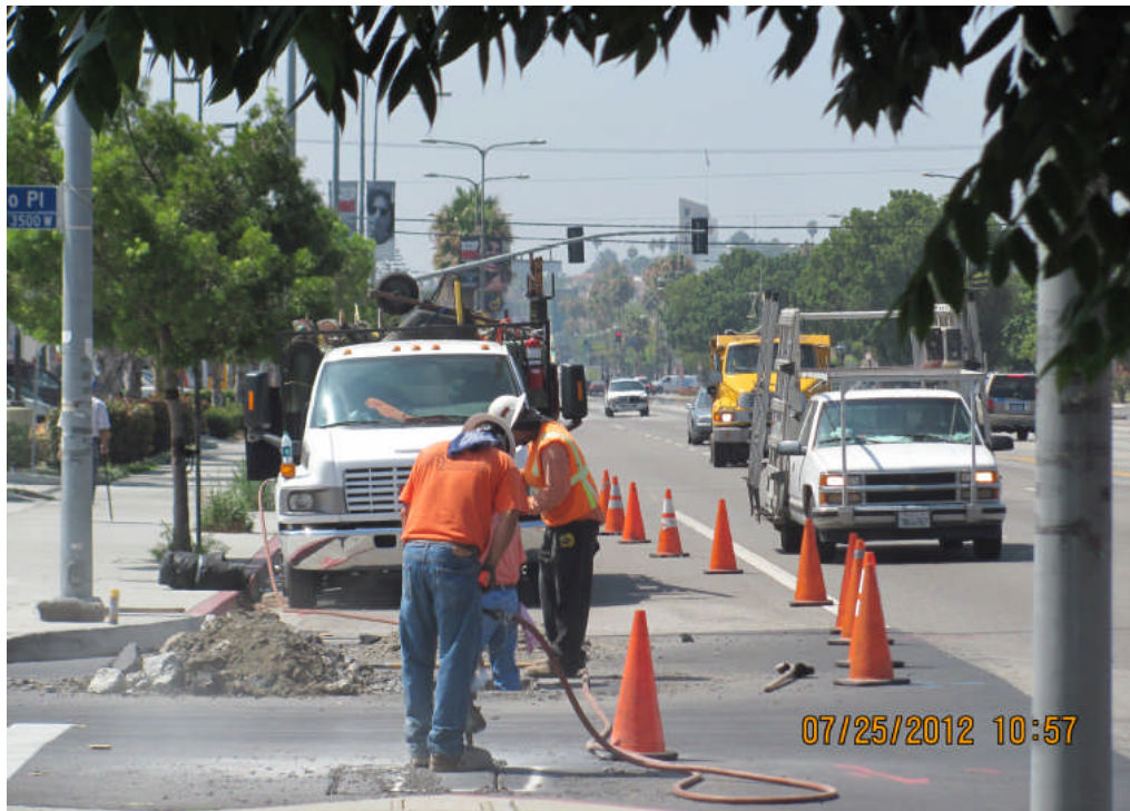
The Gas Co. locating utilities at Rodeo Pl. and Crenshaw Blvd.
