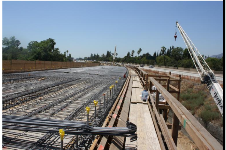
Deck Formwork
