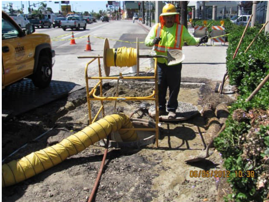
Duct construction at manhole, Crenshaw and MLK.
