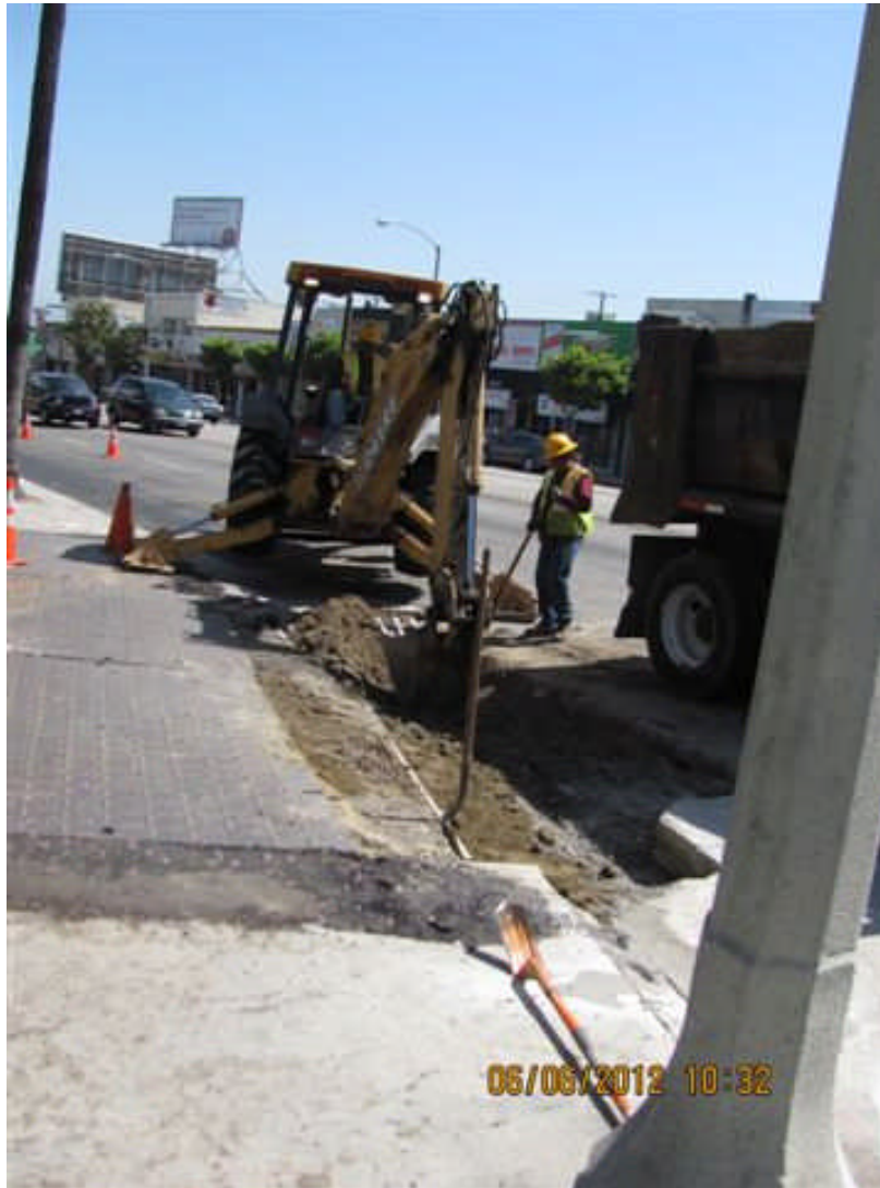
Preparing to place inner-duct at Manchester Blvd.
