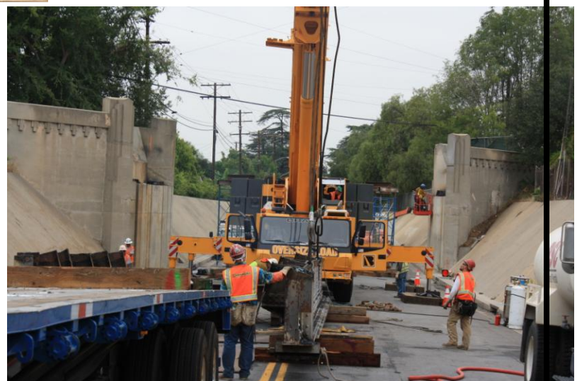
Post-demolition view of Colorado Bridge
