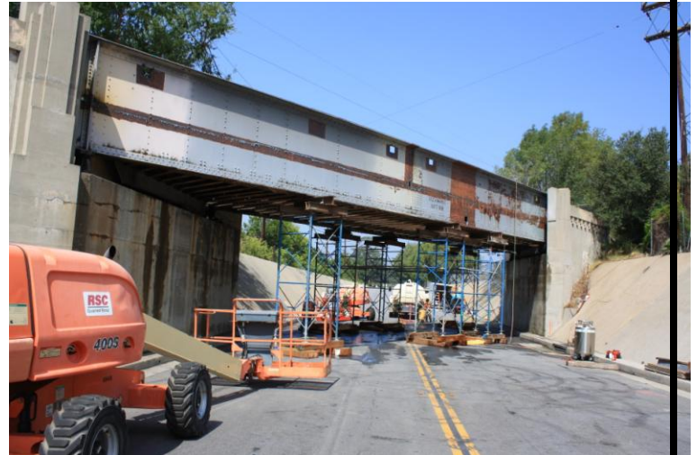
Prepping for Colorado Bridge demolition
