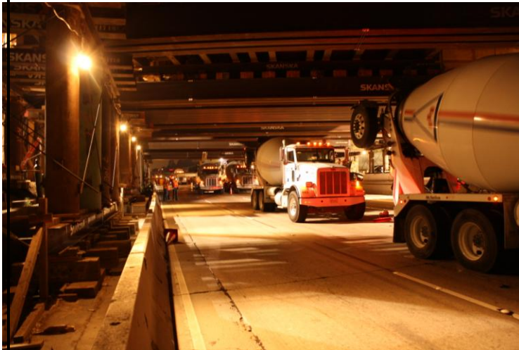
Approximately 215 Concrete Trucks Brought in for the Concrete Pour
