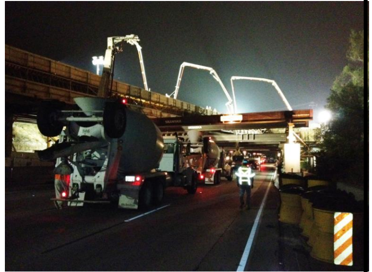
Nighttime Freeway Closure and Concrete Pour
