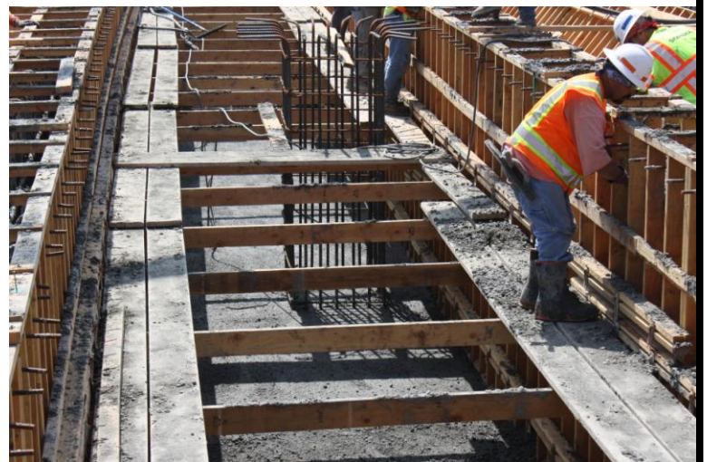
View of Bridge after Concrete Placement
