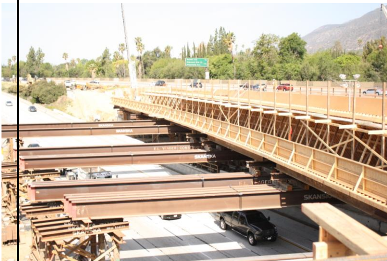
Installation of formwork
