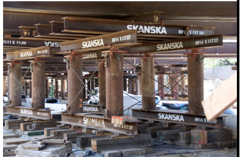
View of fully installed temporary falsework
