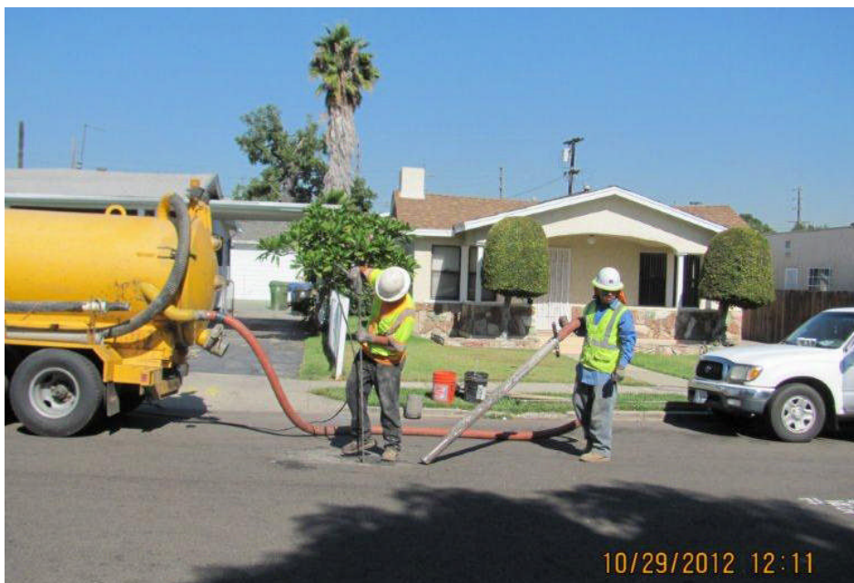
Crews locating utilities near 59 th Street.
